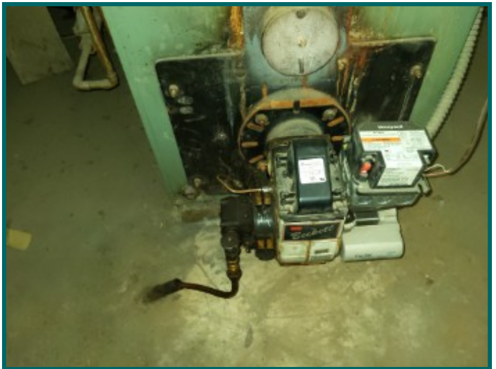
Oil shut off valve at boiler.
