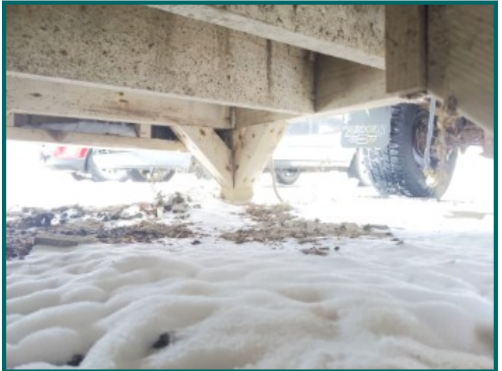
Missing joist hangers and footings were not located at left side porch/landing.
