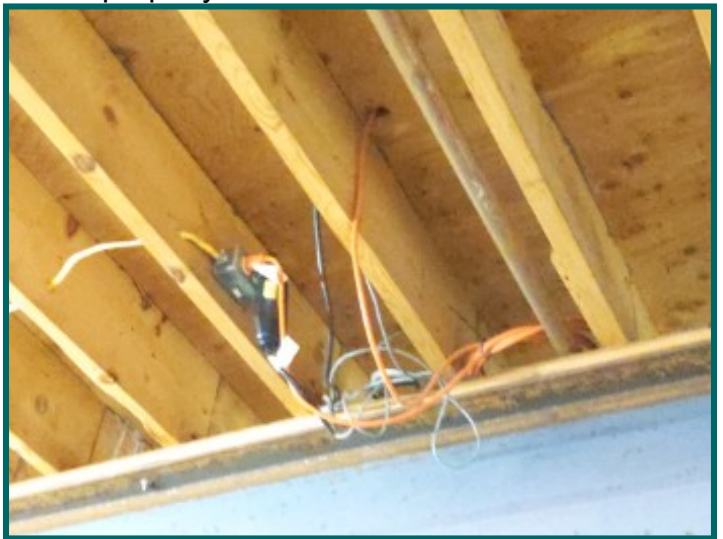
Improper use of extension cord in basement.
