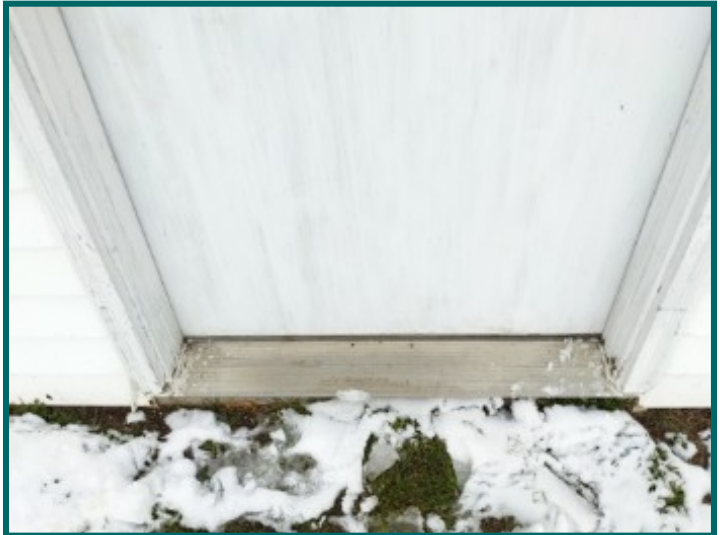
Damage at lower door and frame and peeling paint at right side lower level door.
