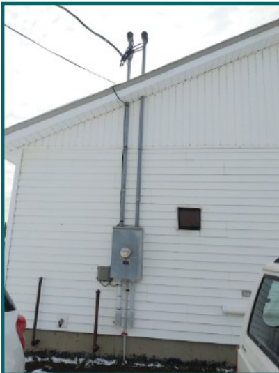
Electric meter and main service entrance at left side of building
