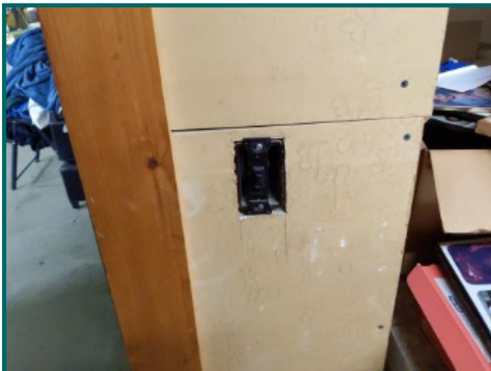
Several missing outlet covers / switch covers throughout.
