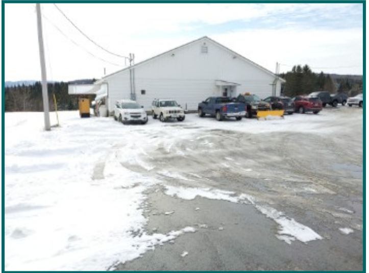
Grading at left side of building is toward the foundation
