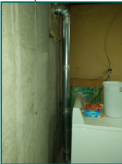
Rigid dryer vent hose is an approved material.
