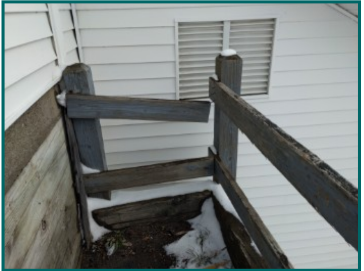
Damaged guardrail
