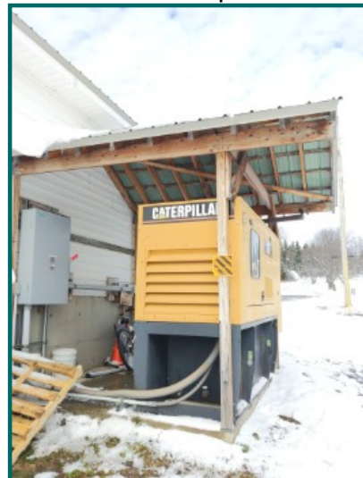
Support post at rear overhang is not plumb.
