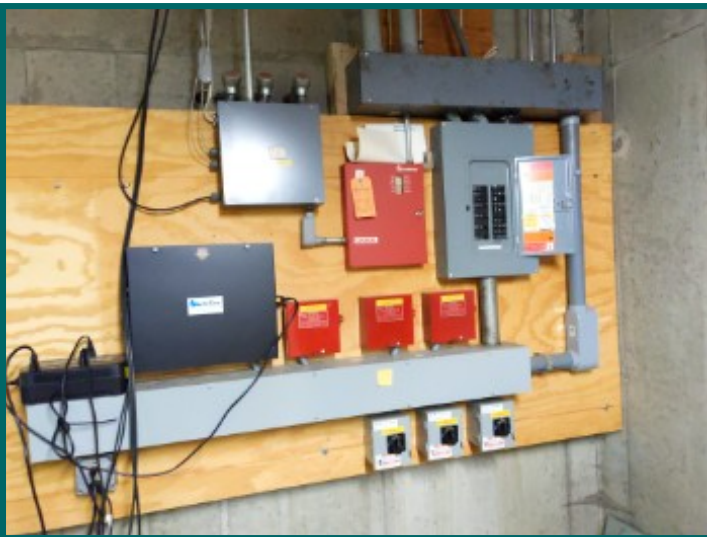
Electrical panel/equipment for gas pumps
