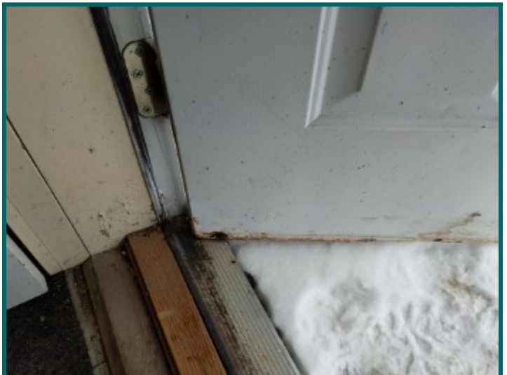
Corrosion / damage at left side door
