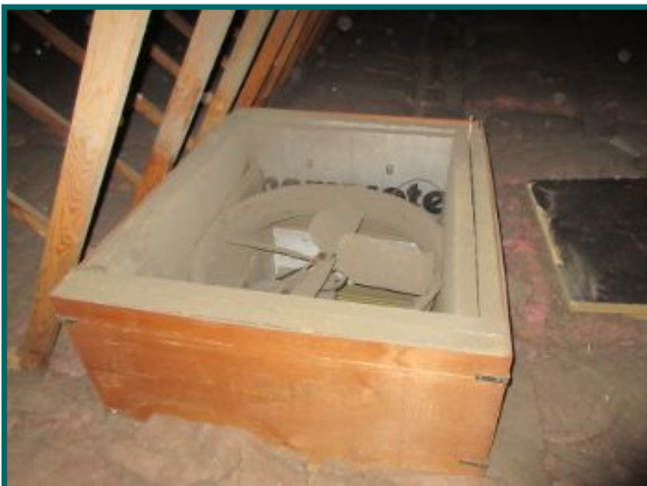
recommend insulating vent fan in winter
