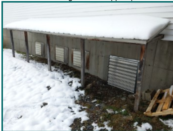
Settlement at rear overhang / missing footings
