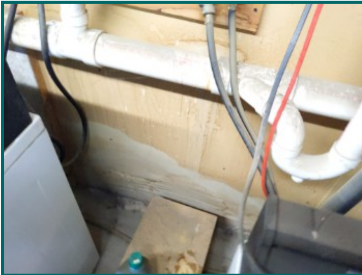
Water staining and damage to wall behind basement laundry. Area tested dry.
