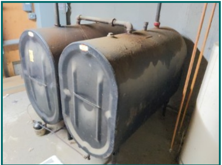
Staining on oil tanks in basement
