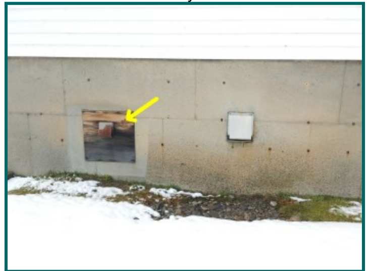
Dryer vent termination
