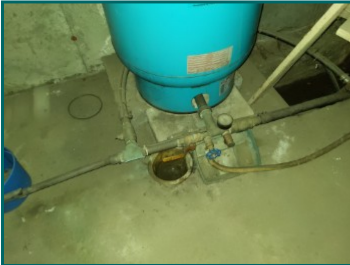
Main water shut off valve is located at well tank. Valve is leaking.
