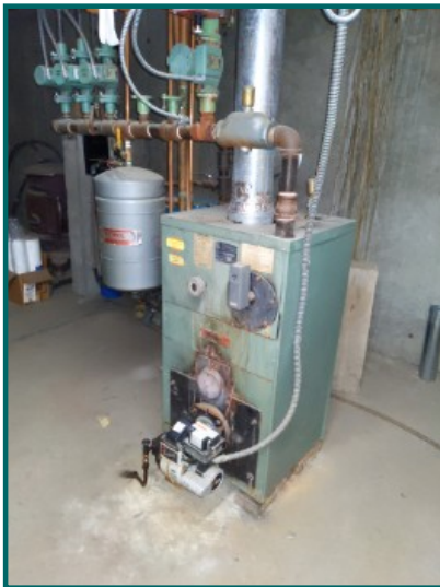
Oil fired boiler in basement, 32 years old. Corrosion on boiler / boiler plumbing.
