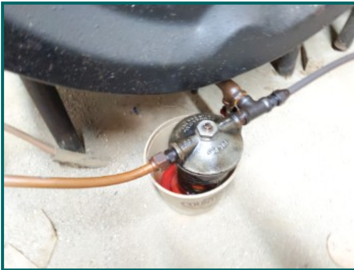
Oil leak at shut off valve/filter
