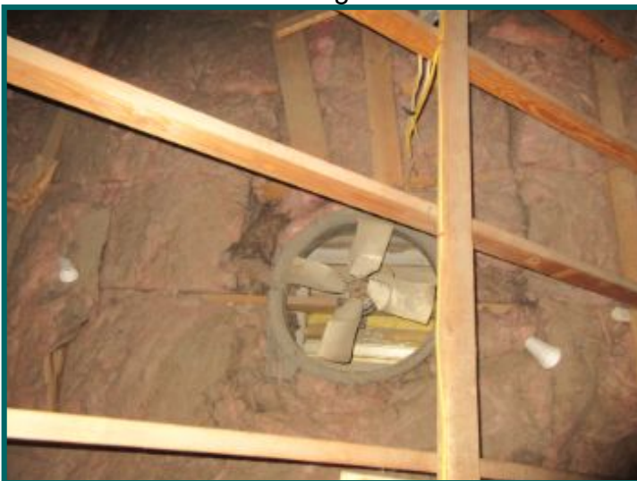
deli area fan improperly terminates in attic
