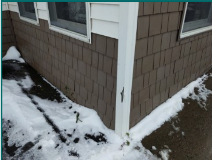
Damaged siding is in contact with ground at front / left side
