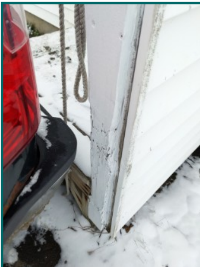
Damaged framing/post at left side landing
