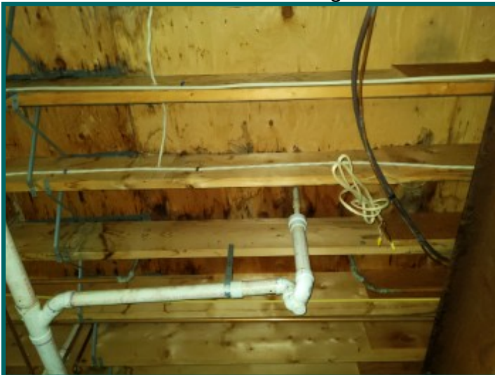
Water staining at rear / left side of basement
