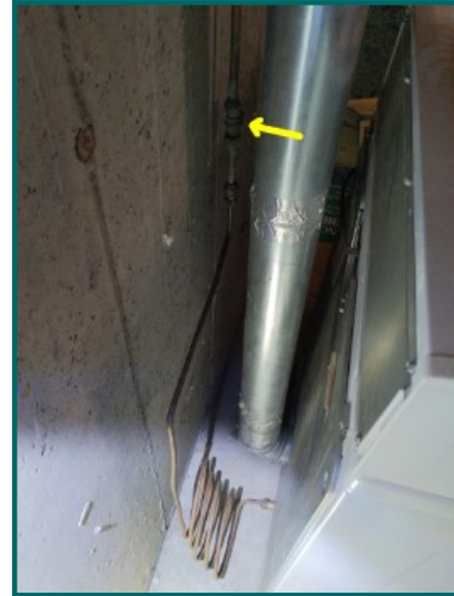
Fuel for dryer is propane gas. Gas shut off valve at dryer.
