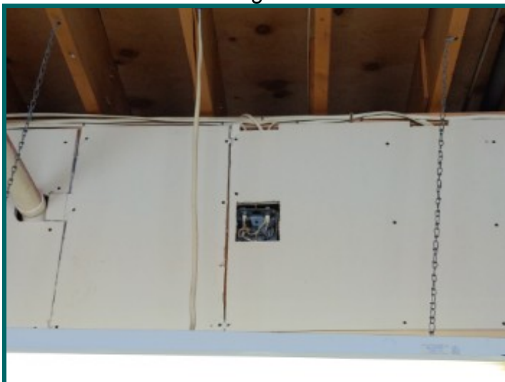
Open junction boxes in basement
