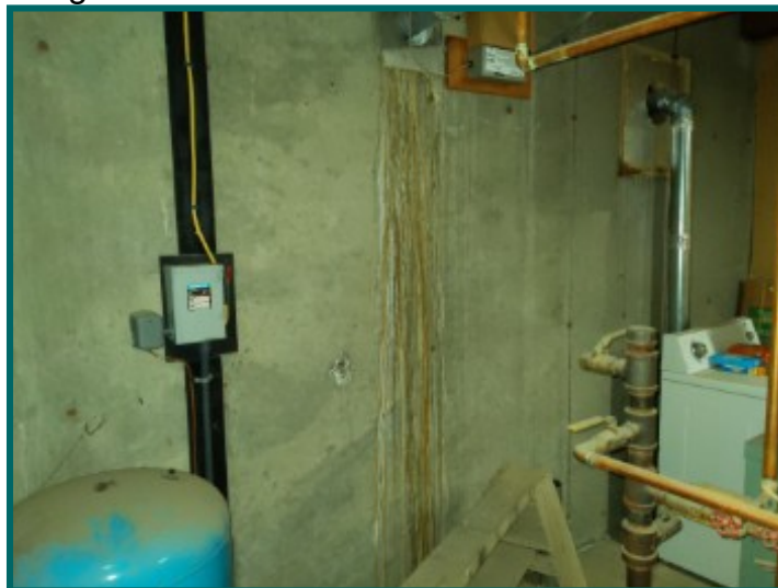
Water staining around boiler vent
