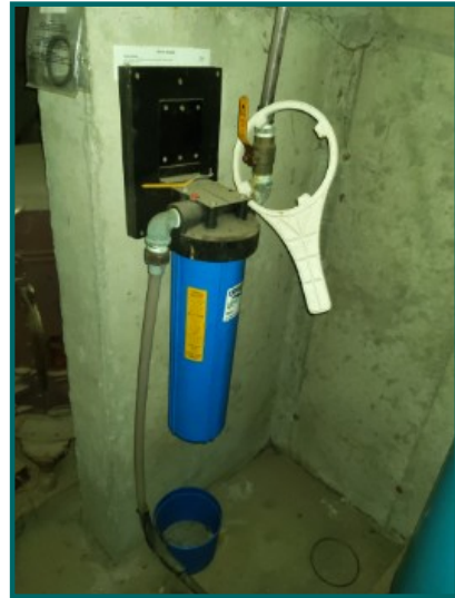
Sediment Filter, recommend changing to clear cover to observe when filter needs changing.
