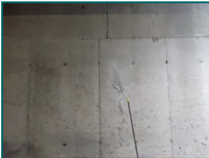
Vertical crack and water staining / efflorescence at left side wall
