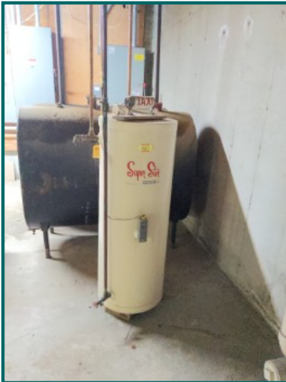
Single water heater integrated with boiler, exact age not determined but appears to be approaching design life.
