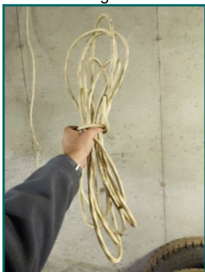
Improperly terminated wires at front basement wall.
