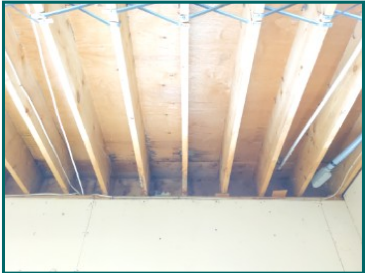
Water staining at right side of basement
