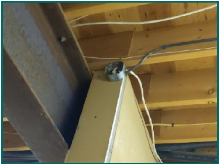
Open junction boxes in basement
