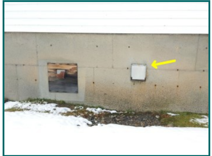
Boiler vent termination
