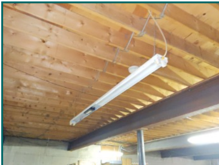
Several damaged fixtures / lights out in basement.
