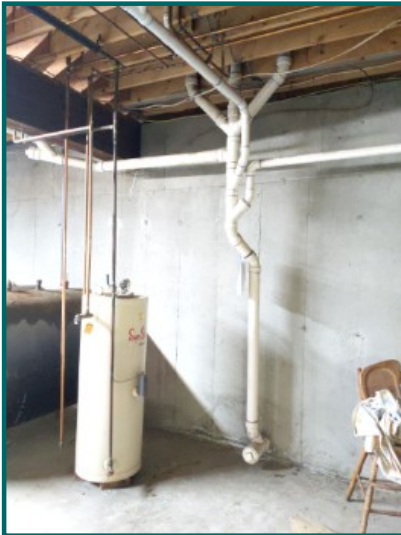
Main drain line termination in basement
