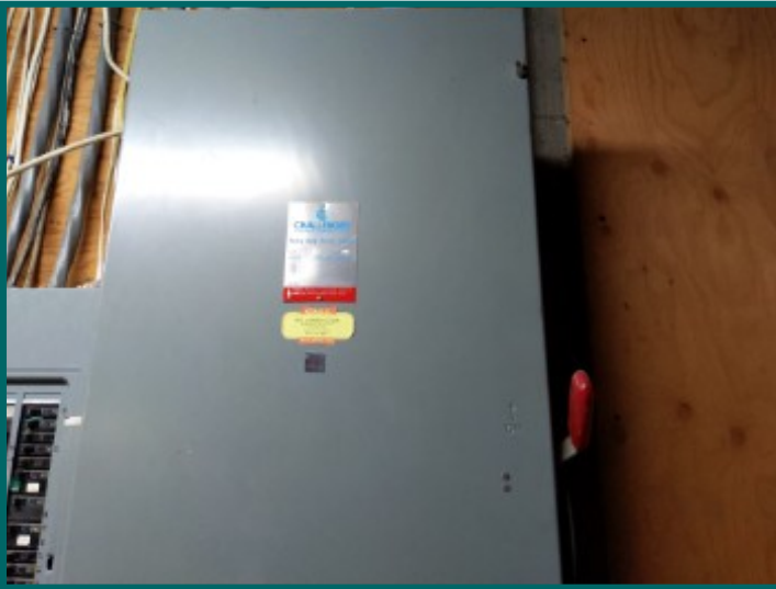
400 amp, 120/240 volt, single phase service disconnect in basement.
