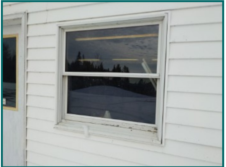
Peeling paint at right side windows.
