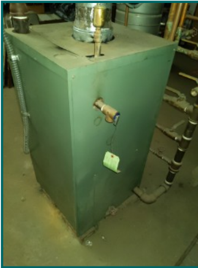
Missing down pipe on boiler TP valve
