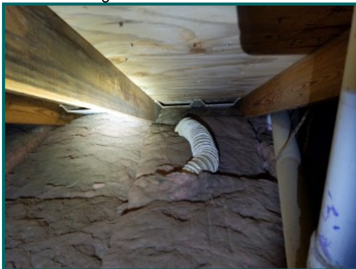
Improper bathroom vent fan termination
