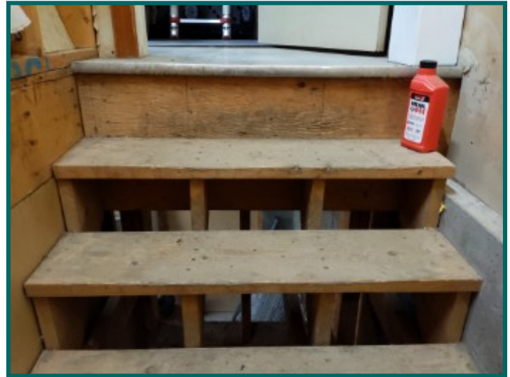
Uneven riser heights / stairs are not built to today's safety standards.
