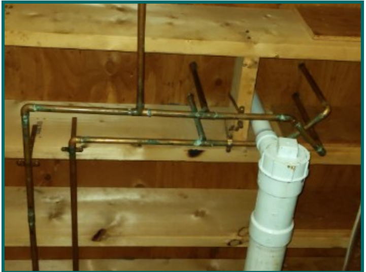
Corrosion on plumbing through basement
