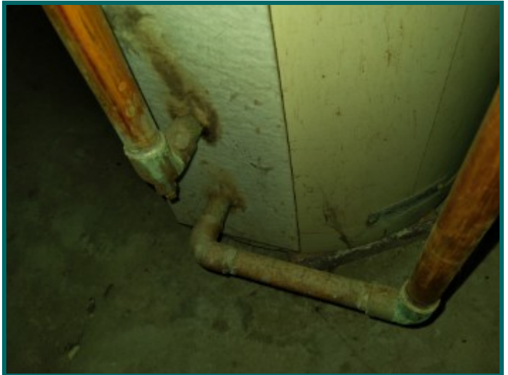
Corrosion at water heater plumbing lines / fittings.
