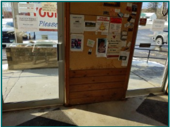
Front door does not seal well
