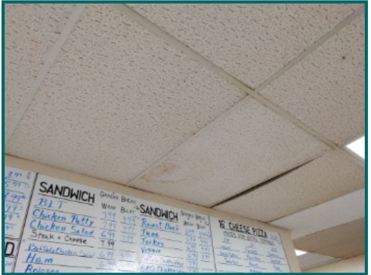
Water staining on ceiling above deli
