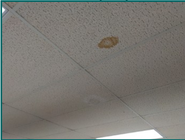
Water staining on ceiling throughout retail space.
