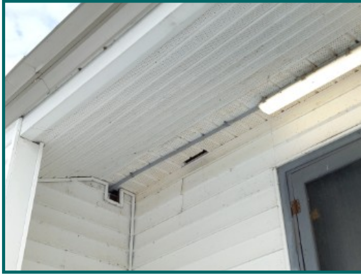
Gap in soffit at front of building
