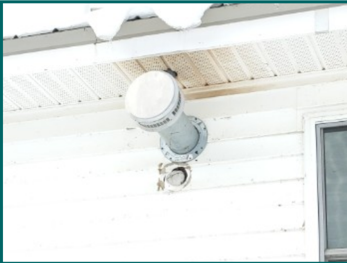
Open penetration at rear of building
