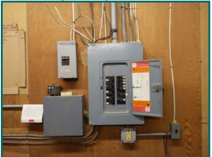
Refrigeration equipment electrical panel
