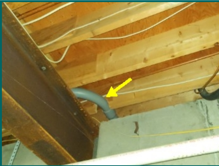
Improperly notched joist at rear / left side of basement
