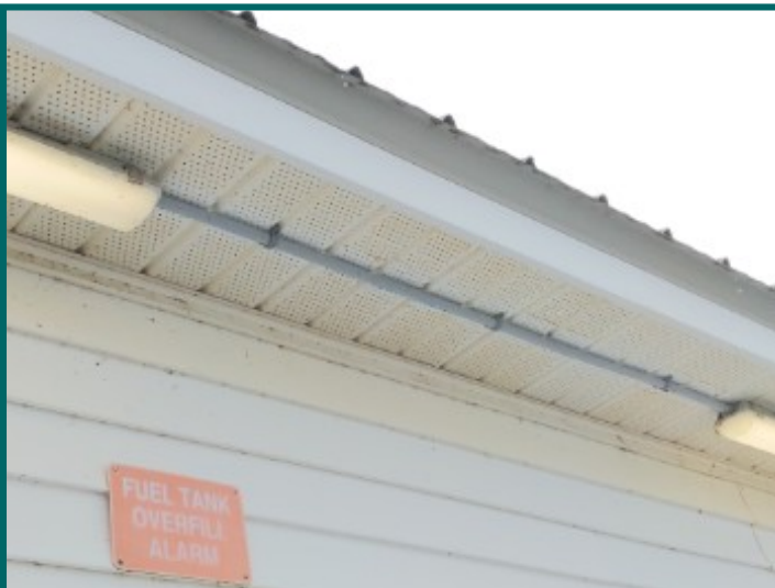
Soffit Vents
