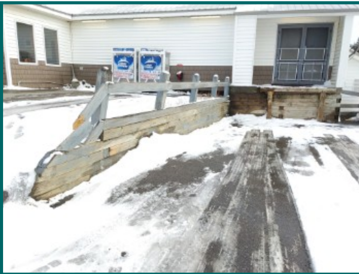
Front retaining wall is damaged / leaning
