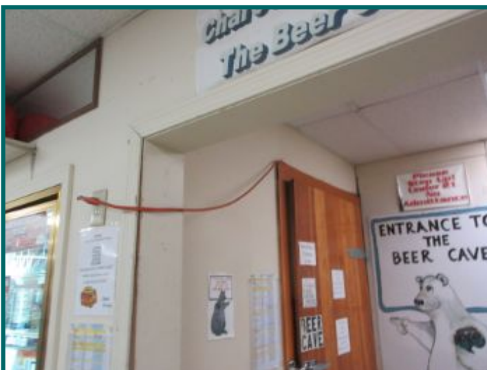
improper use of extension cord
