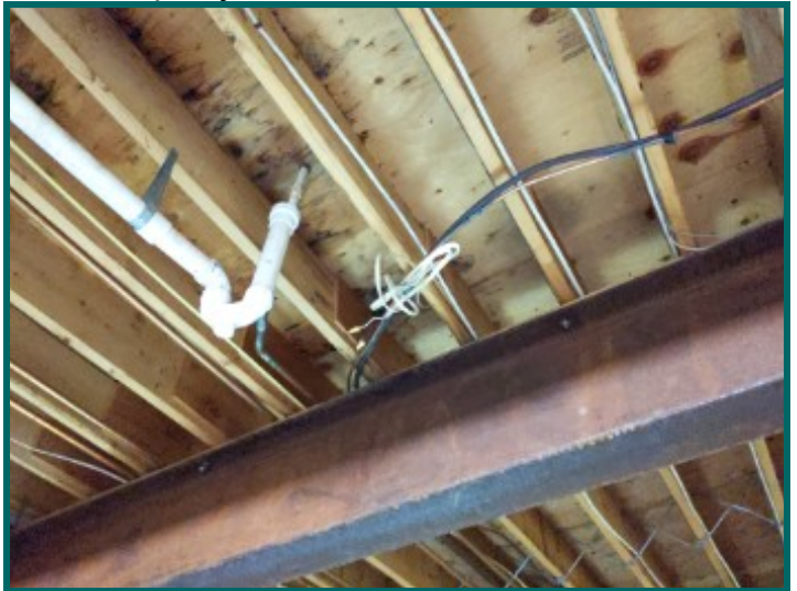
Improperly terminated wires in basement.
