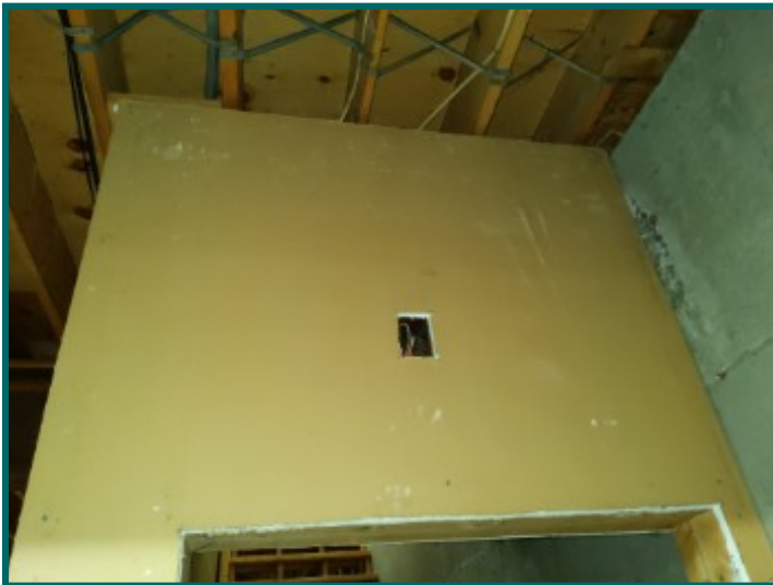
Open junction boxes in basement
