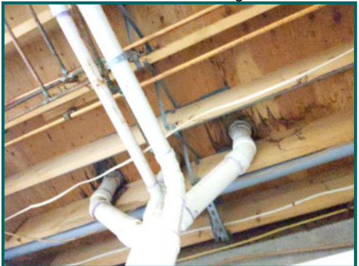
Water staining below bathrooms
