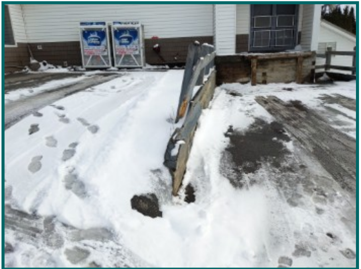
Front retaining wall at loading dock is leaning
