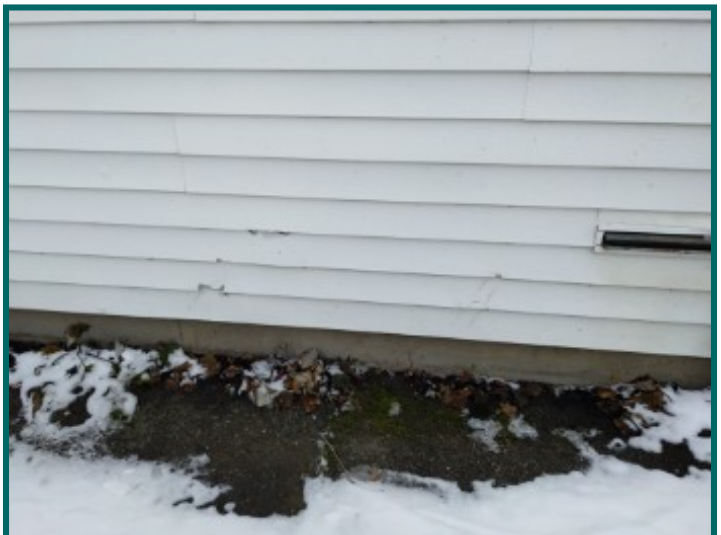
Damaged siding at left side of building
