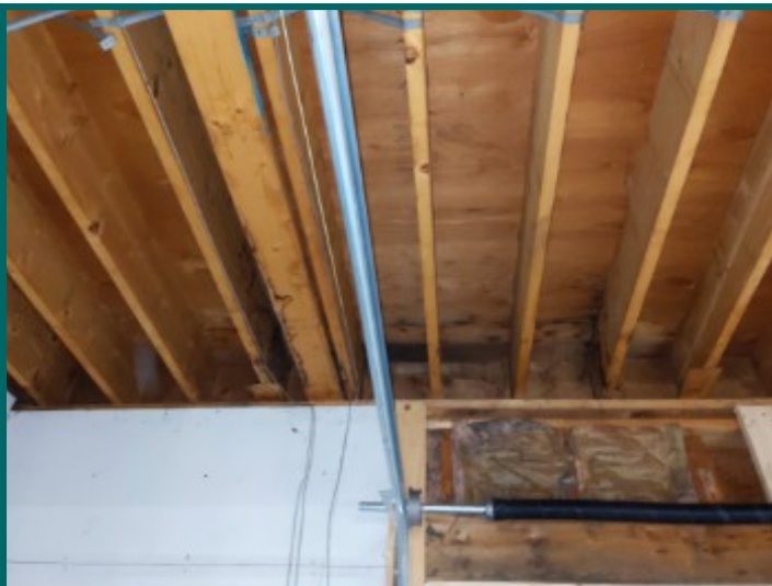
Water staining at right side of basement
