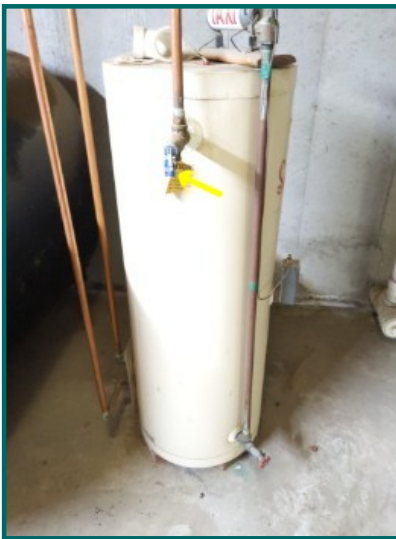
Missing downpipe at TPR valve.
