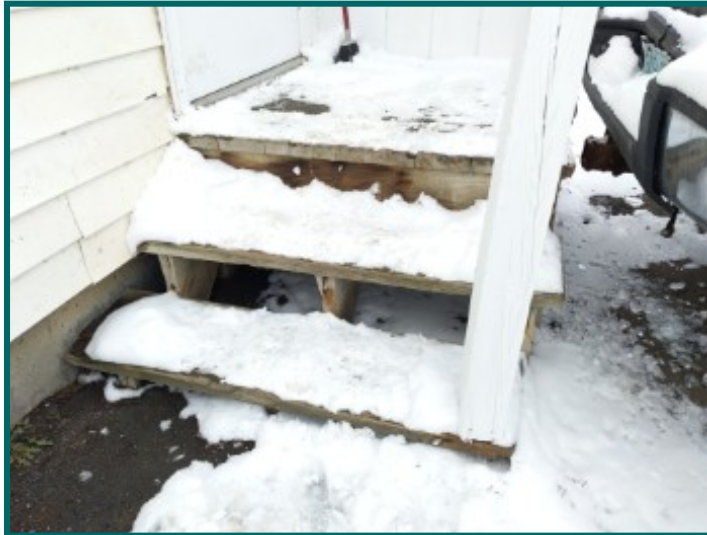
Uneven riser height and damaged framing at left side stairs
