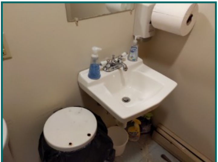
Loose sink in employee bathroom.
