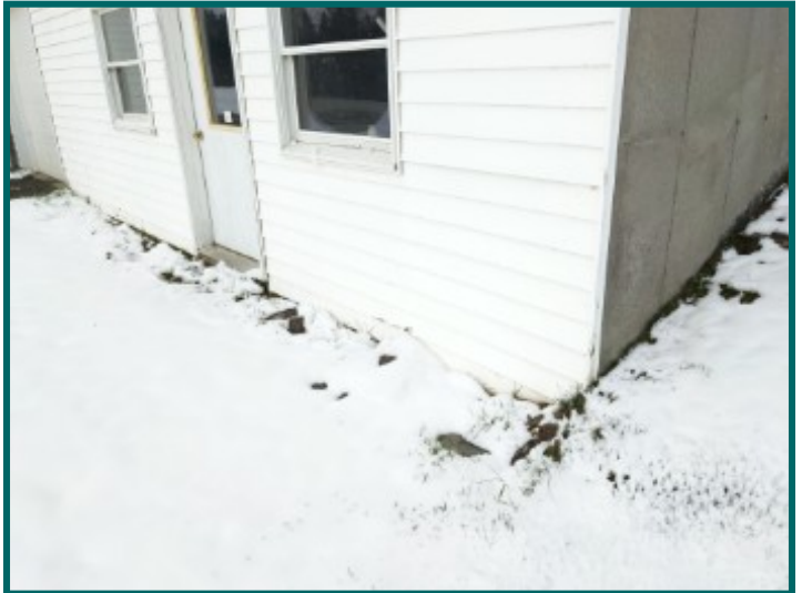
Damaged siding and siding in contact with ground at right side of building
