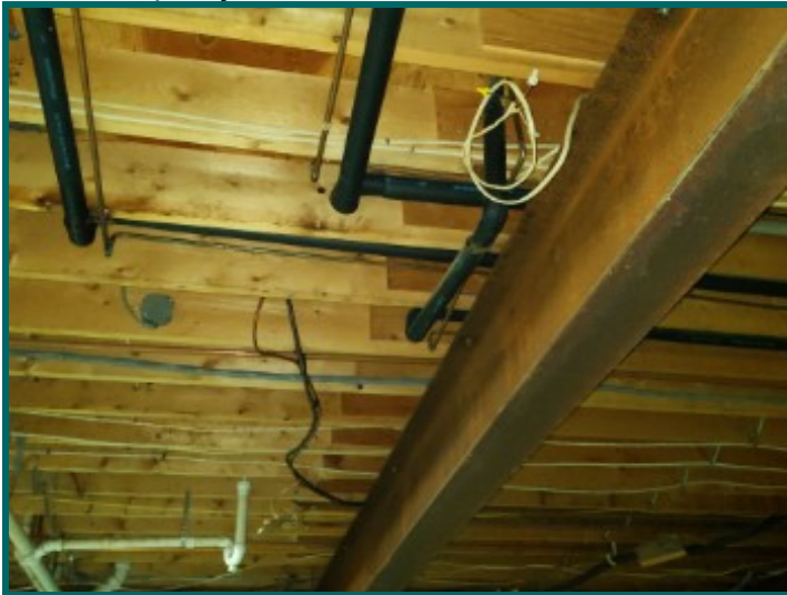
Improperly terminated wires in basement.
