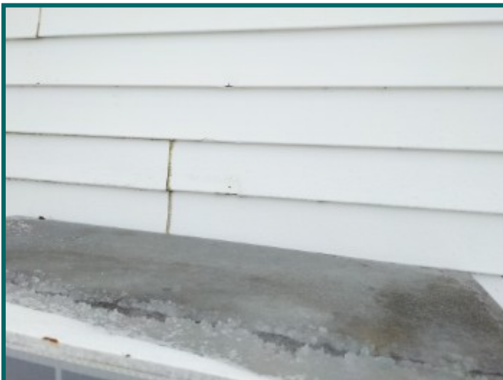
Damaged siding and staining on siding in front of building.
