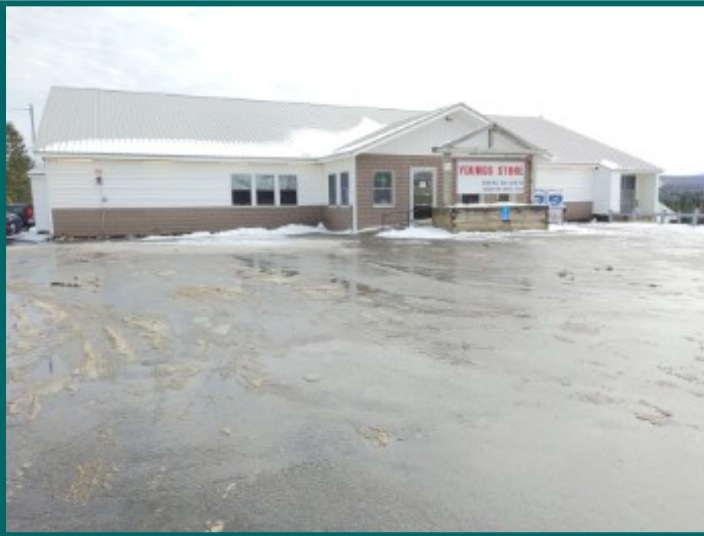
Neutral grading at front
