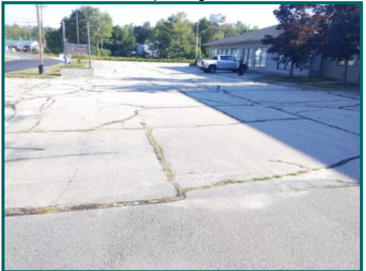
Cracks / damaged surface at front and left side of building
