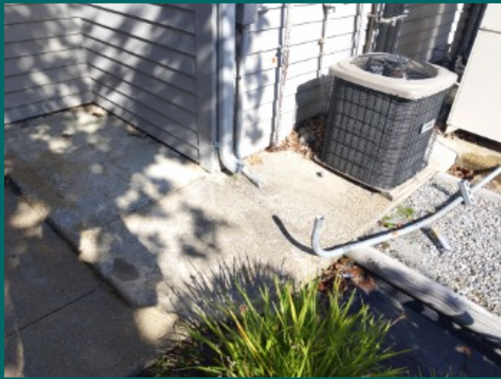
Gutter terminates onto walkway at rear of building.
