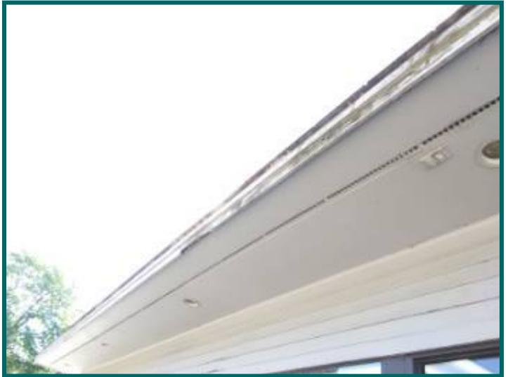
Deterioration to trim at left side
