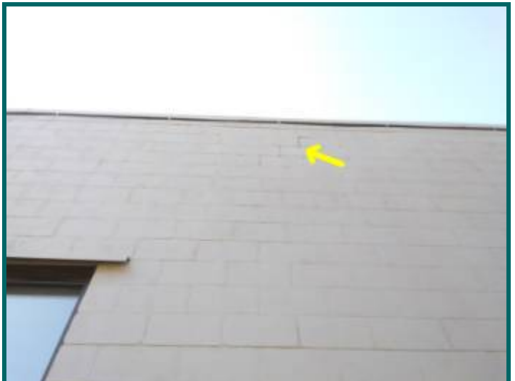
Step cracking rear left
