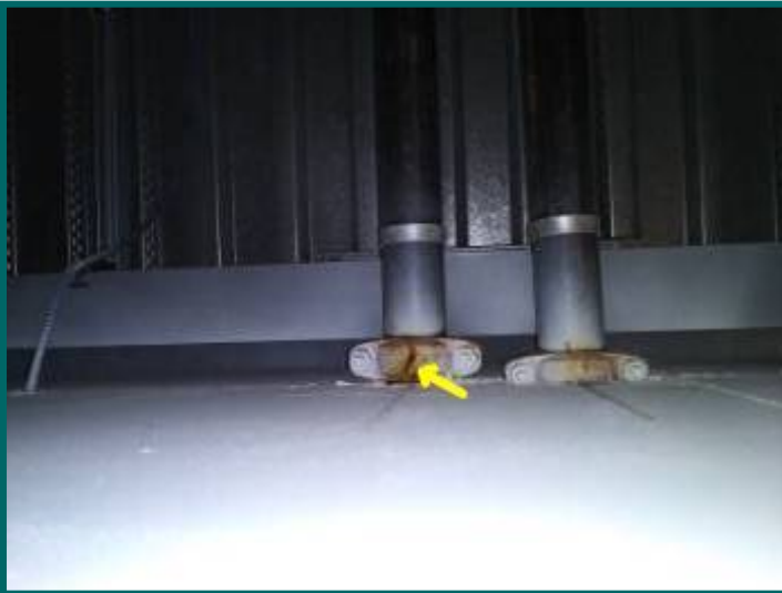
Leak / wet condition at plumbing above right rear office middle building
