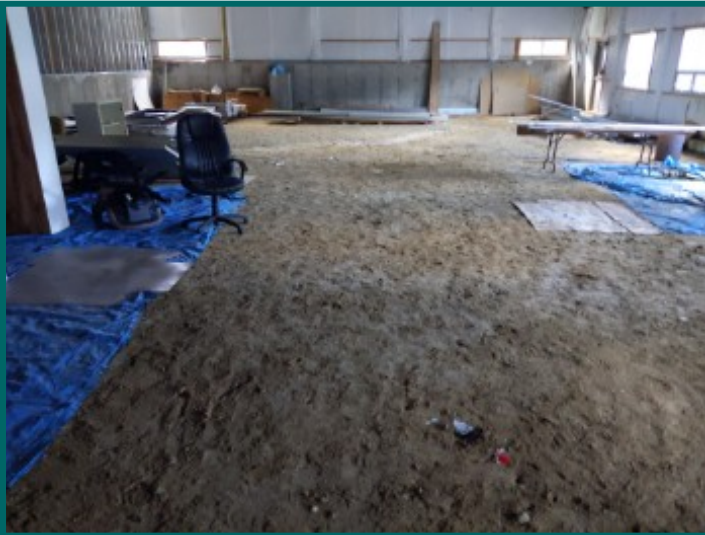
Incomplete finish / dirt floor without vapor barrier at front right.
