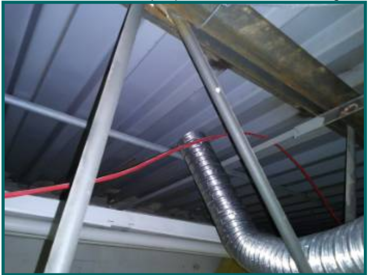
Inproper bath fan termination middle rear bath
