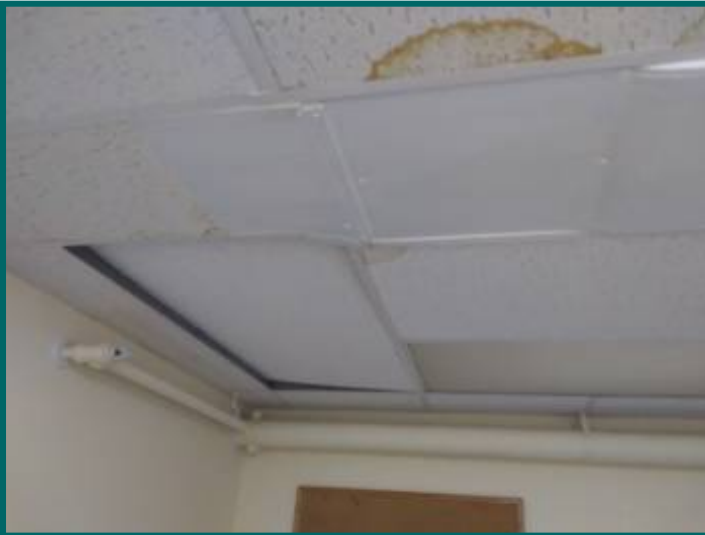
Stains on ceiling tested dry at left building Brad Wuorinen office
