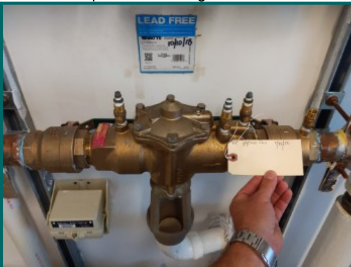
Backflow prevention and most recent service tag
