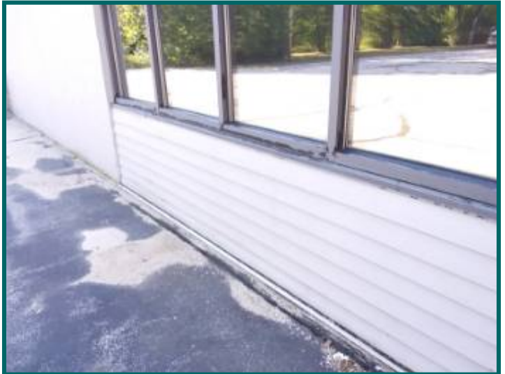
Peeling paint at left rear
