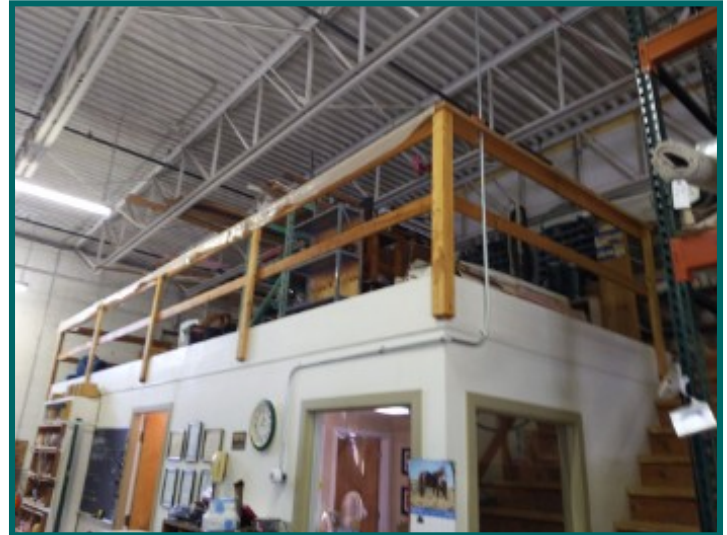
Unsafe rail openings at neatly done mezzanine.
