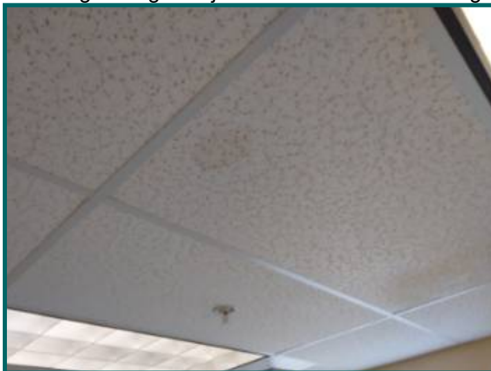
Stains on ceiling tested dry at front middle office
