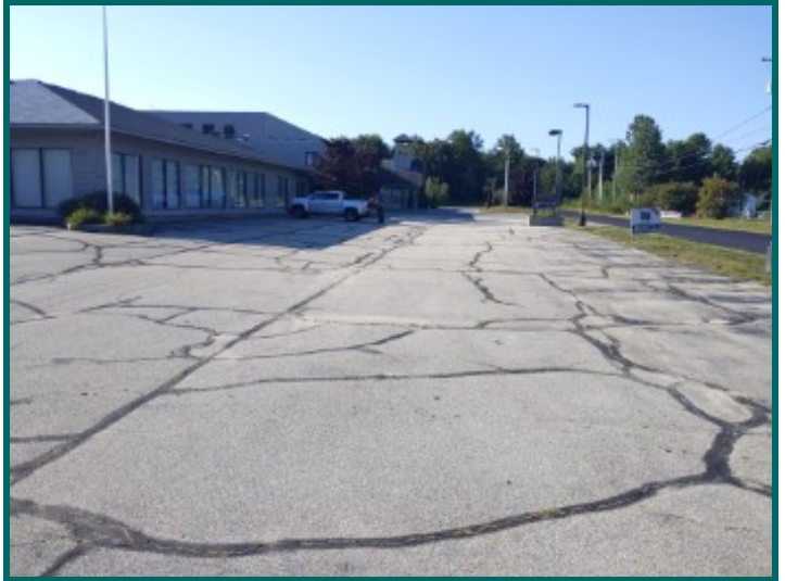
Damaged asphalt surfaces throughout left side parking.
