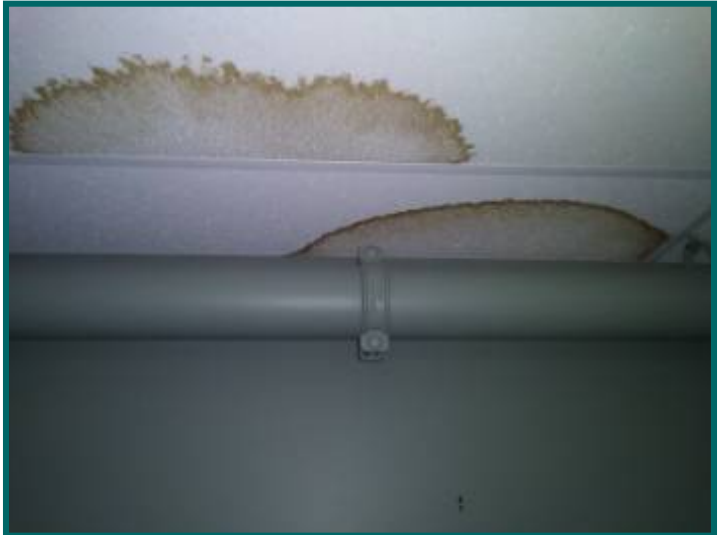
Stains on ceiling tested dry at left building middle
