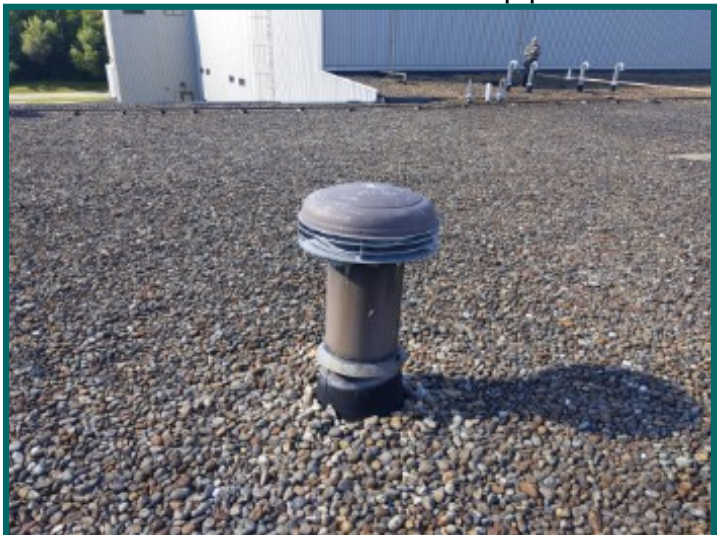
Modine / Neatly done heater vent termination.
