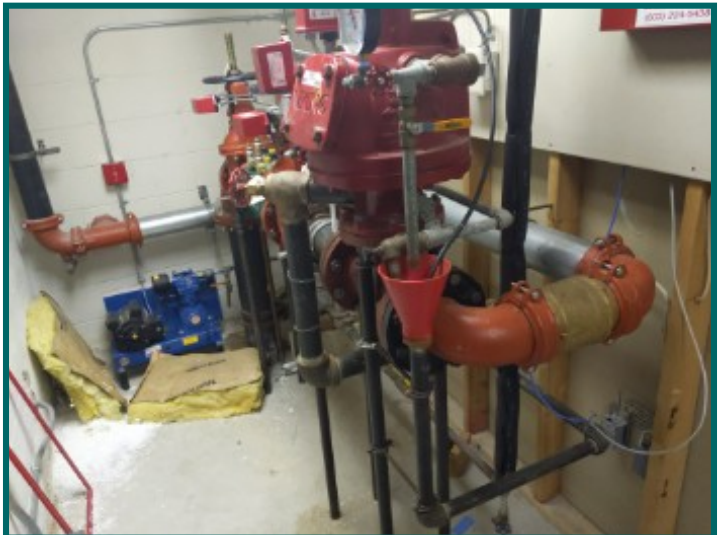
Fire suppression equipment in left building sprinkler room
