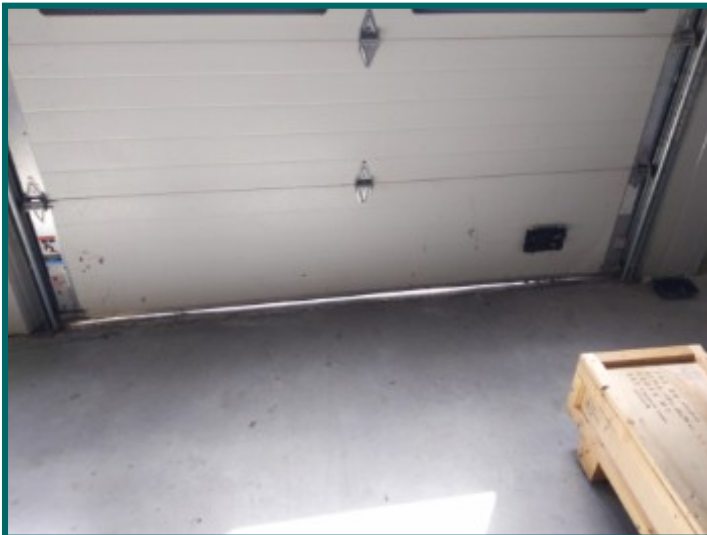
Impact damage at rear overhead door/door does not seal well
