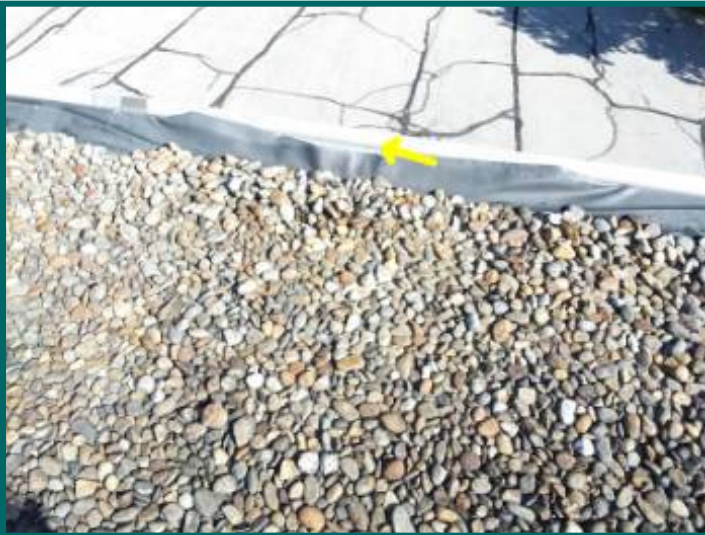
Damaged rubber roofing middle building
