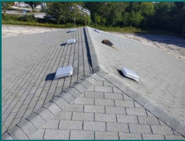
Ridge vent and can vents at left building
