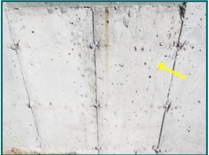
Vertical crack on side wall.
