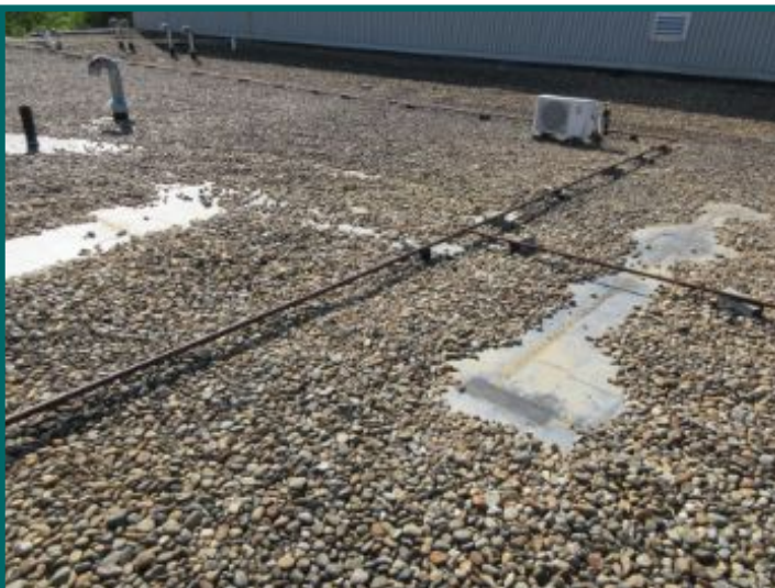
beyond design life / water intrusion at interior
