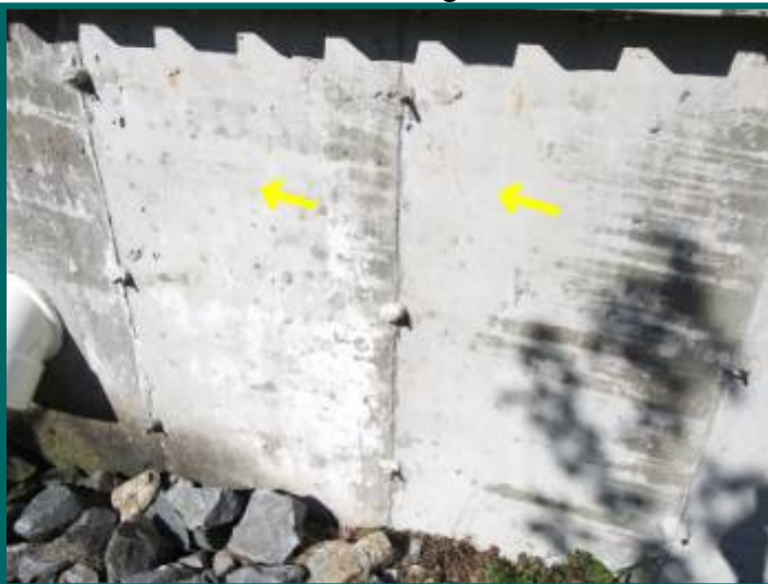
Vertical crack on rear wall
