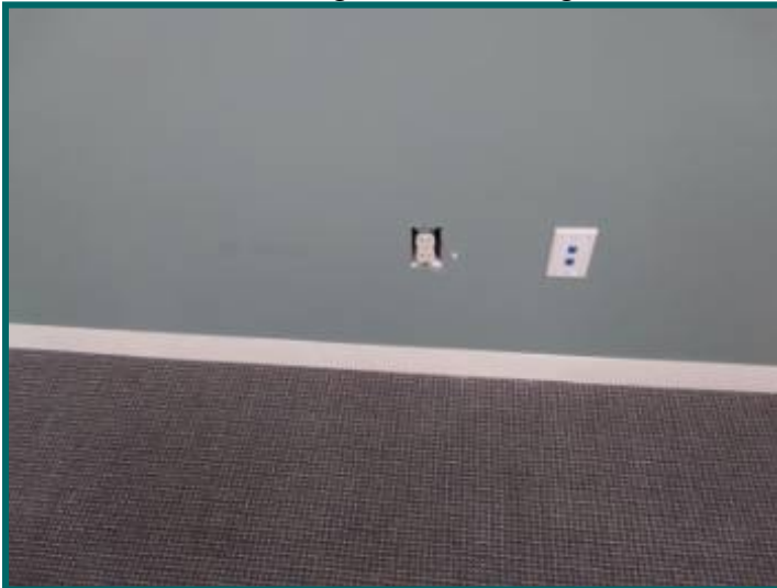
Missing plate cover left building rear
