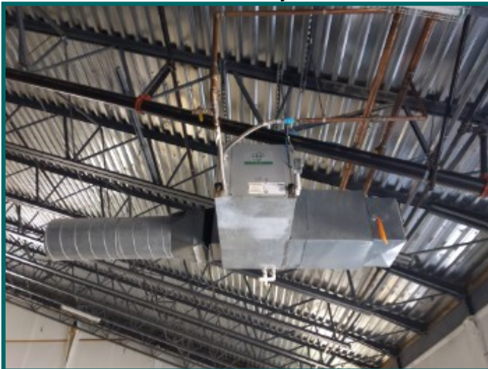
heat pumps located throughout front right, all units were 15 years old
