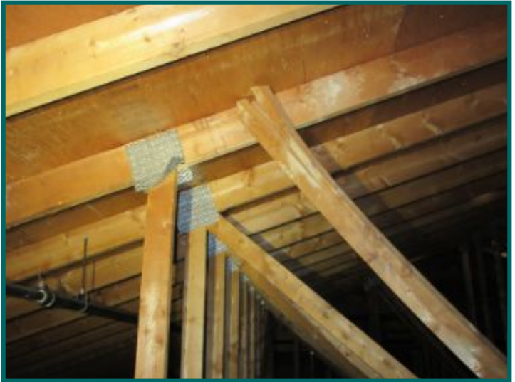
Damaged truss in left building attic
