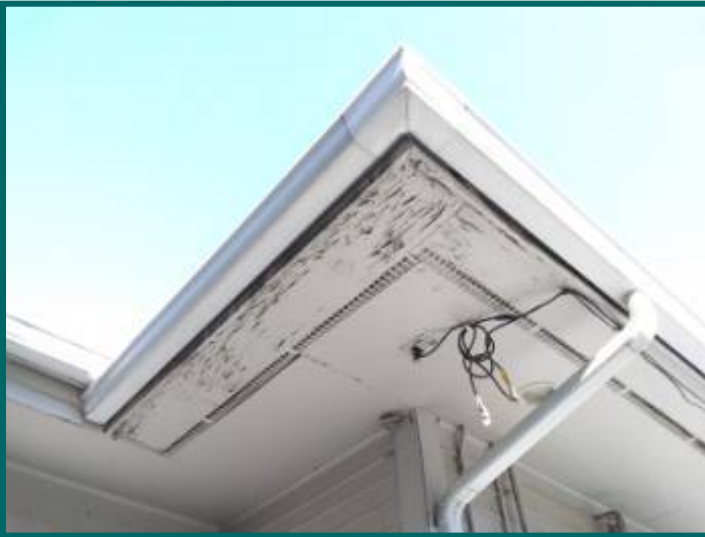
Damage, rot on trim at rear
