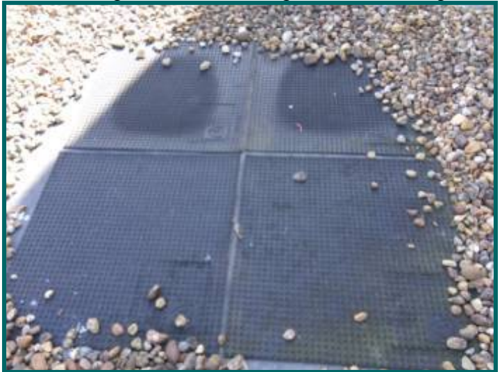
Areas of missing ballast and prior repairs at middle building
