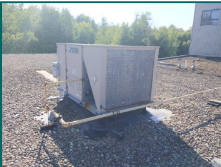
Rooftop unit at rear of middle building, 17 years old
