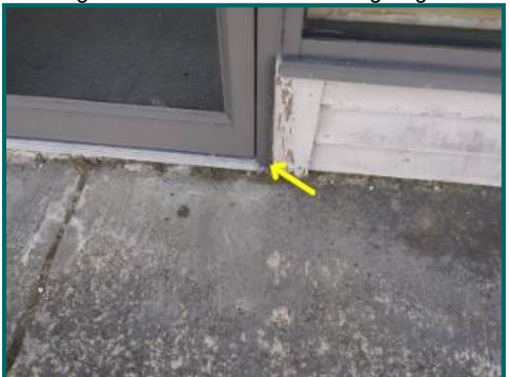
Damage, rot on trim at left side
