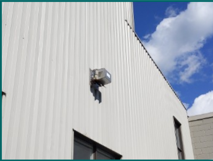
Boiler vent termination
