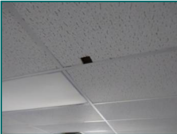
Damaged ceiling tiles at mount Washington room
