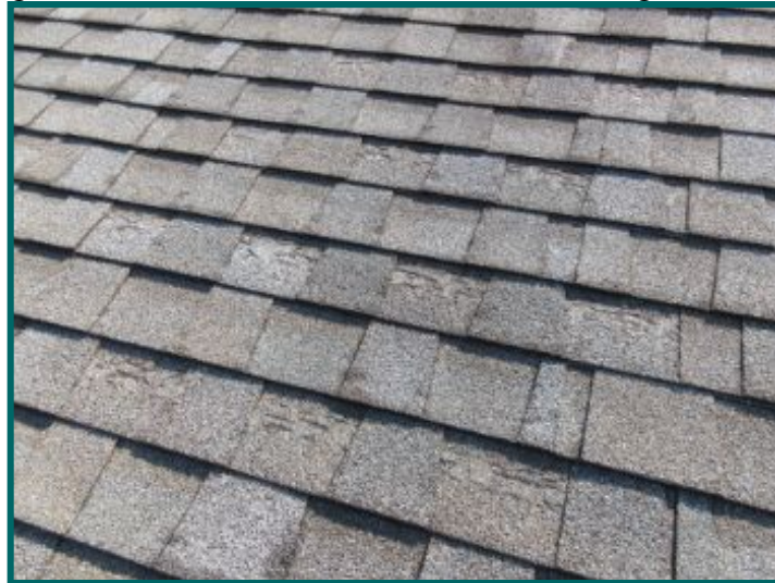
damaged surface at right building front roof
