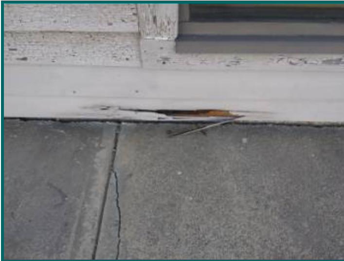
Damage to exterior surfaces in contact with finished grade at left front.
