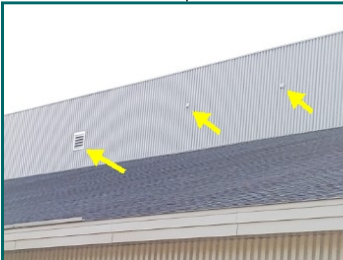
ERV vent termination and bathroom vent terminations
