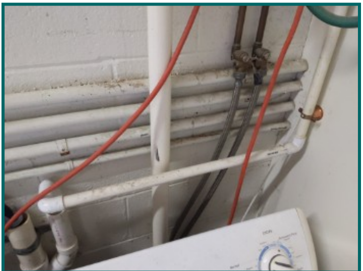
Steel mesh burst proof laundry hoses.
