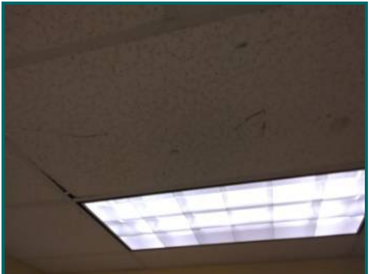
Damage to ceiling at left rear office middle building
