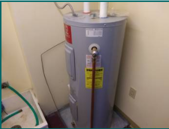
Warehouse water heater 30 gallon 16 years old
