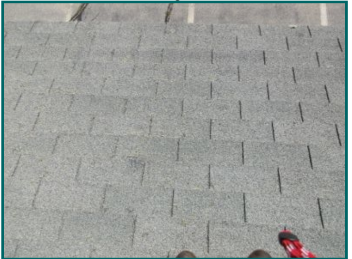
damaged surface / granular loss at left building roof
