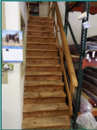
Missing graspable handrail and unsafe rail openings at Neatly Done.
