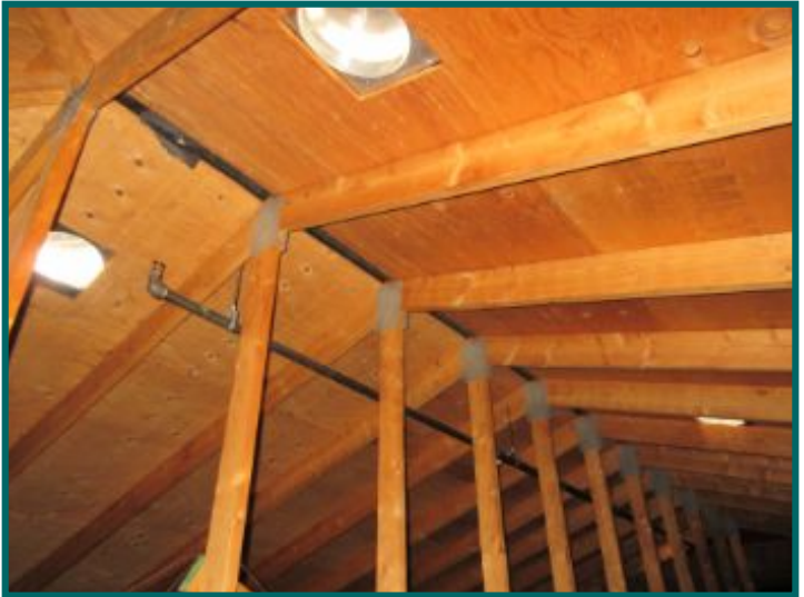
ridge vent and can vents in left building attic
