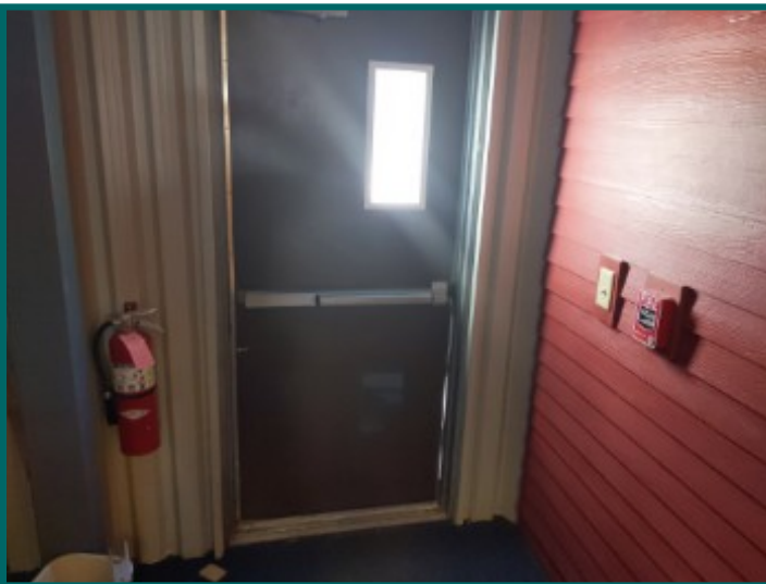
Rear door does not seal well
