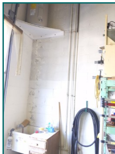
Water staining / efflorescence at neatly done rear wall
