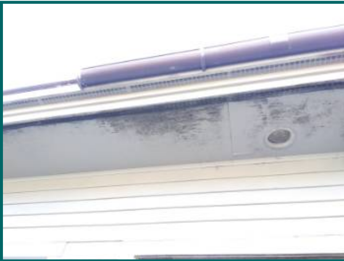
Damage, rot on trim at left front
