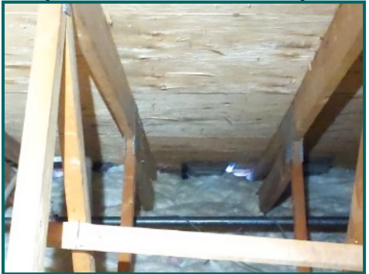
Soffit vents with propa vents at left building
