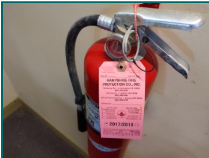
Fire extinguisher tag is expired
