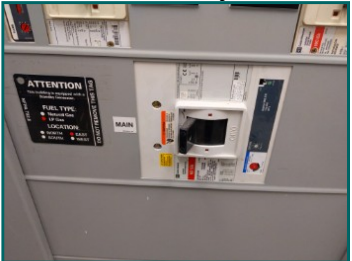
1200 amp three-phase 600 volt service disconnect switch
