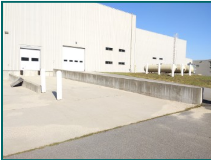
Retaining walls at rear loading dock
