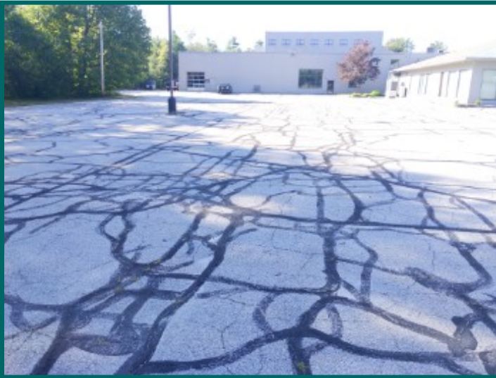
Asphalt surfaces at rear / left side of building appear to be beyond their design life.
