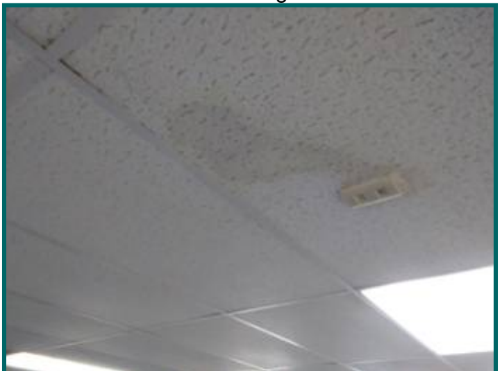
Stains on ceiling tested dry at Mount Washington room
