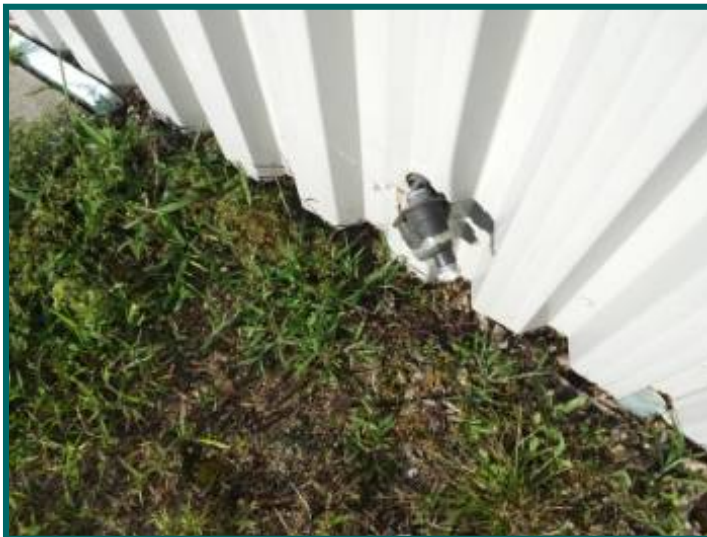
Damaged faucet handle at rear
