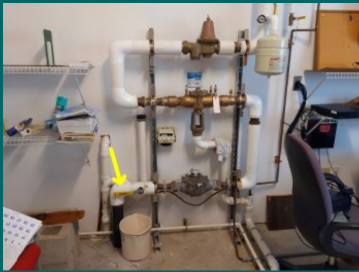
Main water shut off valve / water meter and backflow prevention at right side front room
