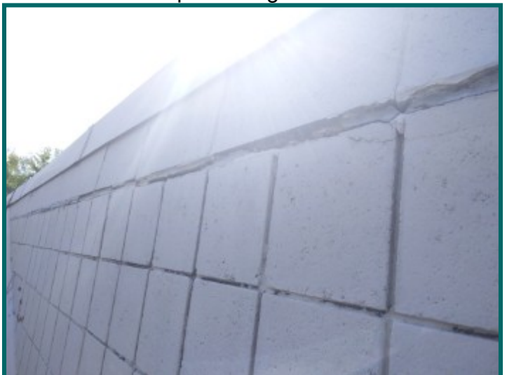
Damaged block / horizontal cracking at front / left side of middle building
