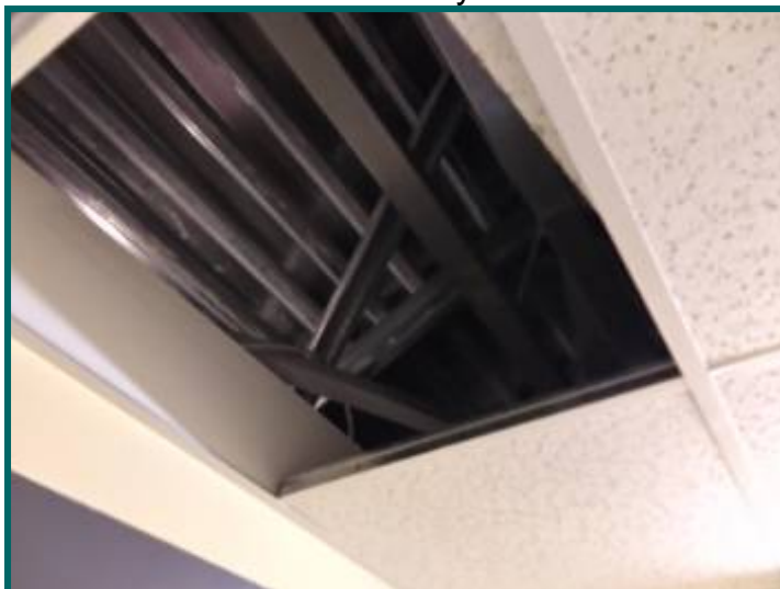
Missing ceiling tiles janitor room middle building
