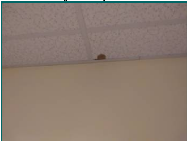
Stains on ceiling tested wet at right rear middle building
