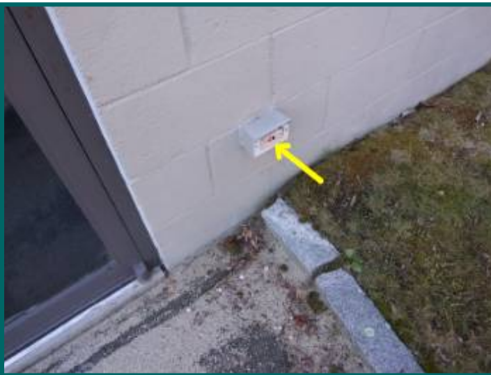
Missing weather proof outlet cover at warehouse
