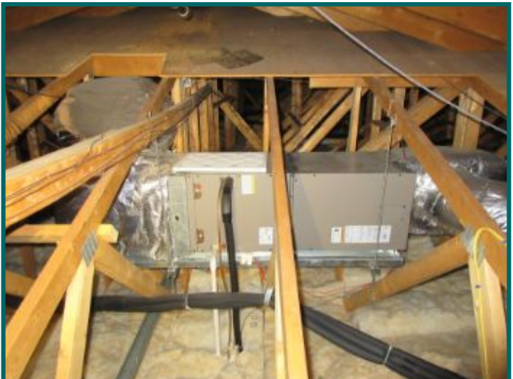
Unable to test left building HVAC, shut down / not operational at the time of inspection. Air handler in attic space above left building, 11 years old
