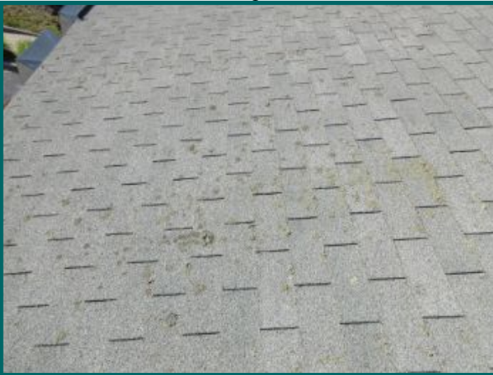
damaged surface / granular loss and fungal growth at left building
