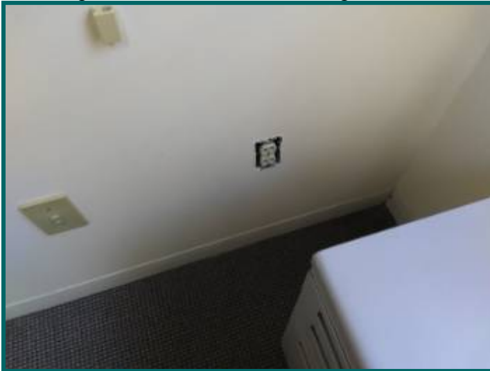
Plate covers missing at left building front office.
