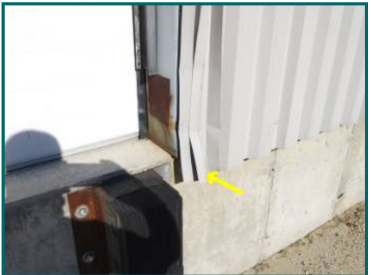
Damage to exterior surfaces at loading dock
