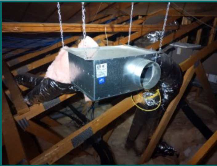
vent terminating in attic at left building
