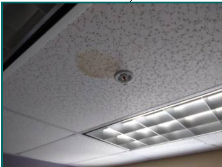
Stains on ceiling tested dry at warehouse office
