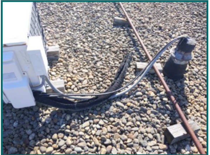
Damaged / mission insulation at rooftop mini split.
