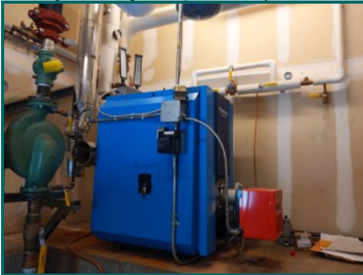
Single boiler for water source heat pumps in rear boiler room, 16 years old
