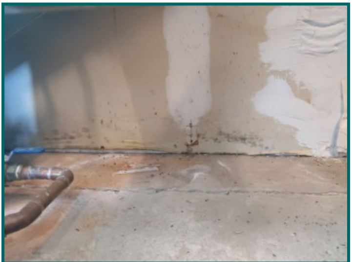
Suspected mold staining in boiler room tested dry
