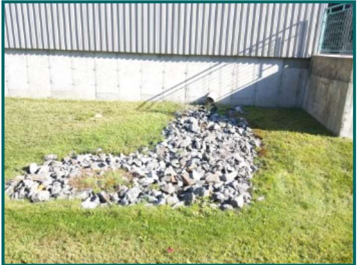
Internal roof drain termination at right side of building.
