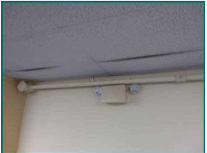
Damaged ceiling tiles at mount Washington room
