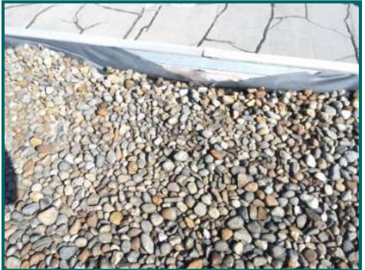
Damaged rubber roofing middle building
