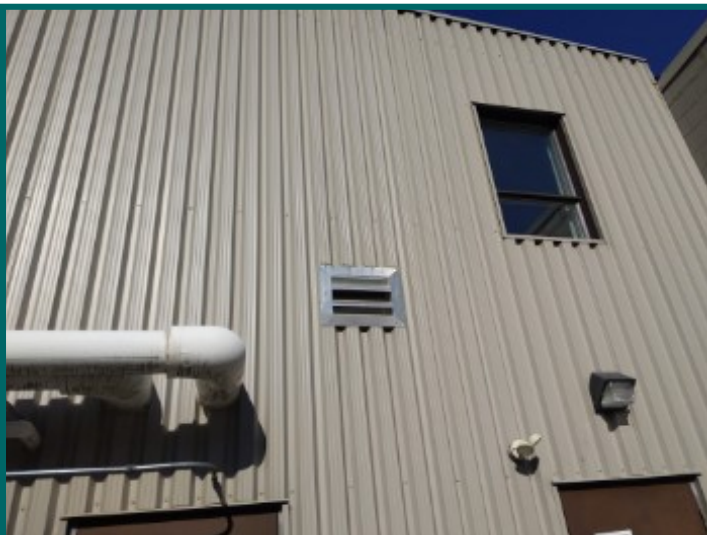
Boiler room makeup air vent
