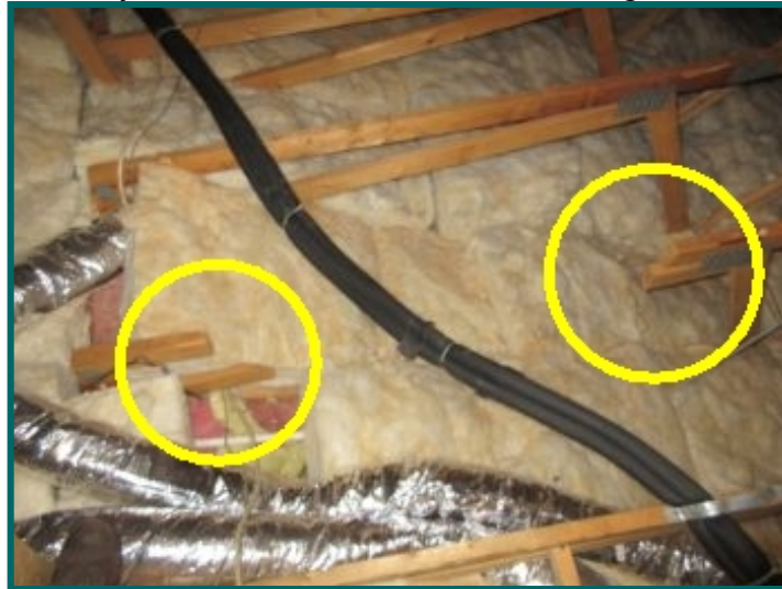
damaged / cut truss in left building attic
