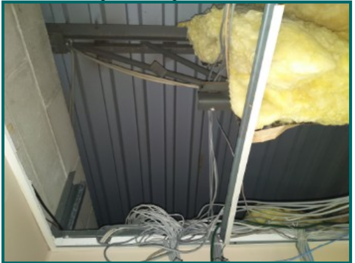
Steel frame on CMU wall at middle building
