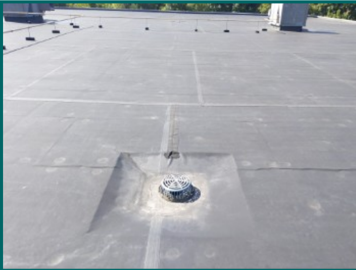
Internal roof drains at right building
