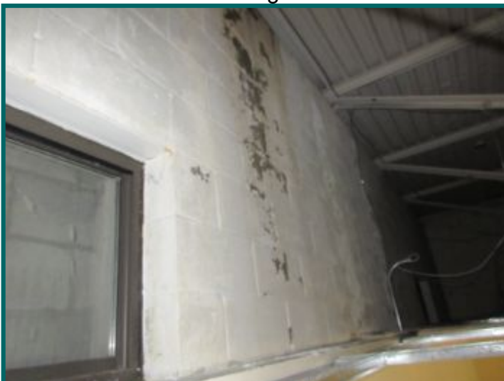
water staining / efflorescence and wet conditions at middle building right wall
