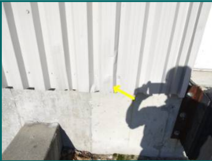
Damage to exterior surfaces at loading dock
