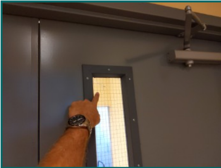
Broken glass at warehouse rear door
