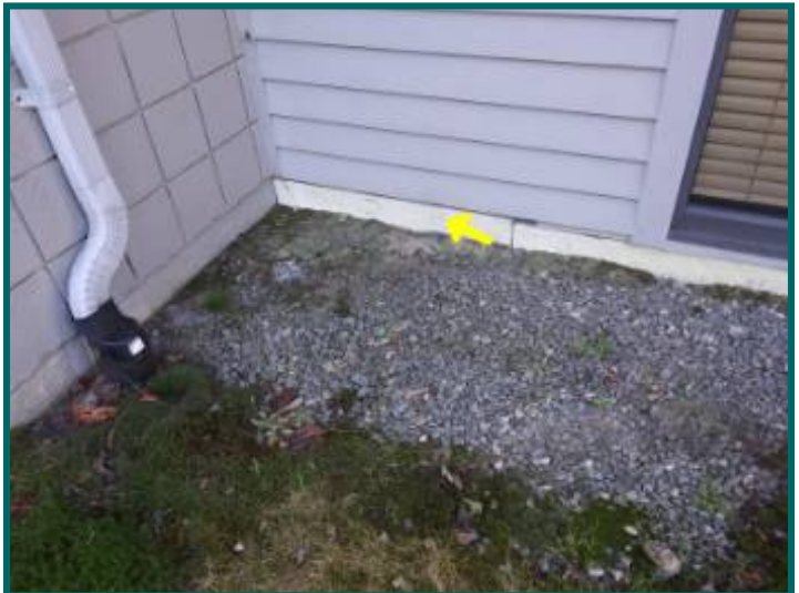
insulation in contact with ground and wood siding
