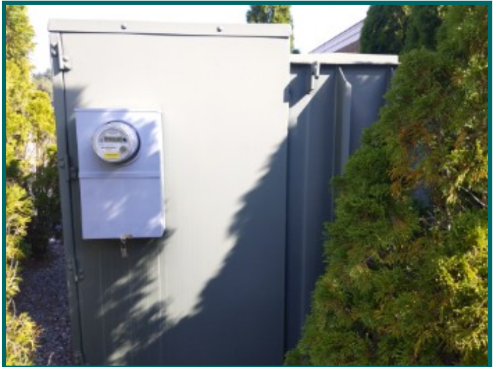
Electric meter is located at main transformer in front of building.
