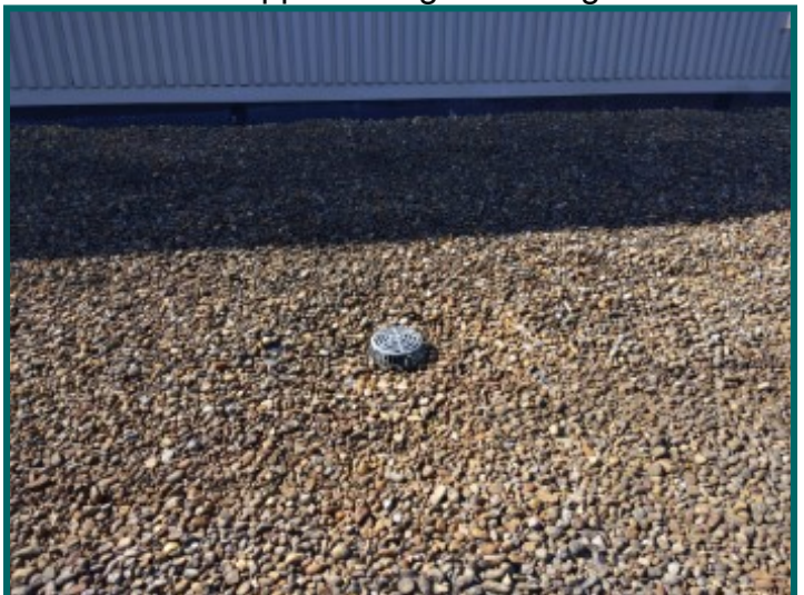
Internal roof drains at middle building. Termination was not located.
