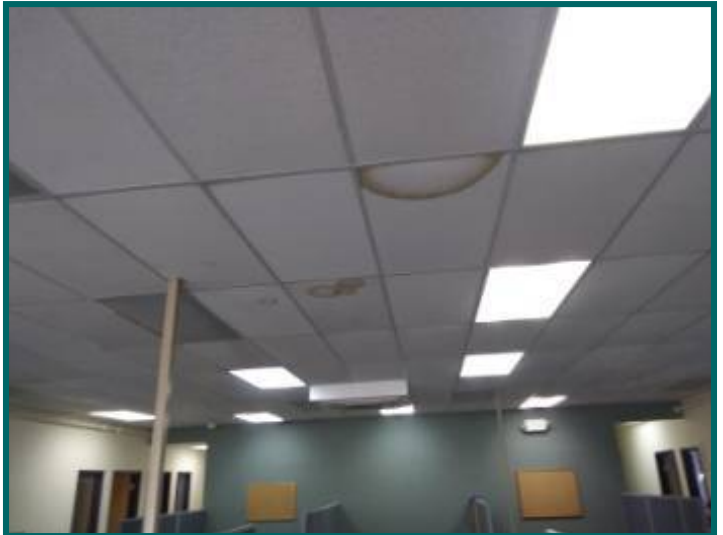
Water staining throughout left building.
