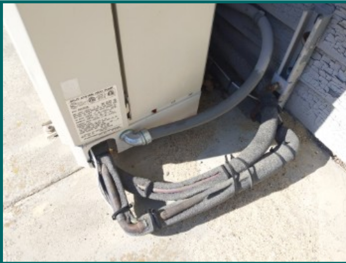
Damaged/missing insulation at rear of building.
