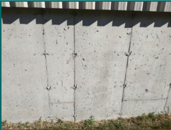
Vertical cracks at right side wall
