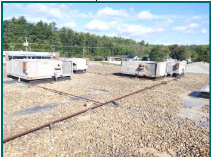
Four rooftop units at front of middle building, all 25+ years old
