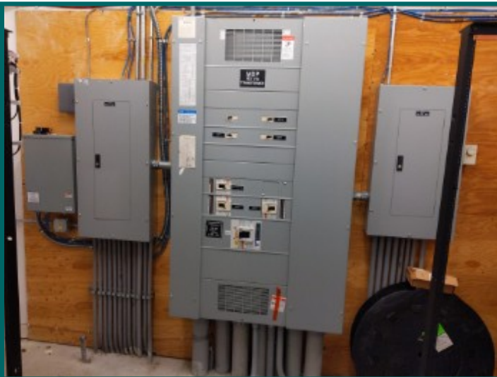
Main electric service equipment in right building electrical room.
