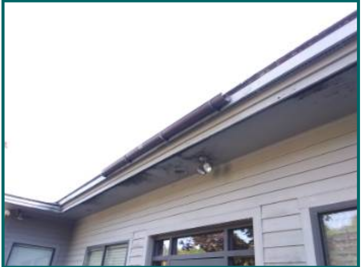
Missing downspout on gutters
