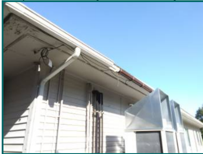
Missing downspout on gutters
