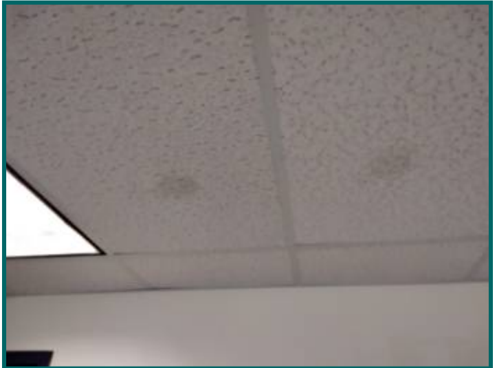
Stains on ceiling tested dry at middle office
