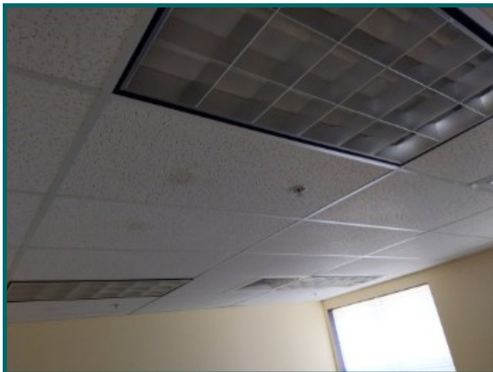
Water staining at right building front office ceiling tested dry
