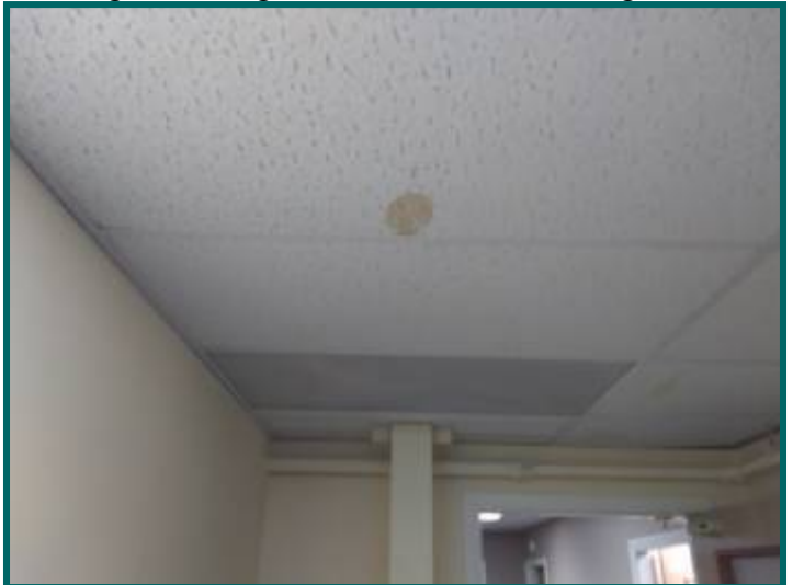
Stains on ceiling tested dry at Mount Monadnock room
