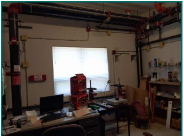
Plumbing riser for fire suppression system
