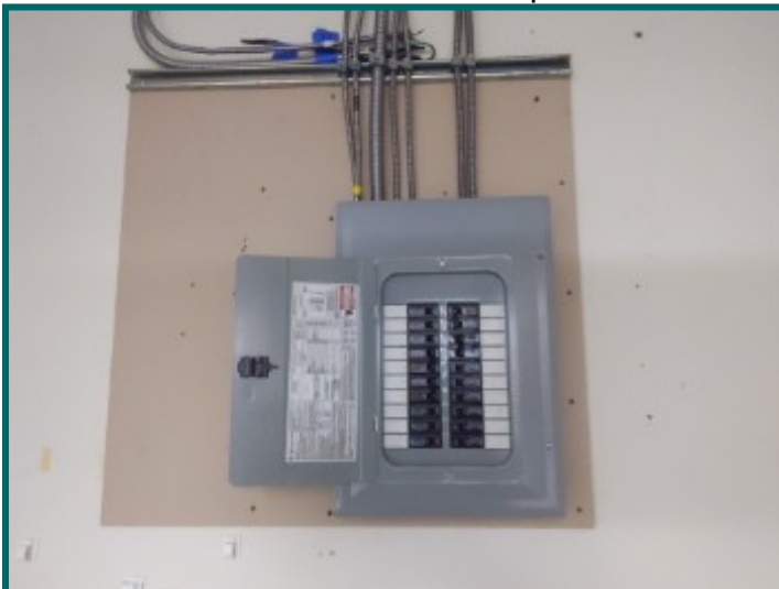
Left building computer server room electrical panel
