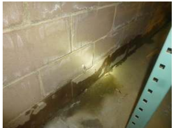
Water Intrusion (South Wall)
