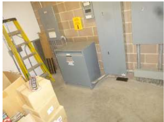
Sub panels and Transformer
