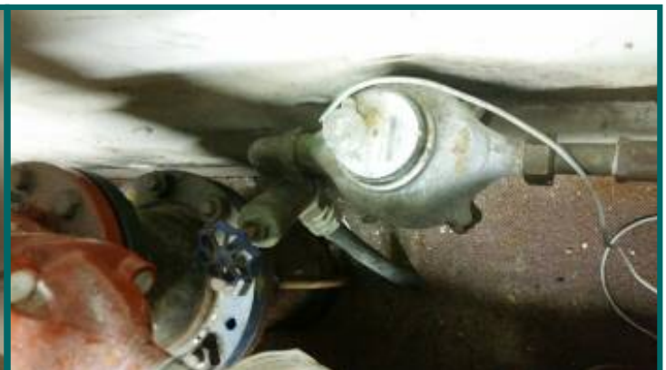
Main water shut off valve is located at water meter.
