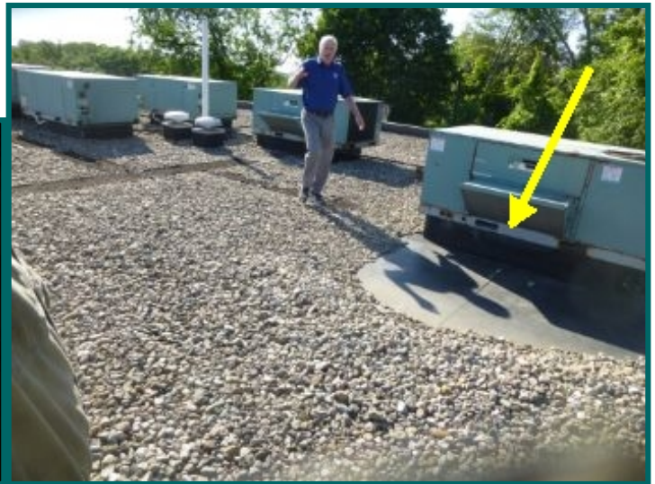
Stone ballast should be evenly spread
