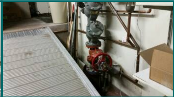
Plumbing riser for fire suppression system
