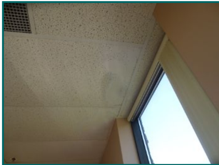
Second floor painted over stains on ceiling.
