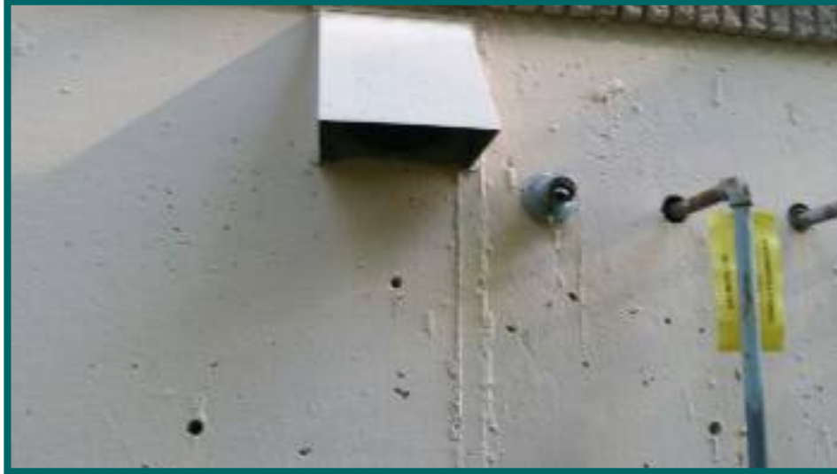
Makeup combustion air vent at rear of building
