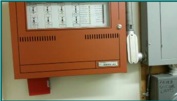
Fire suppression control panel
