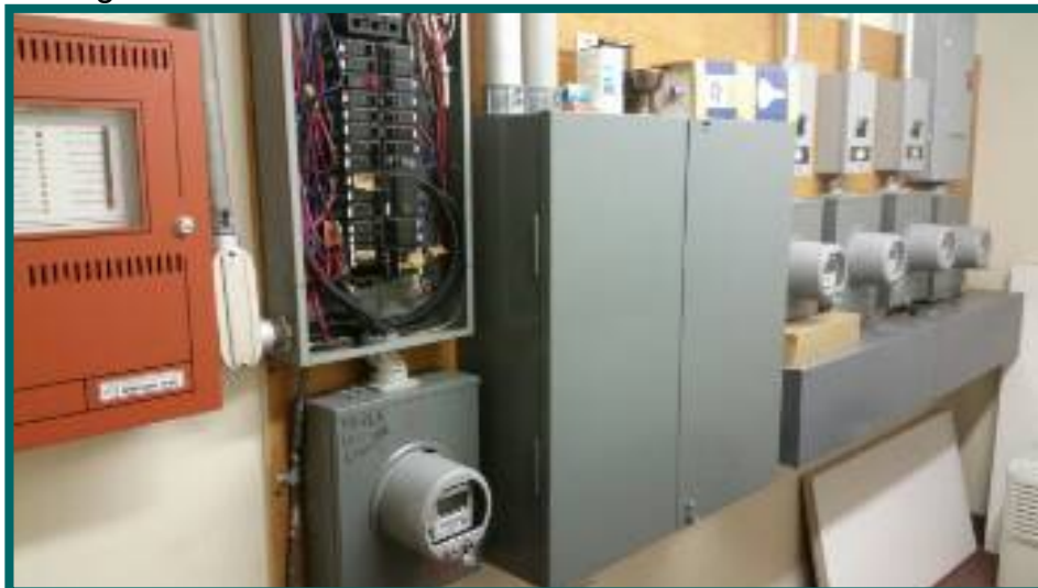
One 200 amp and four 100 amp 3 phase services in basement mechanical room
