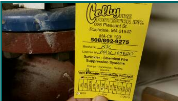
Fire suppression service tag expired in June 2011
