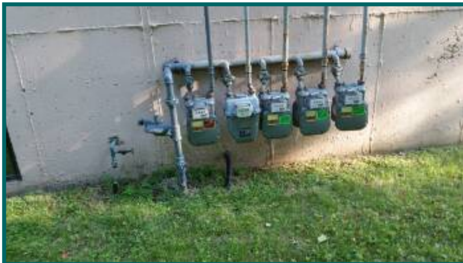
Five gang gas meter bank at rear of building
