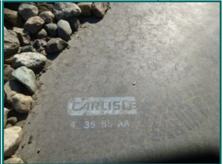
Stone ballast should be evenly spread
