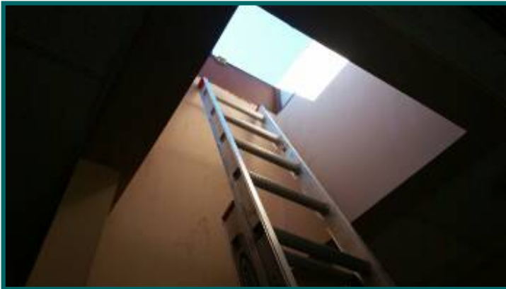
Scuttle access at second floor
