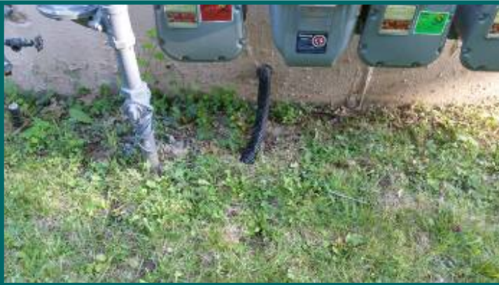
Drain line termination at rear building
