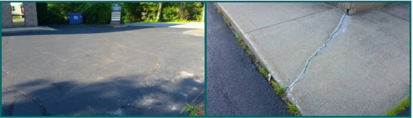
Settlement crack at front walkway
