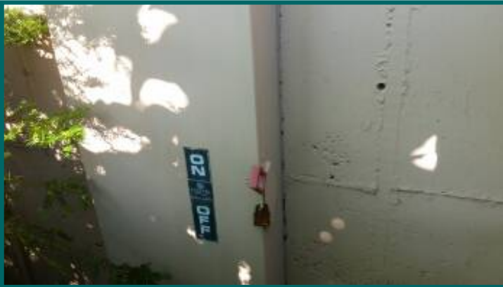
Main electric disconnect switch at left side of building is locked.
