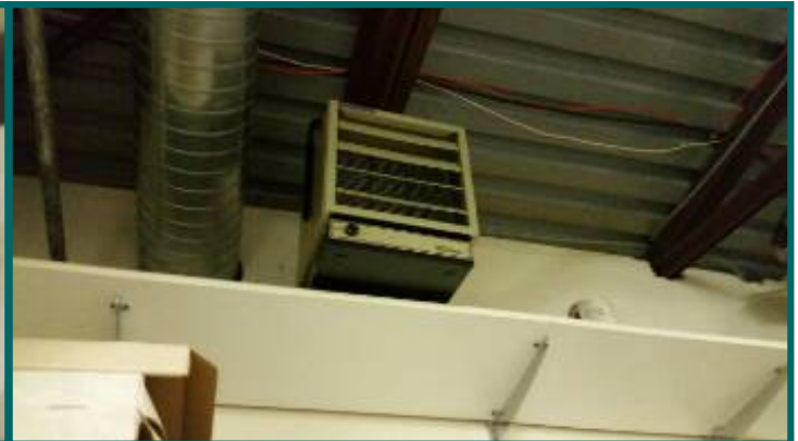
Ceiling mounted electric space heater in basement service room reported does not work.
