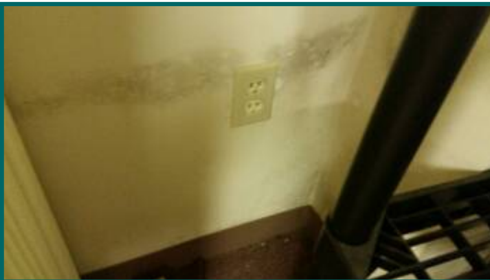
Dark staining basement wall front right corner
