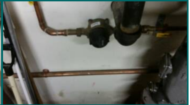
Secondary water meter for dentist office.
