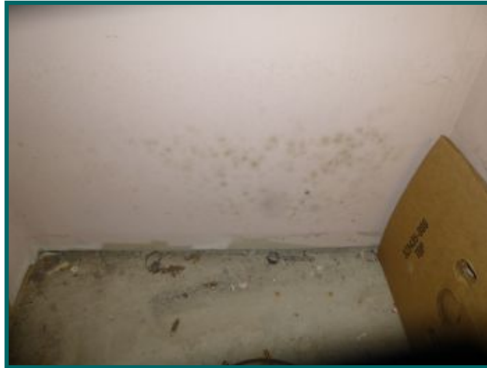
Staining in water heater closet.
