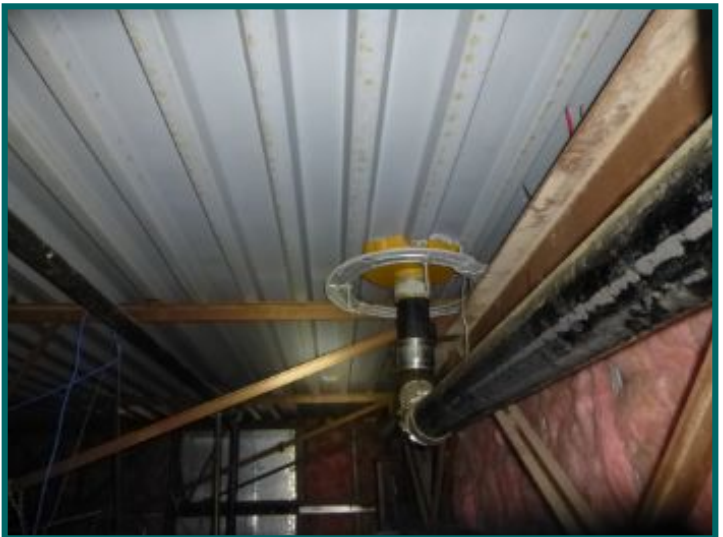
Gutter drain down pipe
