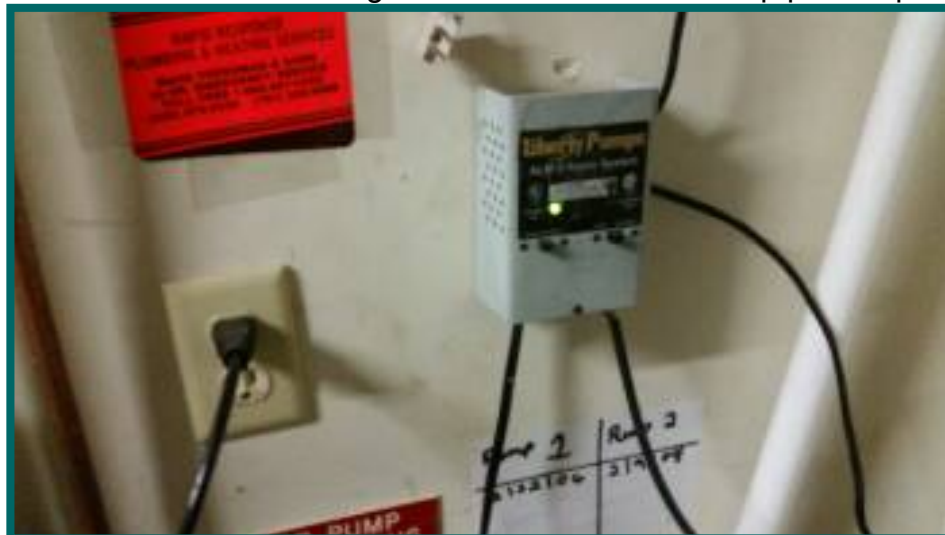
High water Alarm for sump pit
