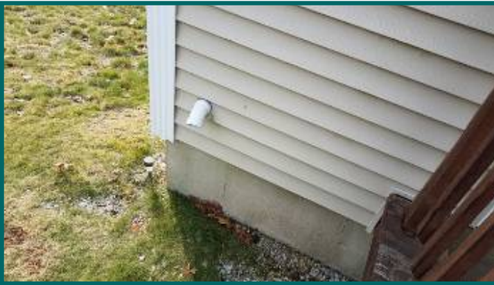
Water heater vent termination at rear wall
