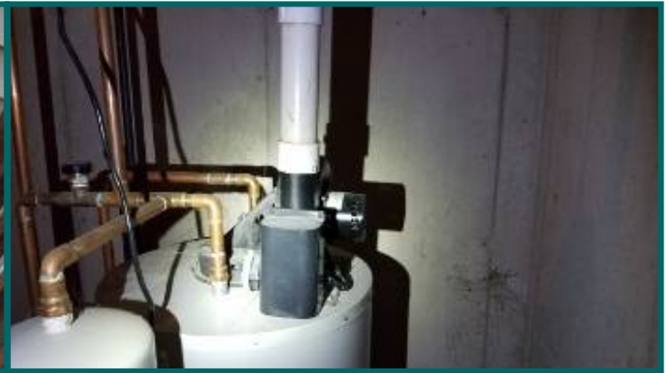
Water heater is power vented to plastic side vented pipe.
