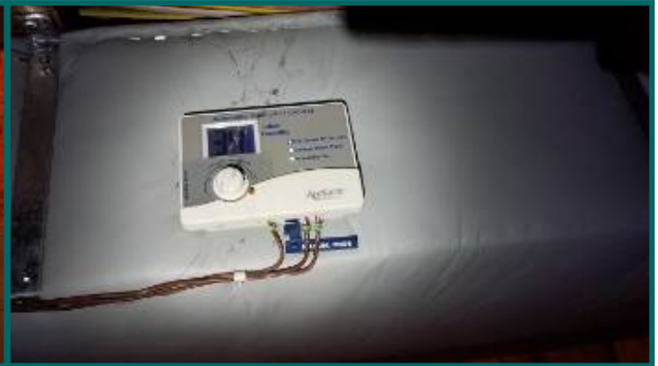
Humidistat to control humidifier located at main furnace trunk.
