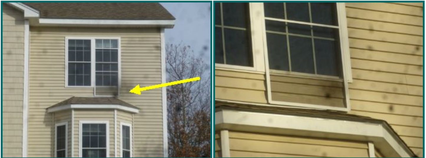
Loose or damaged screen at front window
