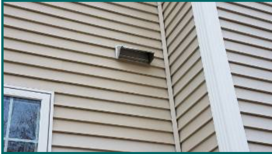
Kitchen vent termination at rear wall not in use.
