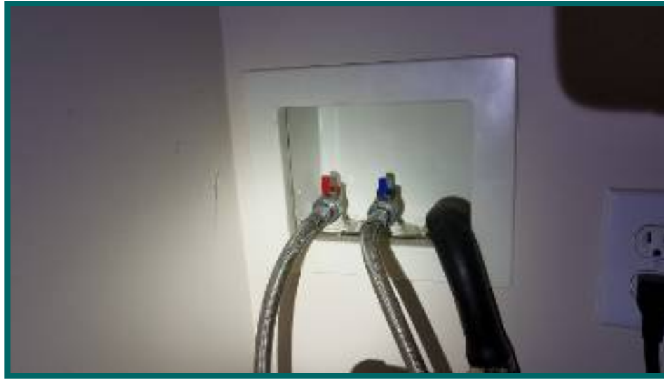
Steel mesh burst proof laundry hoses.
