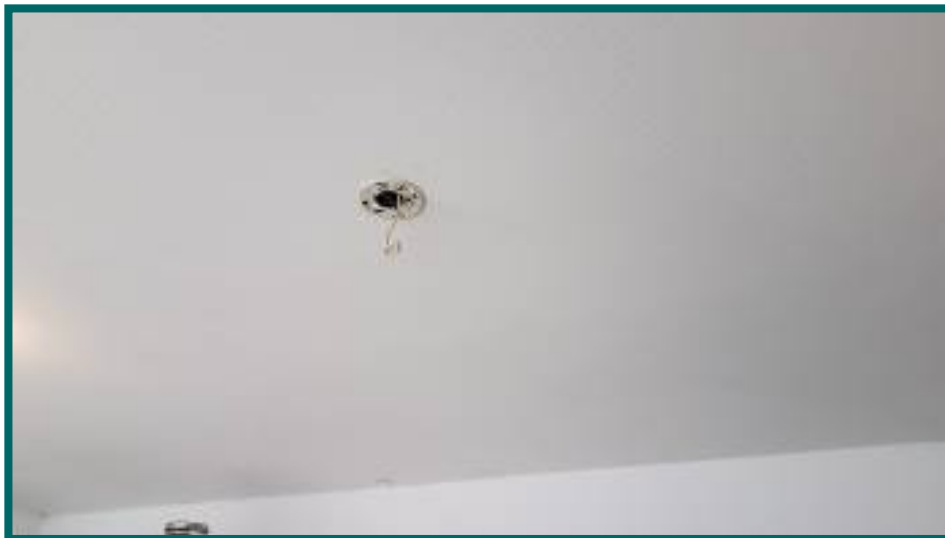
Smoke detector missing at garage
