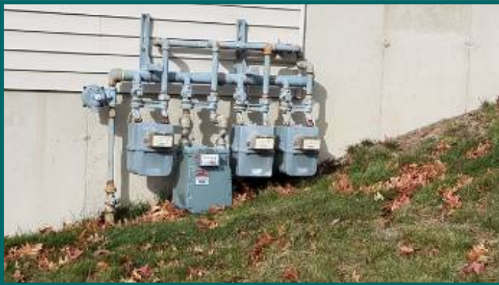
gas meters not individually labeled
