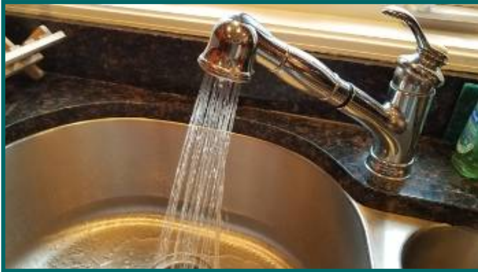
Sprayer wand does not properly divert from spray to stream
