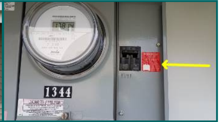
Main service disconnect at electric meter
