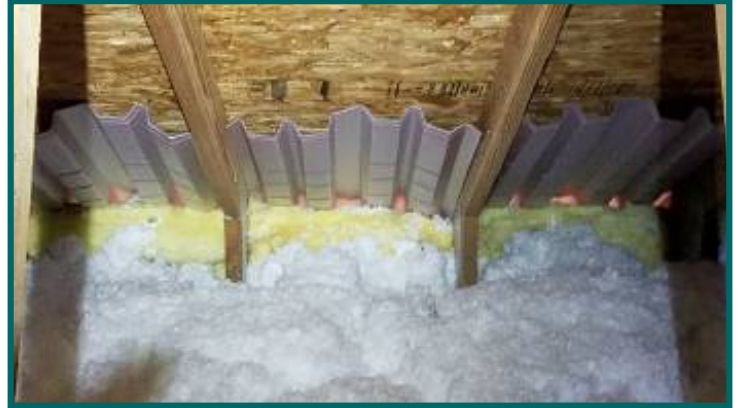
Soffit vents with propa vents
