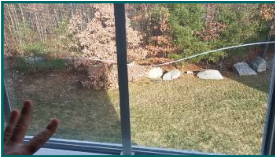
Broken glass at rear bedroom rear wall
