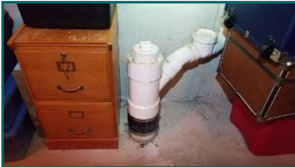
Main drain line termination
