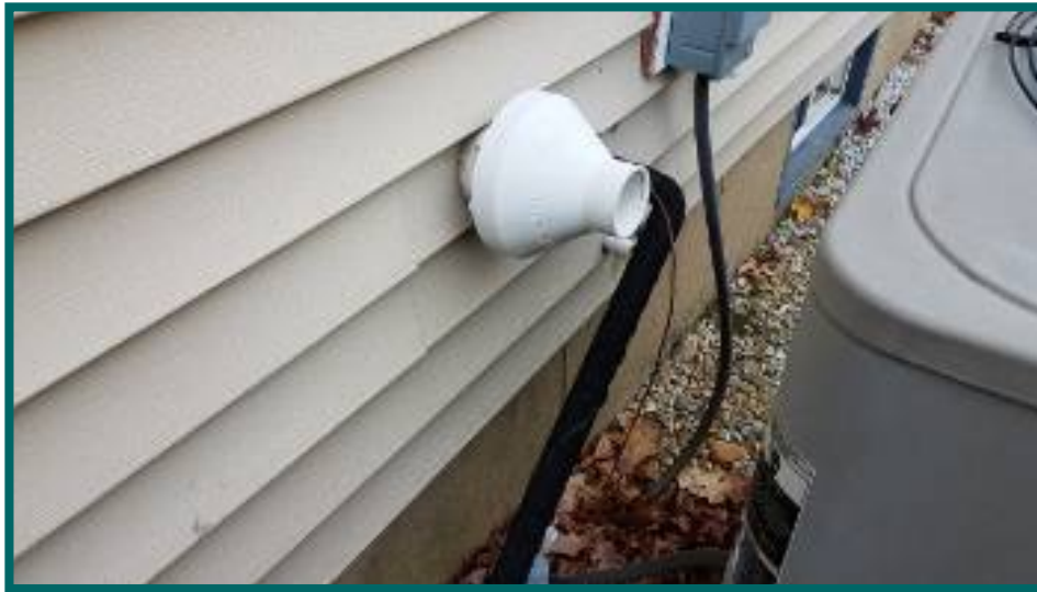
Furnace / boiler vent termination at rear wall.
