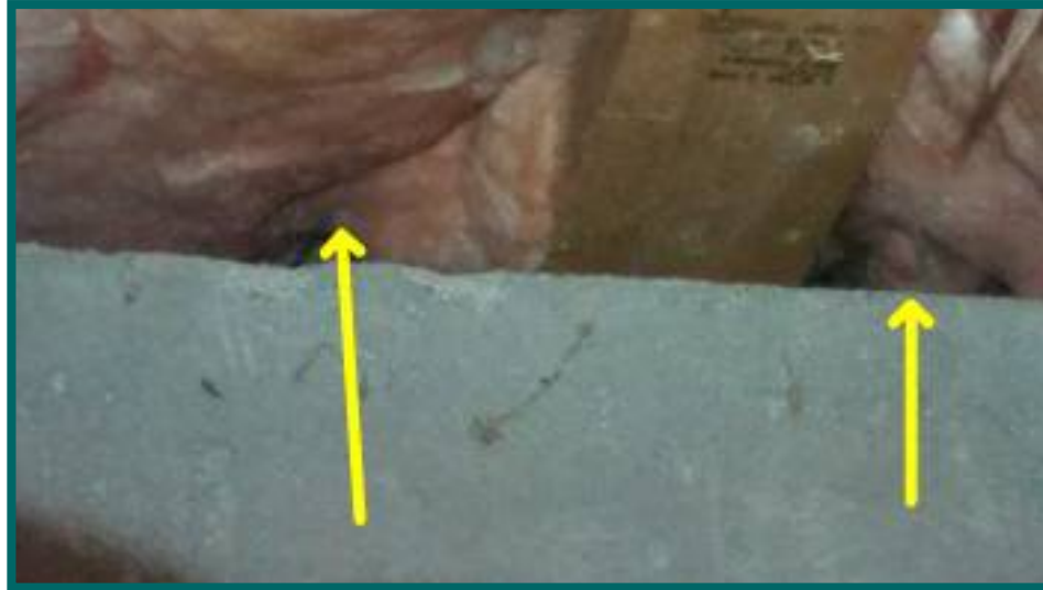
rodent tunnels in underfloor insulation along rear wall
