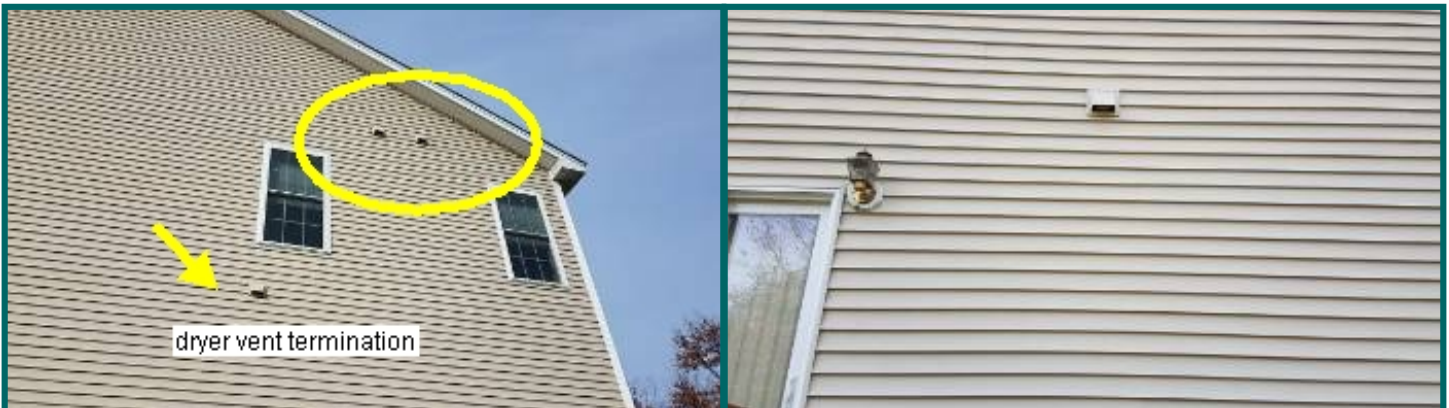
Bath fan terminations at exterior wall.
