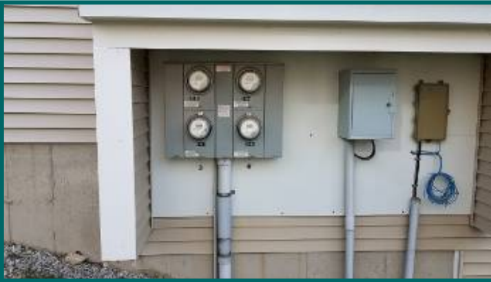
Electric meter and main service entrance
