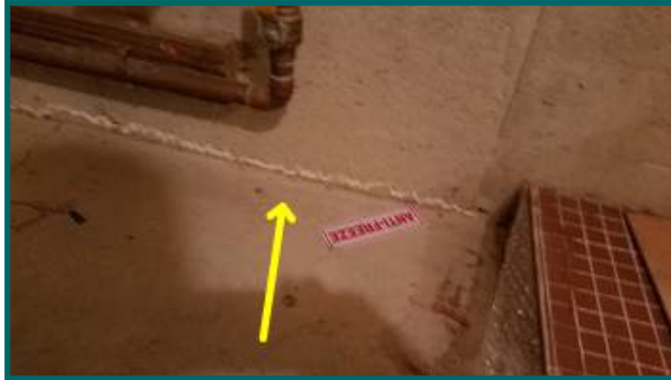
Efflorescence
