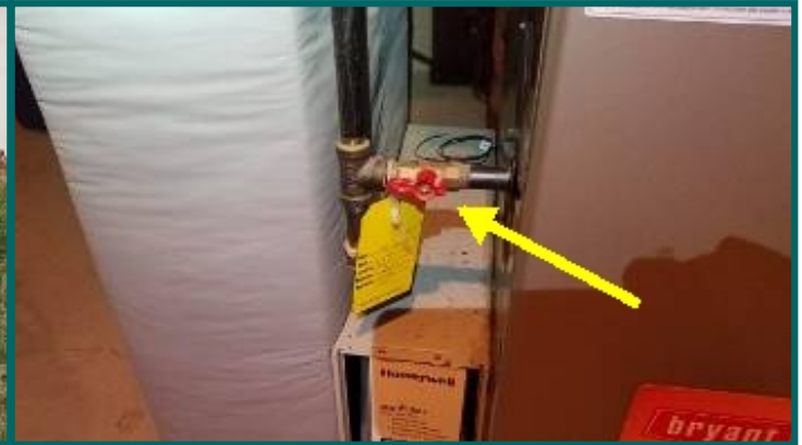
Fuel shut off located at furnace / boiler.
