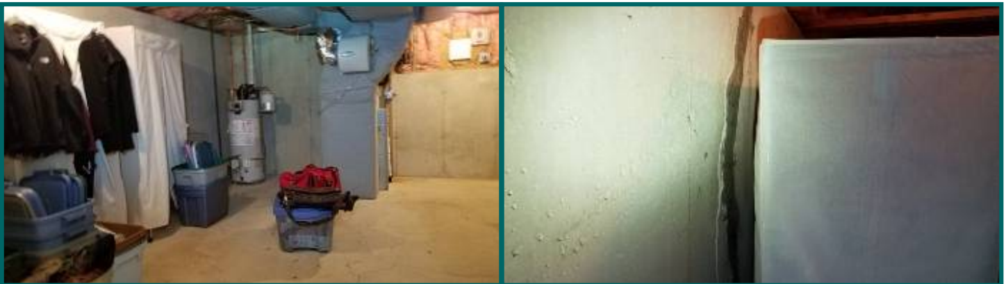
repaired crack on rear wall
