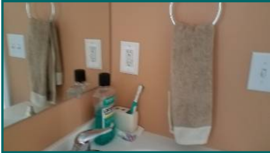
Master bath GFI outlet protects other bath outlets
