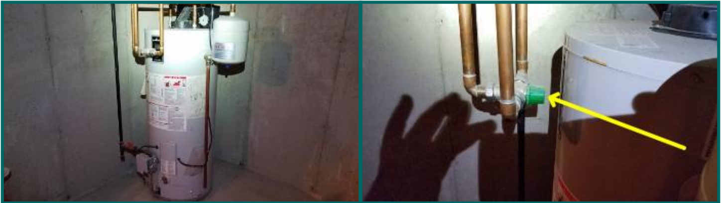
Mixing valve to adjust water temperature
