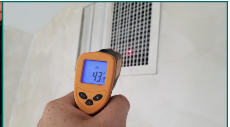
Air blowing cold at second floor
