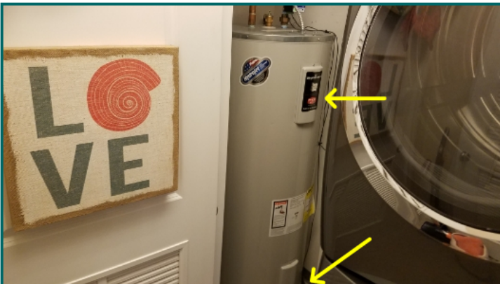
For electric water heaters temperature is adjusted by set screws behind upper and lower access covers.
