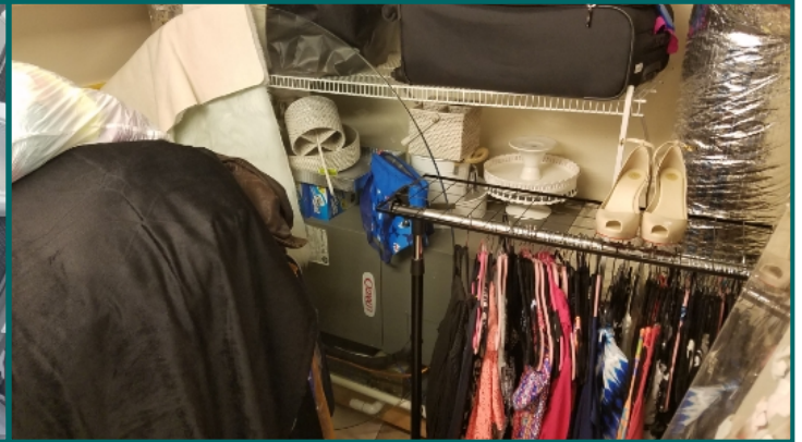
Second floor air handler providing conditioned air only. Limited inspection due to stored items.
