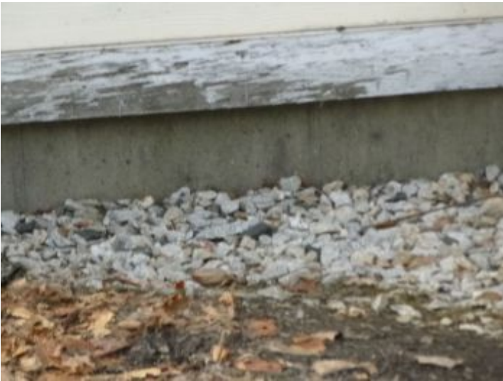
Peeling paint at front surfaces.
