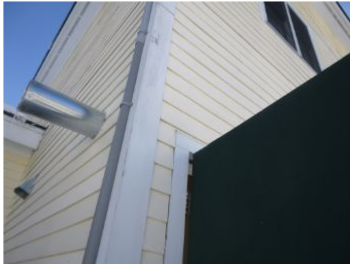
Return air and negative pressure fan vent for pool room.
