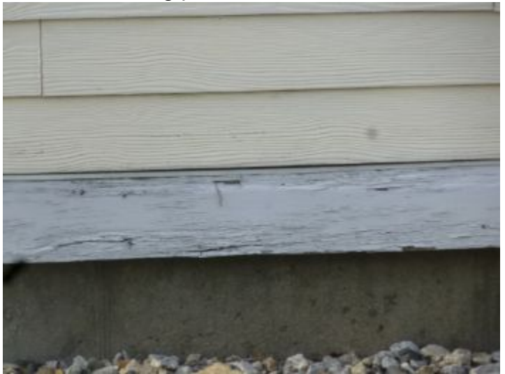
Peeling paint at front surfaces.
