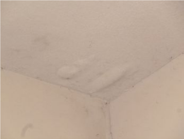
Blistering ceiling surface in garage bay,
