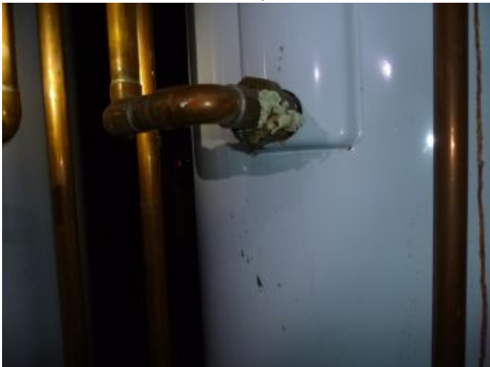
Corrosion on fitting.
