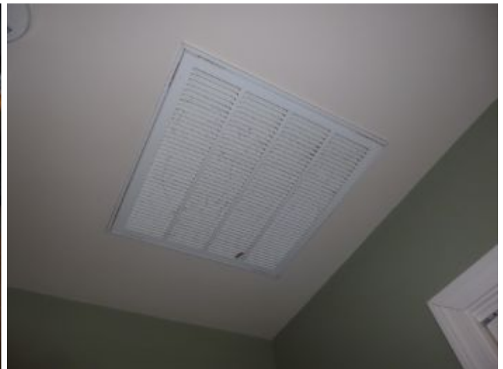
Filter access on ceiling in owners quarters.
