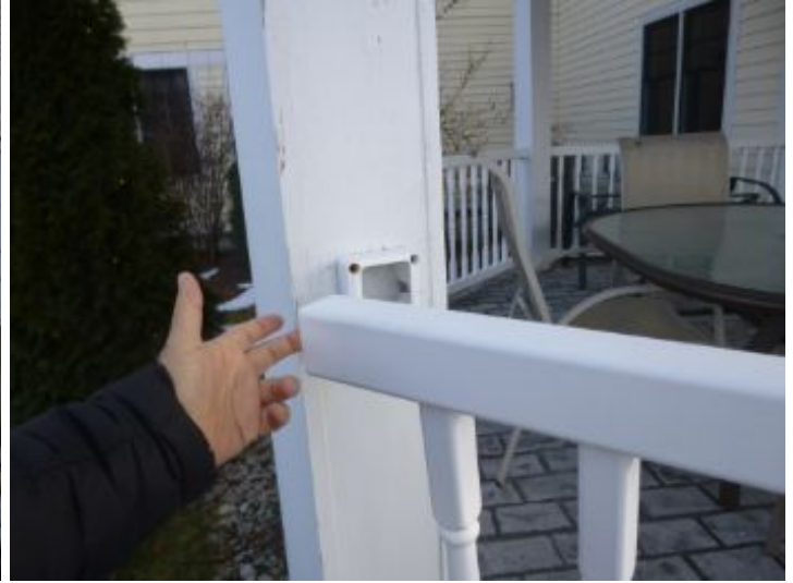
Damaged hand rail at rear of building.
