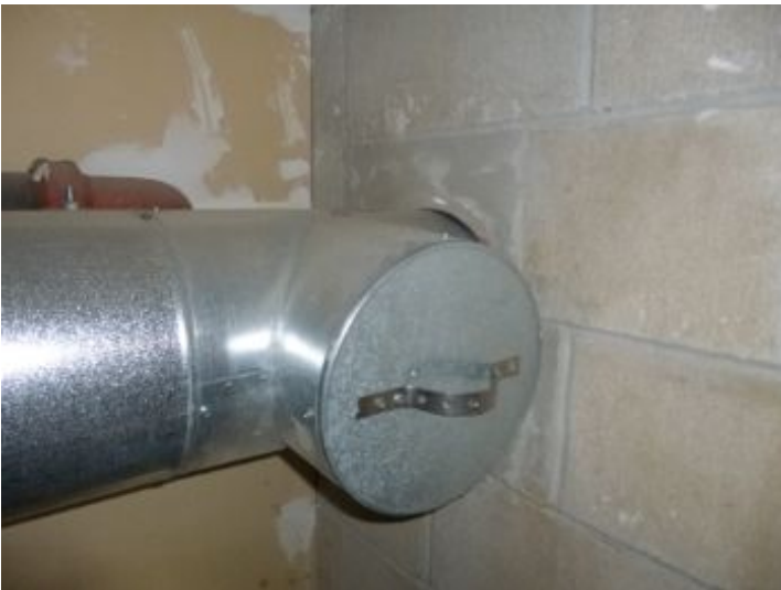
Boilers vent to chimney.
