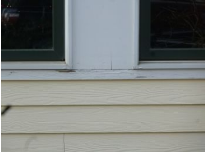
Peeling paint at front surfaces.
