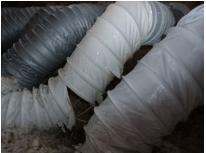
Damaged bath fan vent, nesting in vent, at maid closet attic area.
