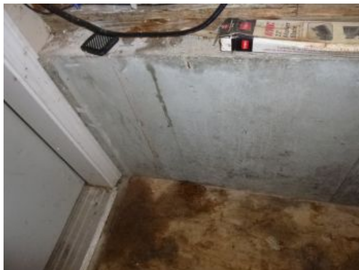
Water on wall at rear basement door.
