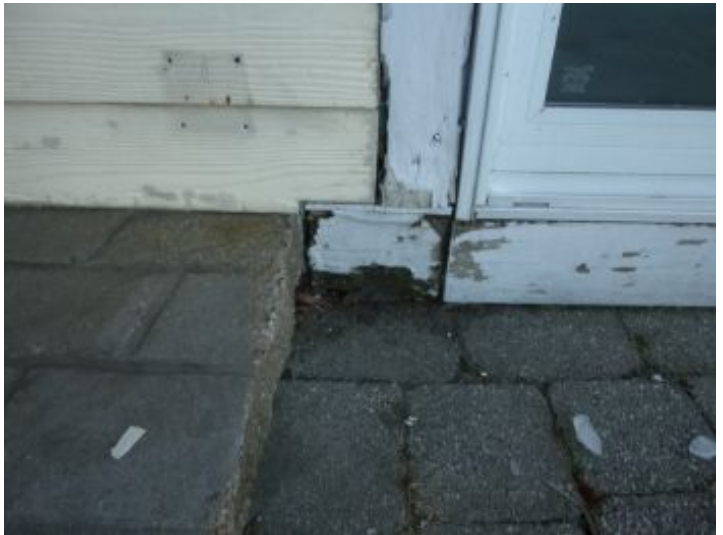
Damaged trim and siding at exterior wall of pool room.
