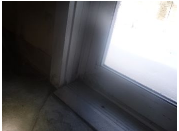
High moisture, dark staining , deterioration to wall surface in pool room.
