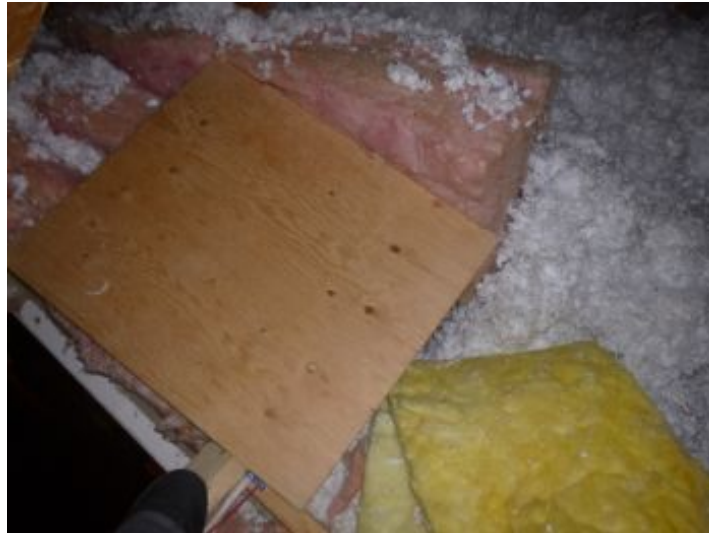
Scuttle covers should be insulated.
