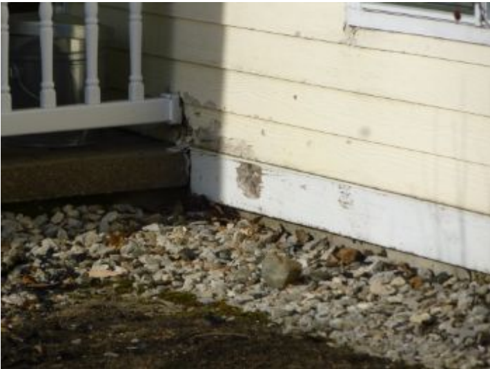
Deterioration to composite board siding at front building surface.
