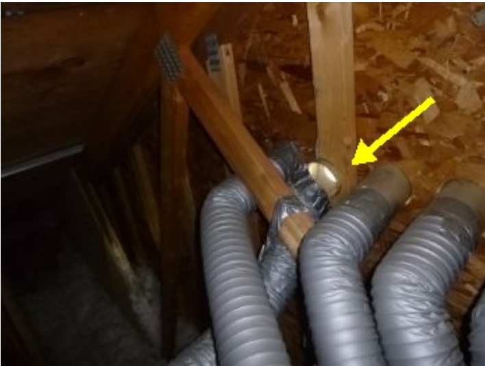
Damaged bath fan termination at middle hall attic area.
