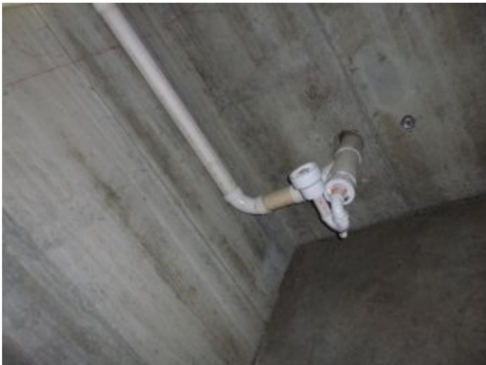
Main drain line to septic system.
