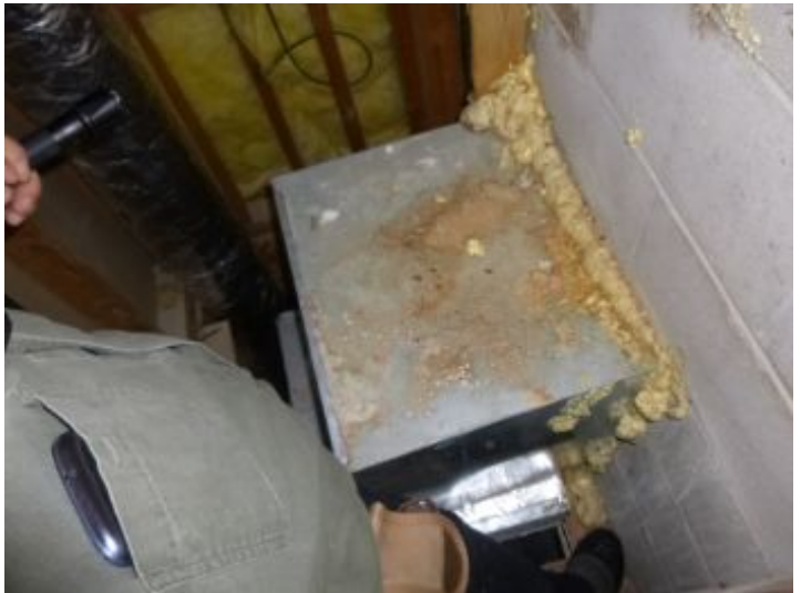
Mechanical chase for pool ventilation equipment, appears to be causing moisture into attic.
