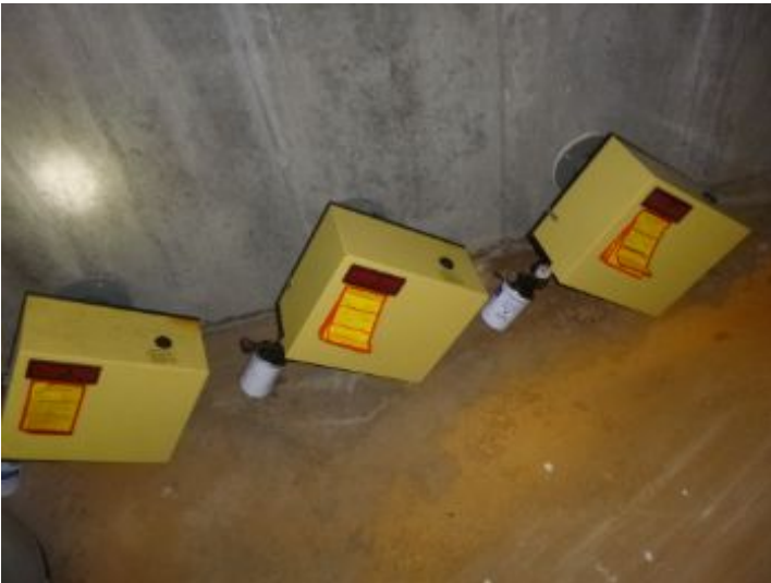
Burners to convert boilers to oil if warranted.
