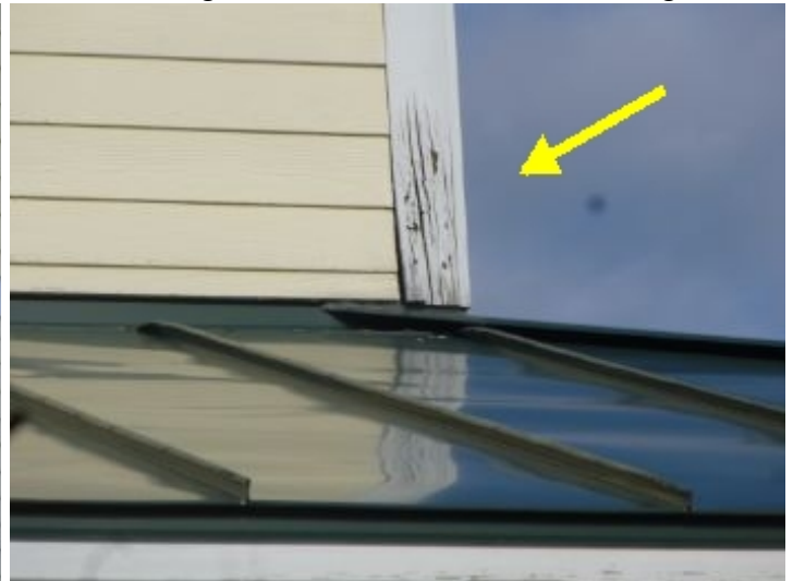
Damaged trim at left side surface.
