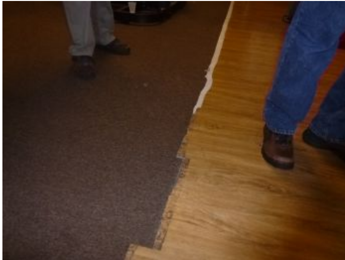
Laminate flooring in health club is loose, missing transition trim.
