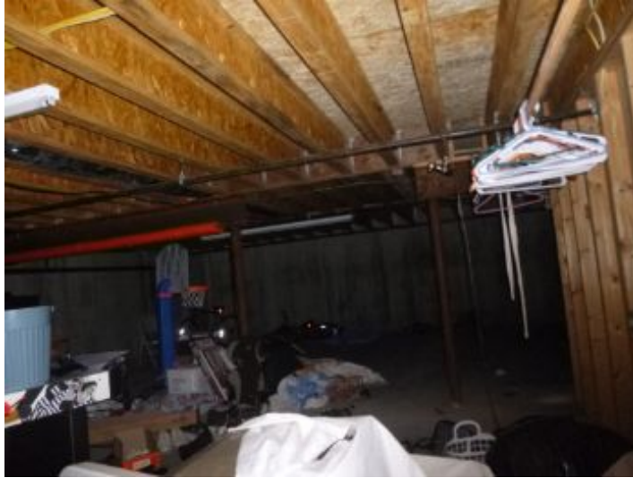
Framing, steel wood beams. engineered I beam joists.
