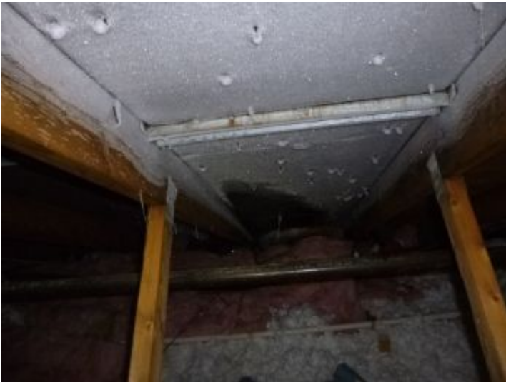
Frost , staining, wet surface at maid closet attic area
