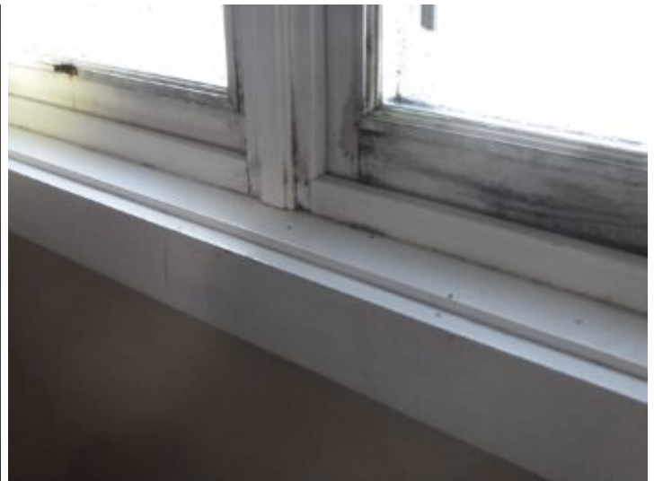
Condensation , staining on pool room windows.
