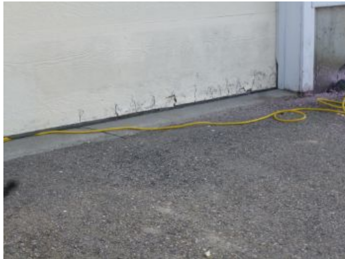
Deterioration to lower overhead door at rear of building.
