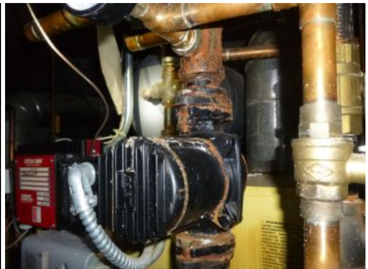
Some staining on boiler fittings.
