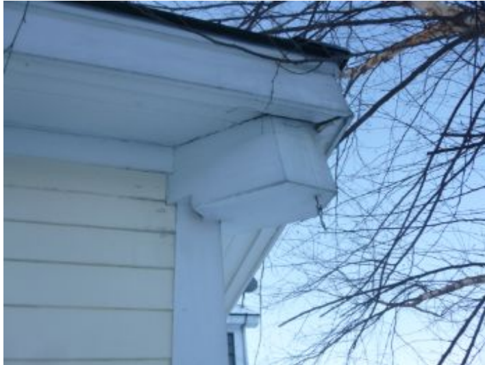
Trees in contact with rear surface of building.
