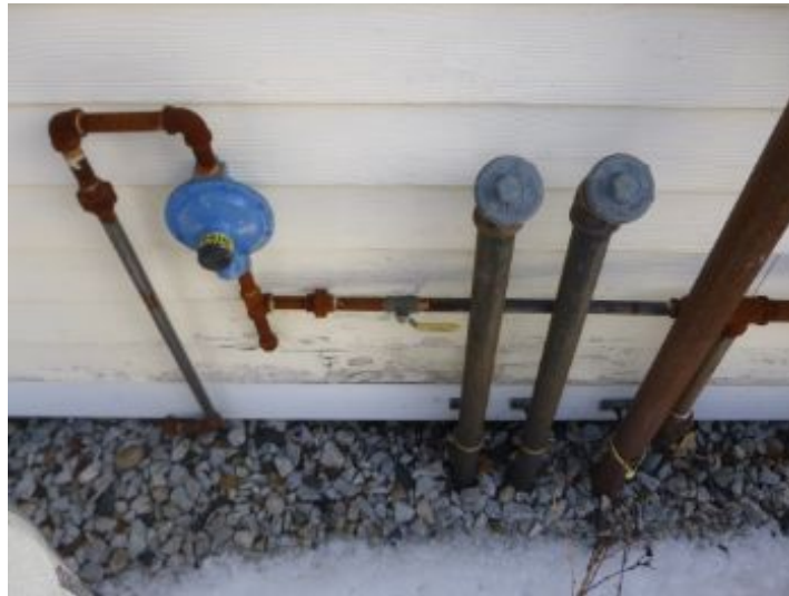
Propane gas piping entrance at rear of building.
