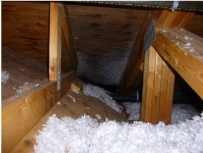
Frost , moisture staining on attic above owners quarter.
