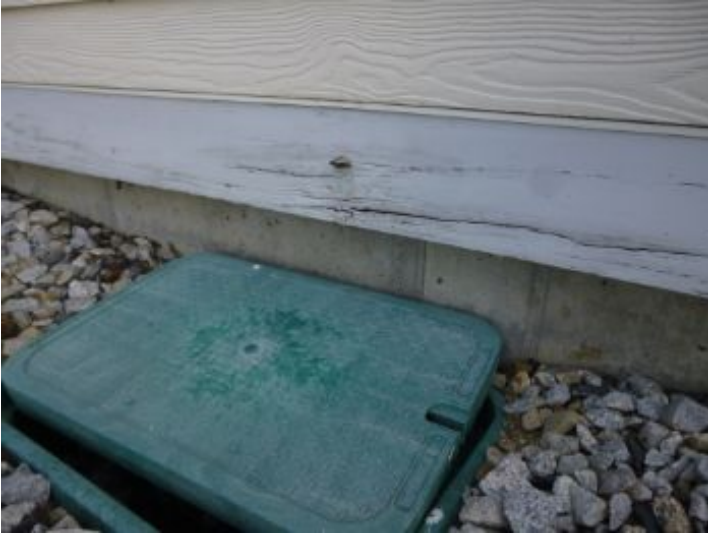
Damaged lower trim at rear building surface.
