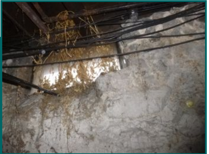
Vines growing into basement walls should be removed.
