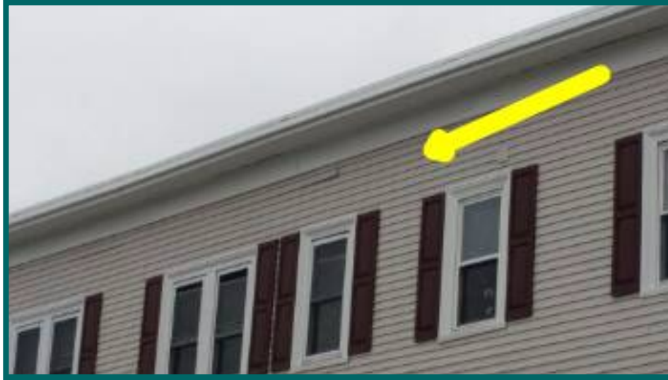
lifting siding at front wall surface
