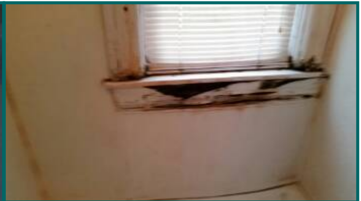
rot on window and wall unit 9 bathroom, requires immediate attention.
