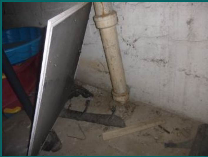
There are three drain line terminations in basement.
