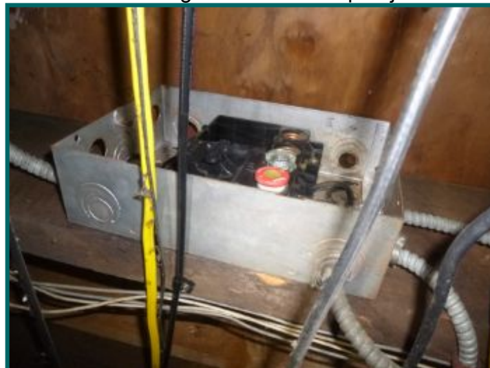
Screw in fuse sub panel, missing cover.
