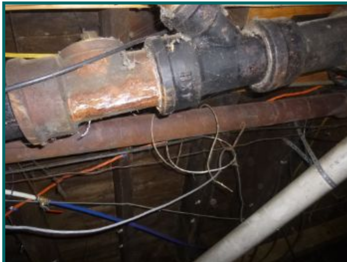
Corrosion on drain lines.
