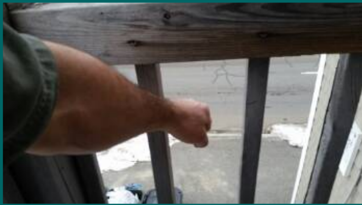
rail openings exceed four inches
