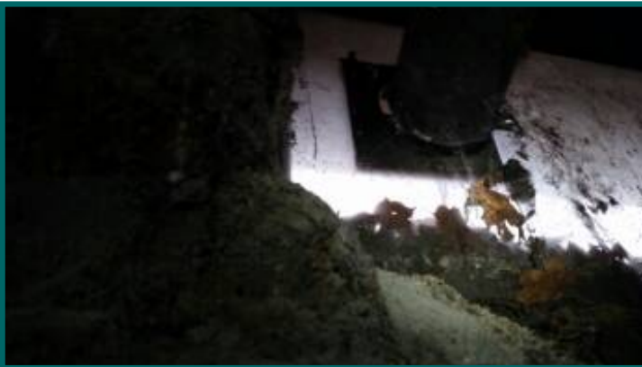
Front basement window dryer vent termination needs to be covered to prevent entrance of vermin.
