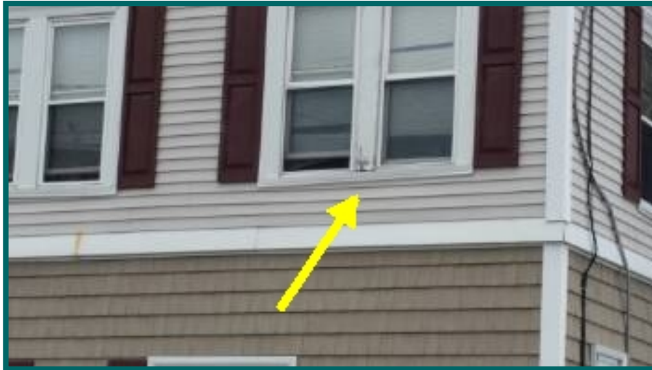
Frame rot at front window
