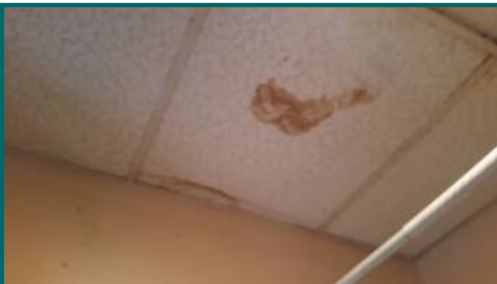
water staining tested drive unit 4 bathroom
