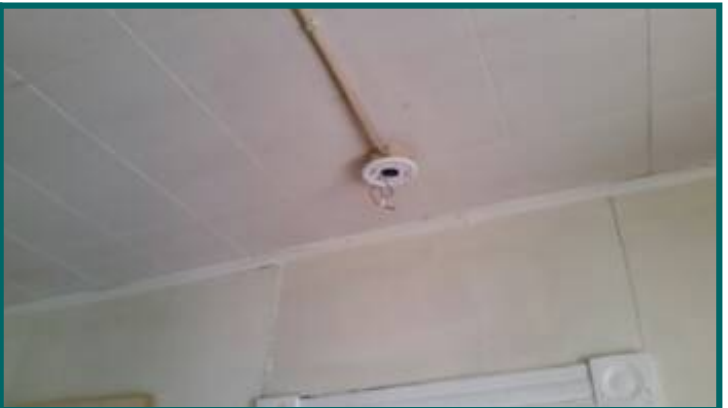
unit 11 smoke detector missing
