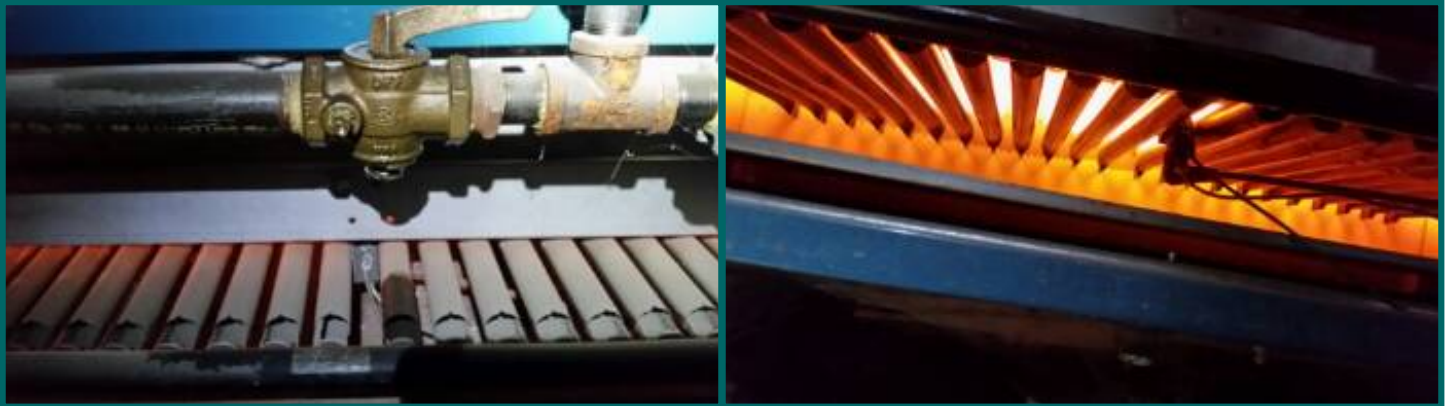
leak at gas shutoff valve inside boiler cabinet
