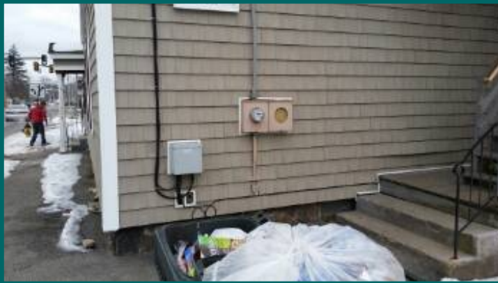
building is has one electric meter
