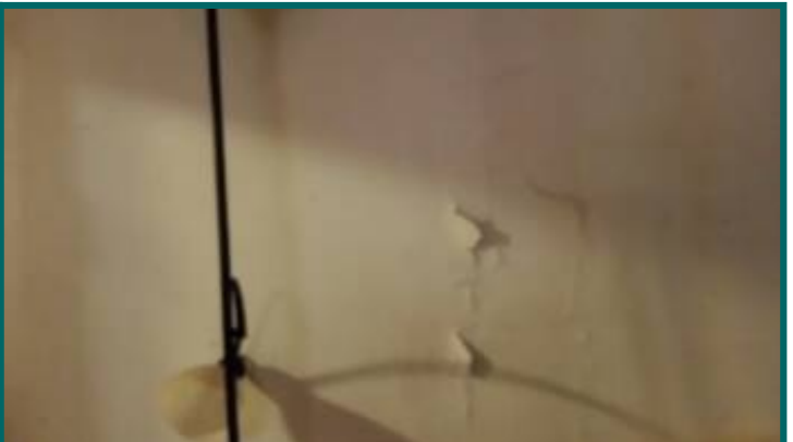
peeling paint damage unit 2
