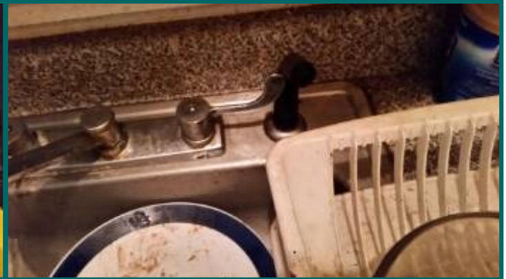
deterioration to faucet fixture damage spray wand unit 9
