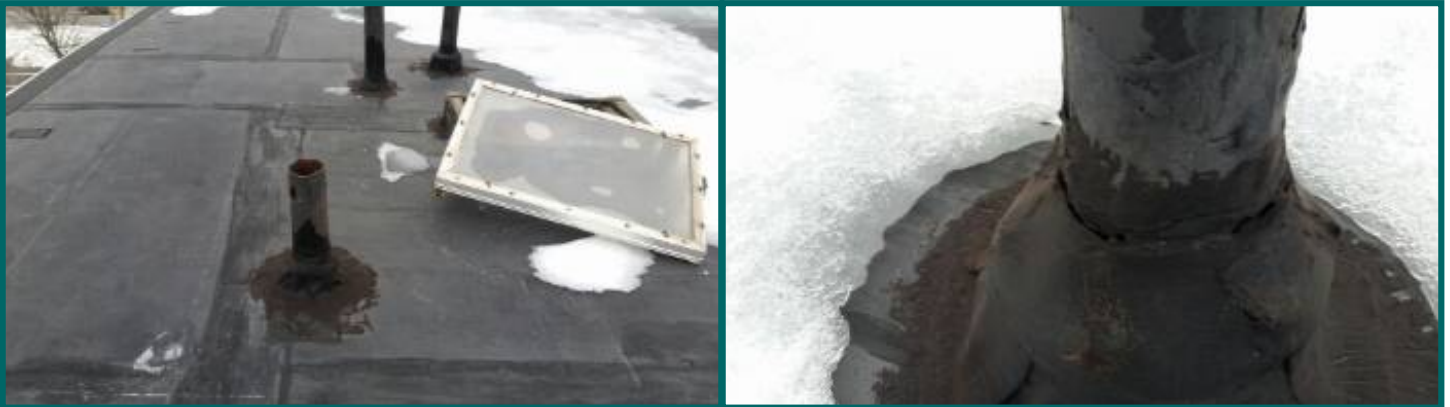
cracking in vent stack flashing needs to be resealed
