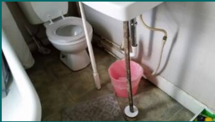
unit 7 bathroom sink leaking damage support post
