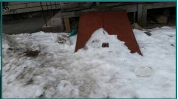
Bulk heads are commonly areas of water intrusion need to be monitored and sealed or repaired from time to time.
