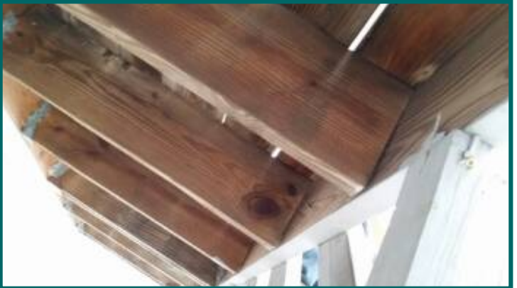
Missing Joist hangers.
