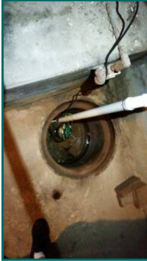
sump pump in boiler room
