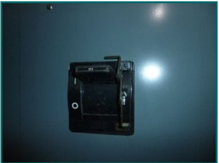
Main breaker disconnect 600 amp three phase.
