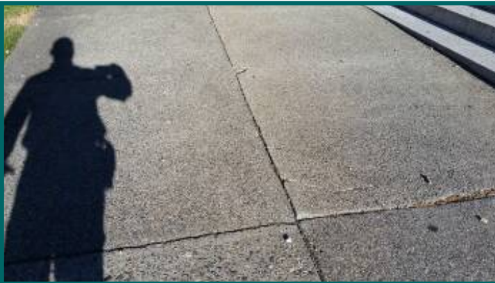
cracks and settlement in concrete surfaces front of building
