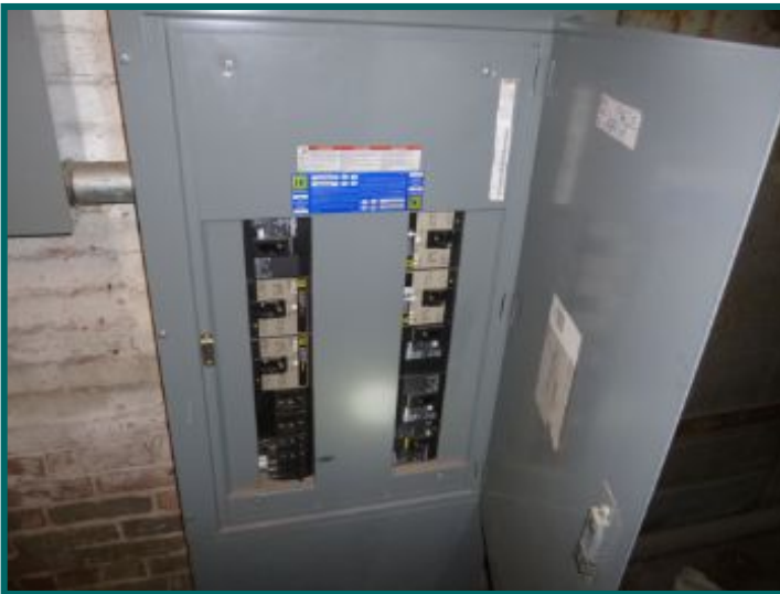
Numerous electric panels through out building , reported to be 10 years old.
