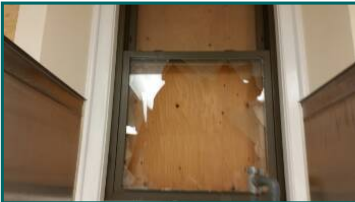
Broken basement window
