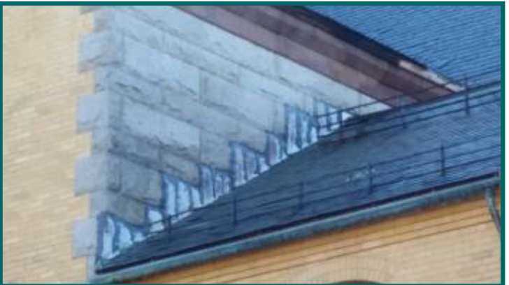
tar covered flashings will need to be monitored and serviced from time to time
