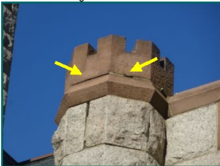
damage brick rear surface
