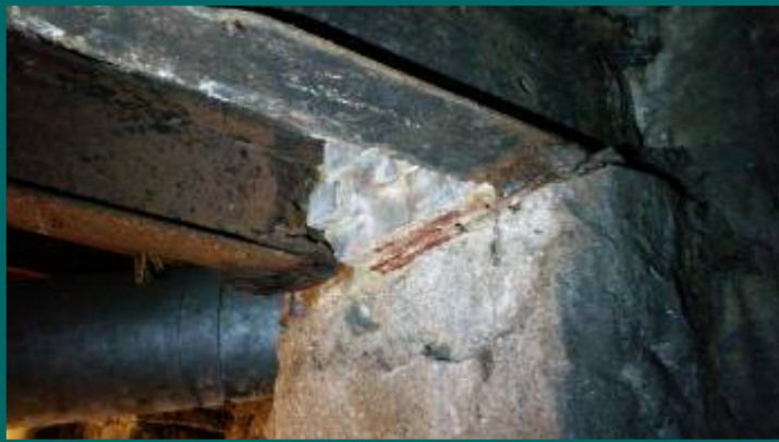
Corrosion on steel beams at bulkhead area
