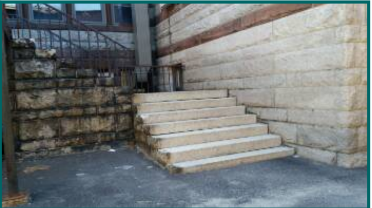
missing handrail side of building
