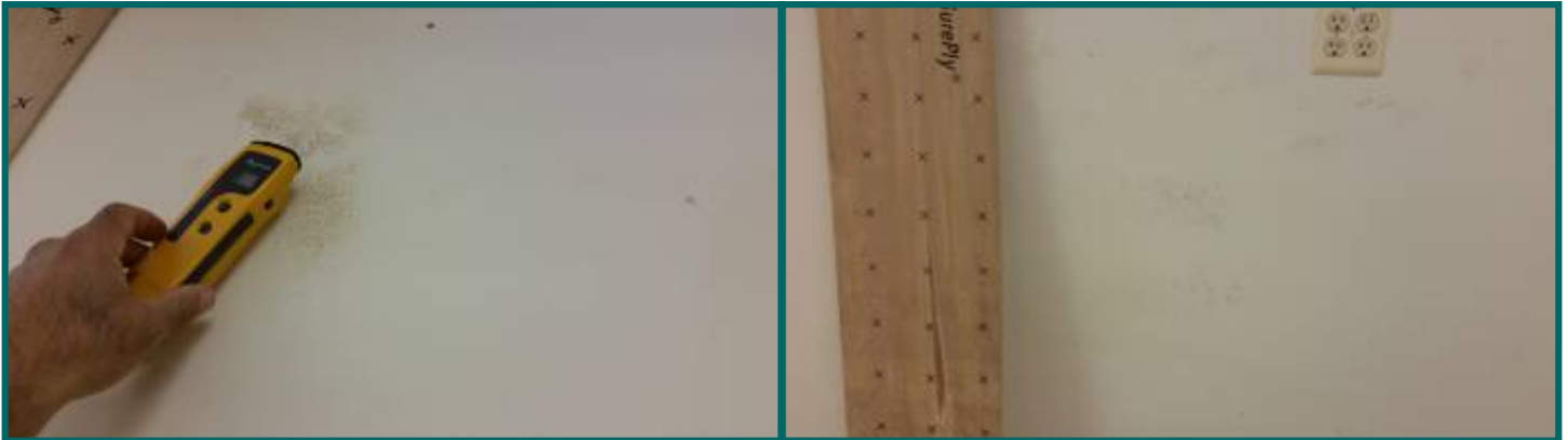
Front basement walls stains elevated moisture
