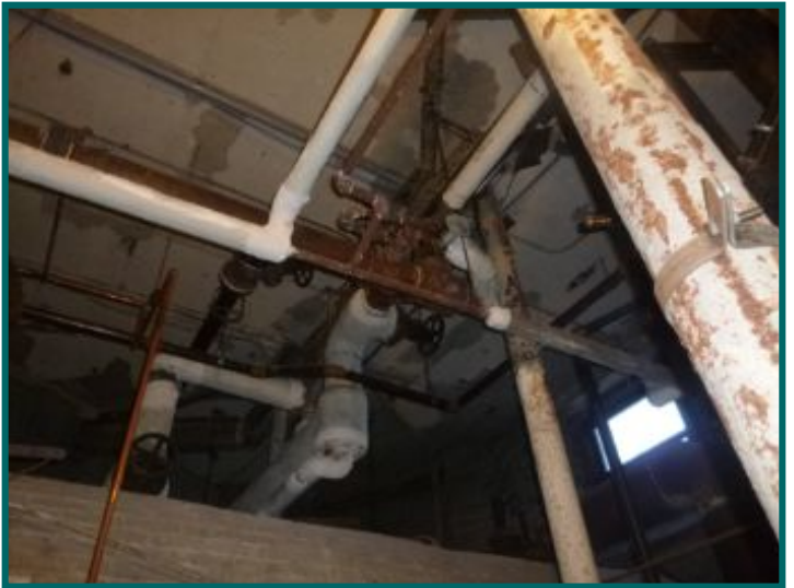
Suspected asbestos insulation.
