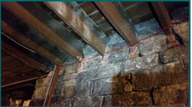
ceiling stains near bulkhead
