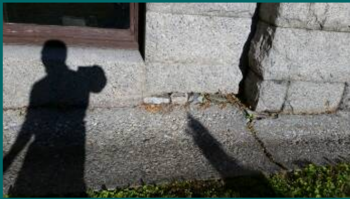
damage surface front of building this area appears to be letting rain run off into the building .
