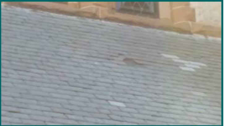
missing shingles front roof surface
