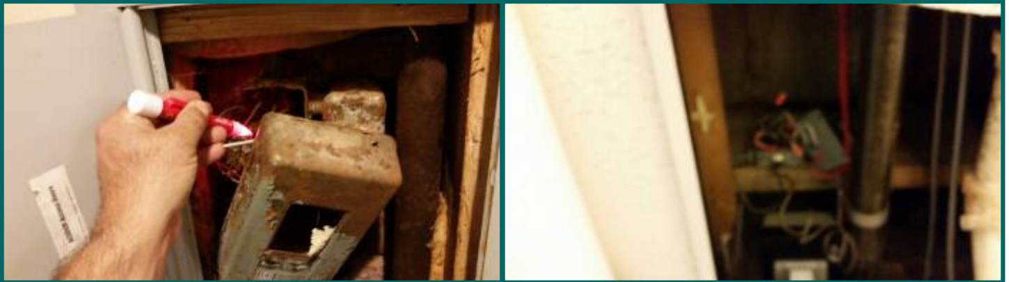
Rust damaged electric box in basement.
