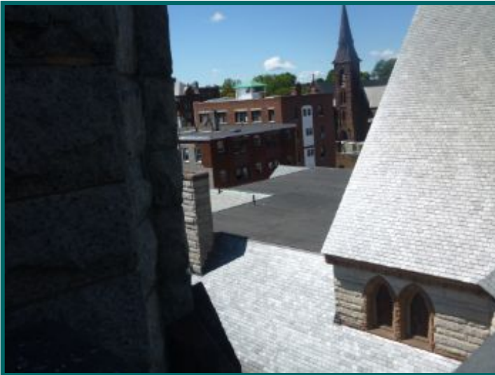
Flat rubber roof at rear of building.
