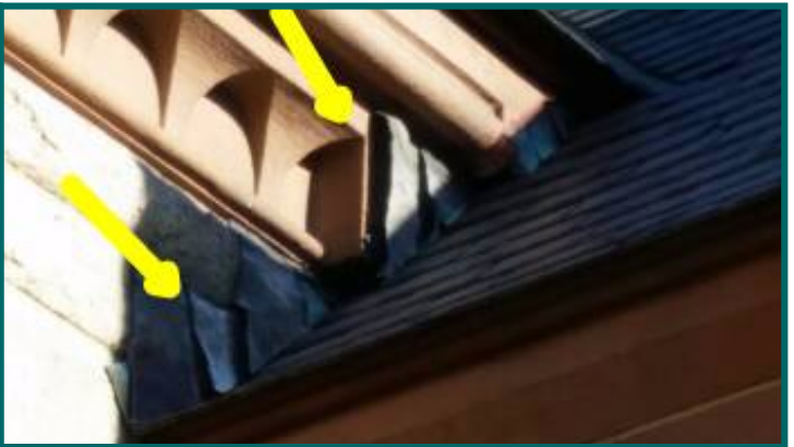
damaged flashing front of building
