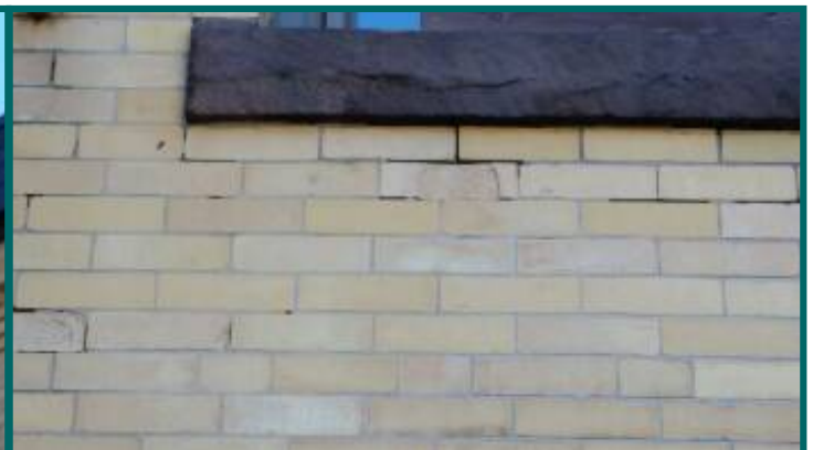
deteriorated grout rear brake surface
