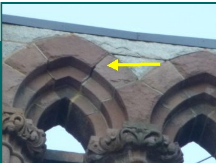
Gap in grout line front tower.
