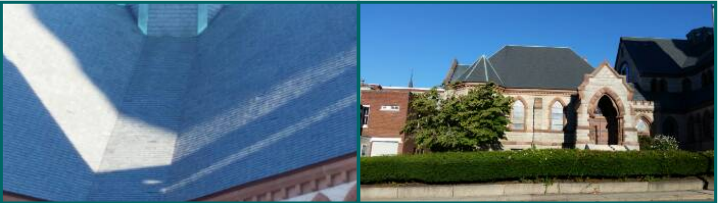
areas of missing and damaged shingles on main roof front roof surface
