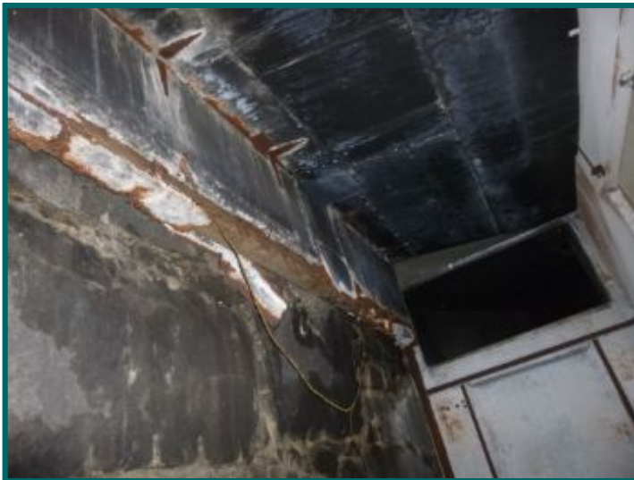
Staining on basement duct work.
