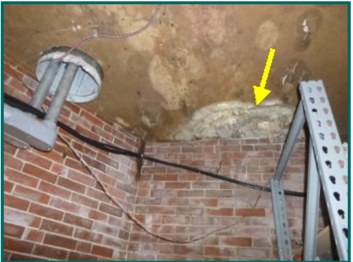
Suspected leaks at perimeter wall ceiling areas, suspected mold .
