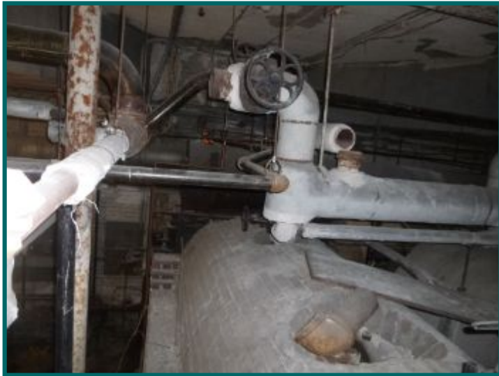
Suspected asbestos insulation.
