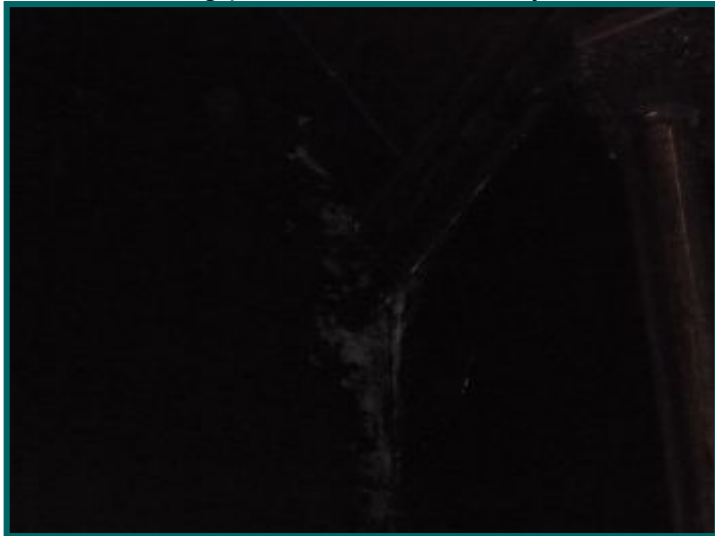
Efflorescence at wall ceiling transition. Evidence of water intrusion.
