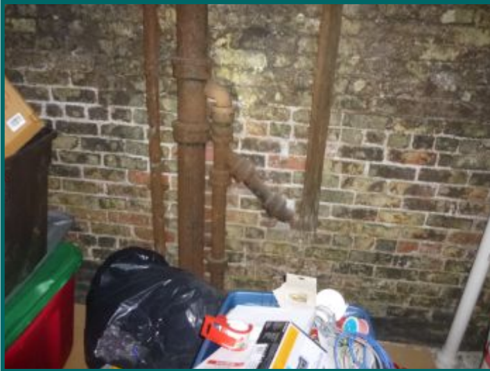
Corrosion on plumbing lines.
