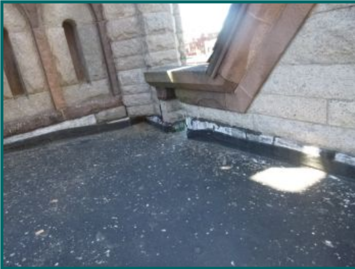
Rubber roof between two front towers.
