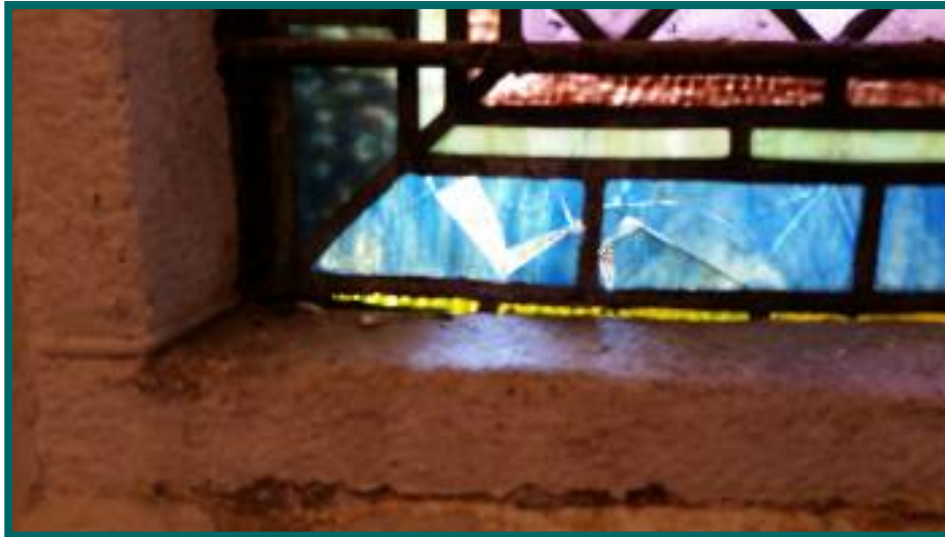
broken glass front foyer stained window
