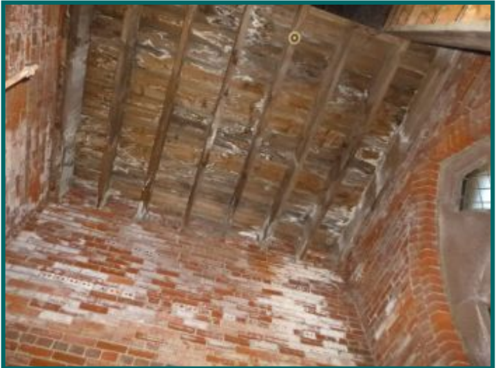
Staining on ceiling at right side tower.
