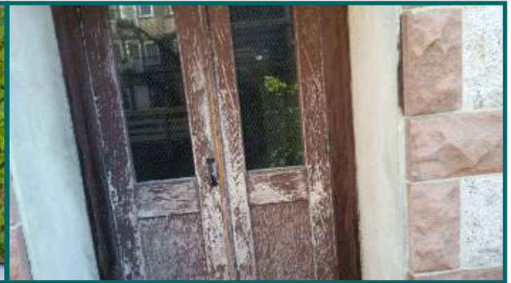
peeling paint at side door
