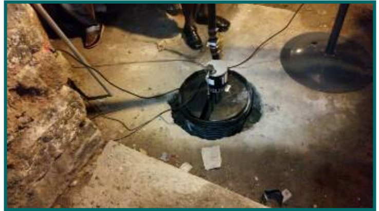
sump pump at bulkhead
