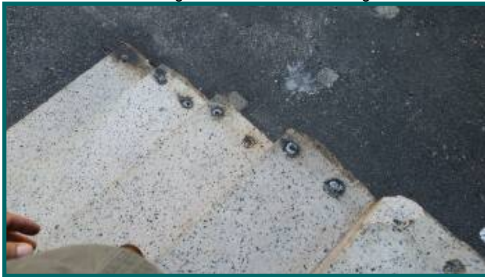
broken missing handrail
