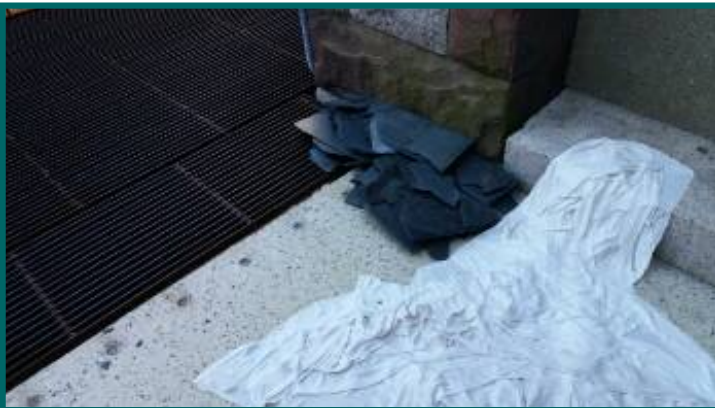
fallen shingles around building
