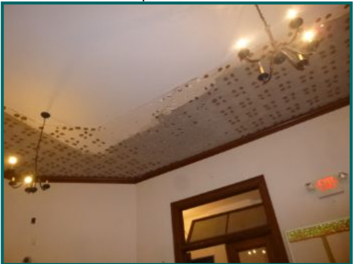
Damaged missing ceiling tiles.
