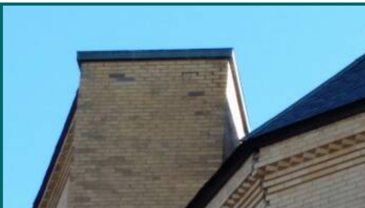
deteriorated grout rear brick surface
