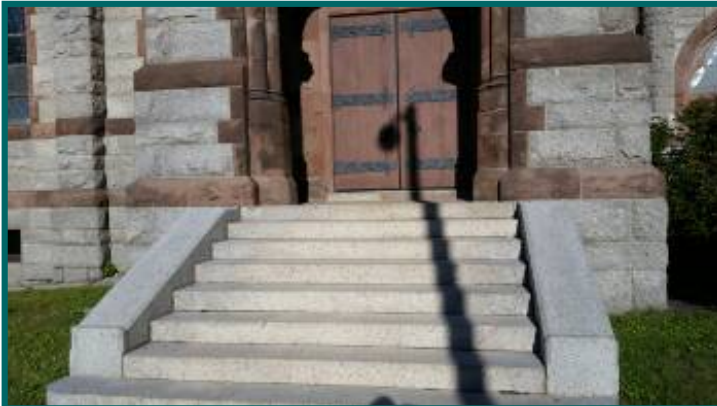
missing handrails front of building
