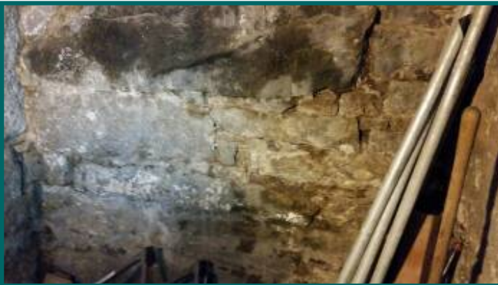
water staining near bulkhead
