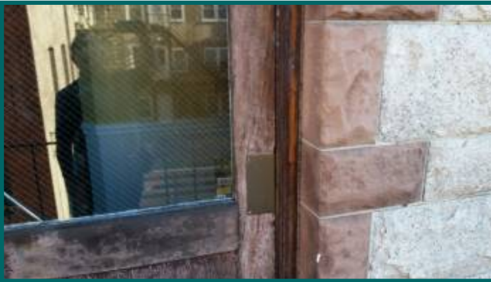
peeling paint at upper side door
