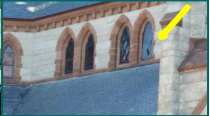
missing glass left side main church window
