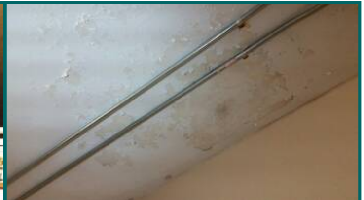
Peeling paint in basement.
