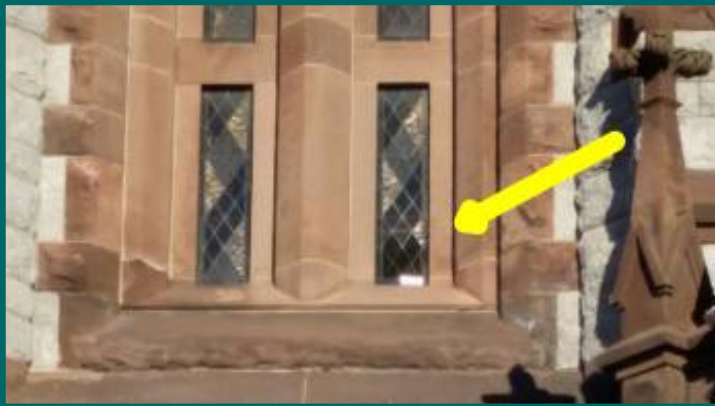
missing glass front left tower
