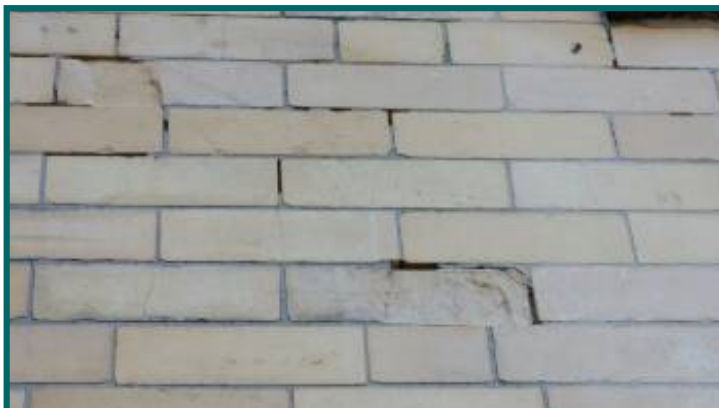
damage brick rear surface
