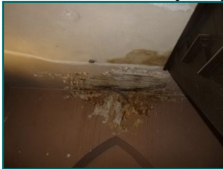
Staining at left side tower stairs, may be from pigeon activity, may be unsanitary.
