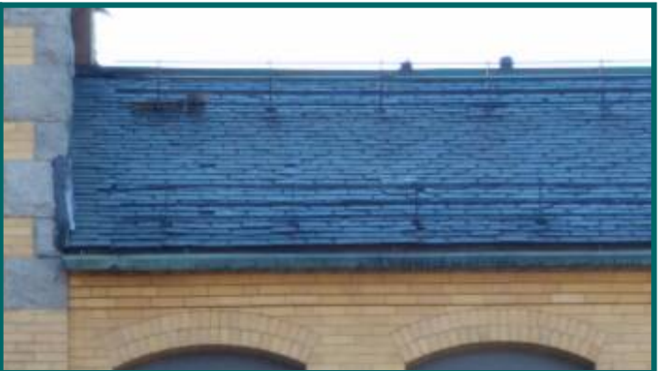
damaged missing shingles rear roof
