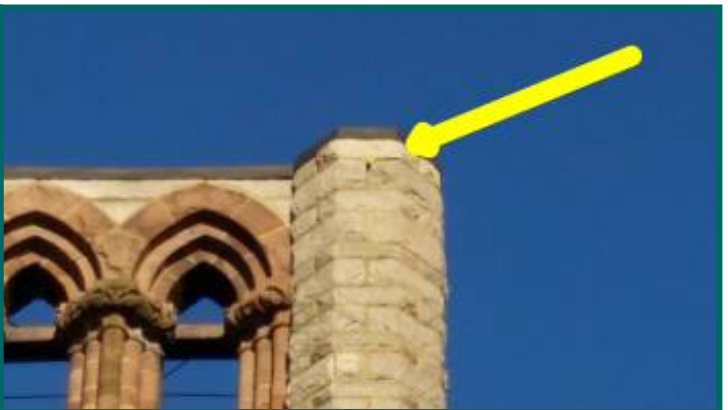
missing grout front left tower
