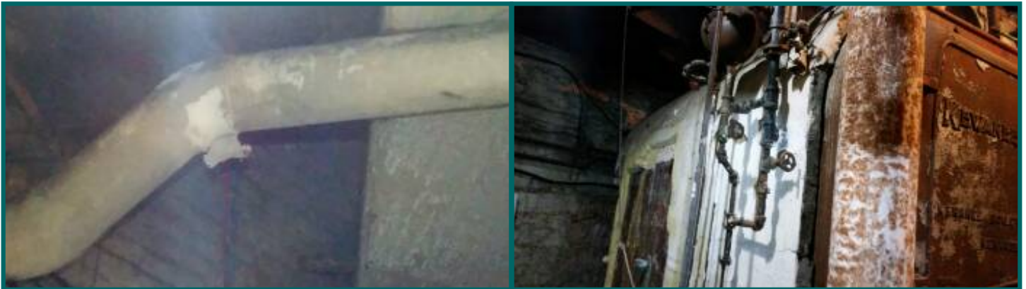
suspected asbestos
