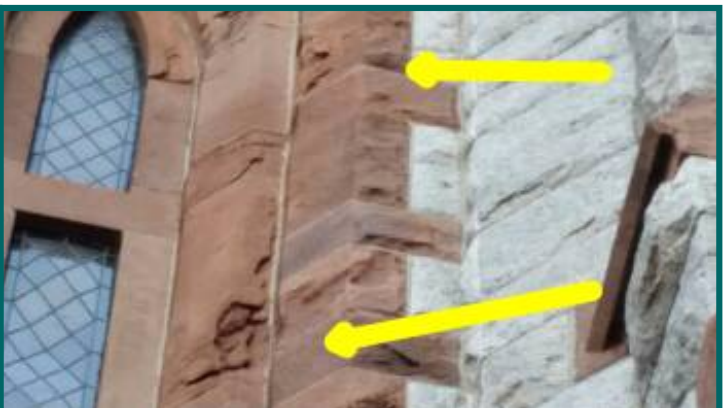
deterioration to stone work around windows at front right tower
