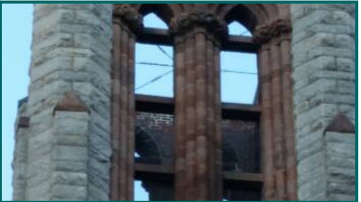
deteriorated grout right side tower front columns
