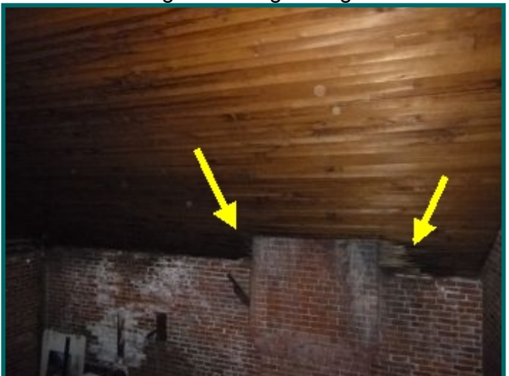
Staining around chimney transitions.
