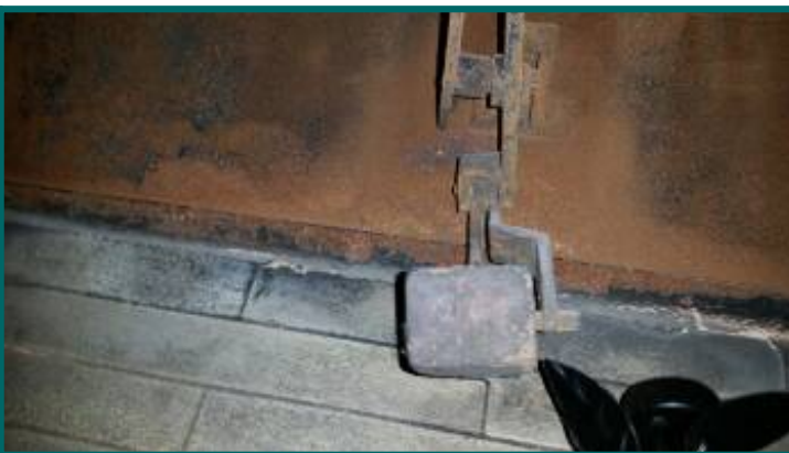
Damper damaged first floor fireplace
