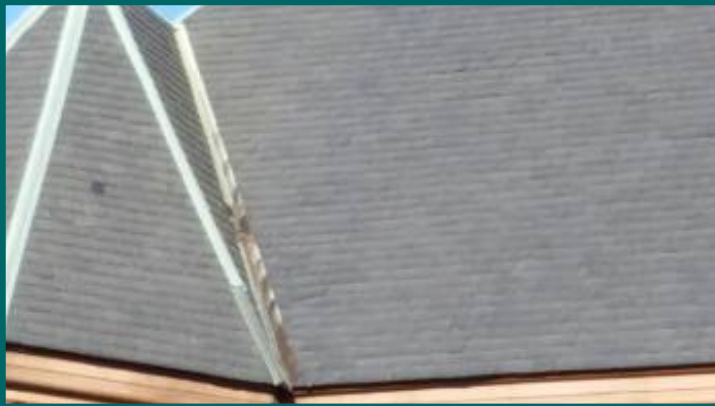
loose shingles front roof surface
