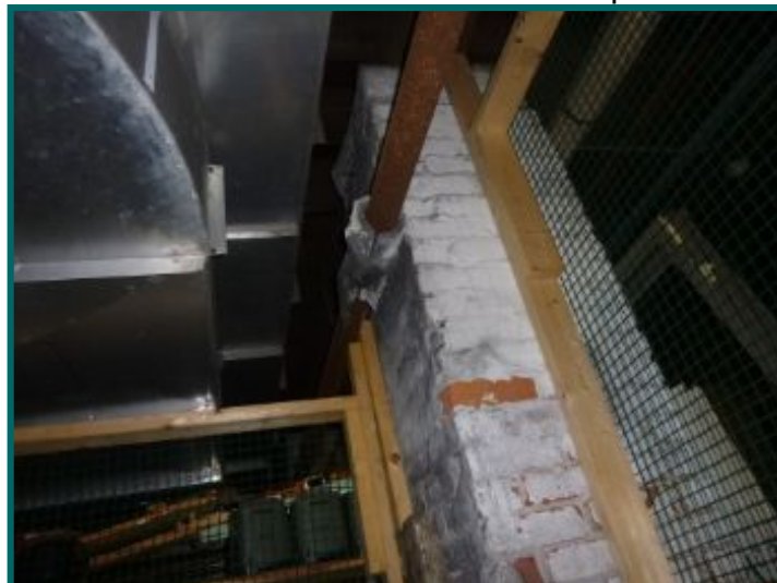
Suspected asbestos insulation.
