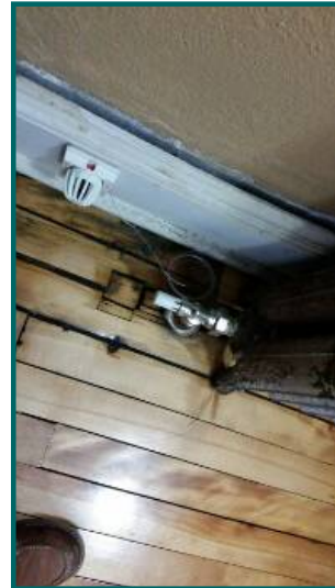
damage floor rear sanctuary office below heat register
