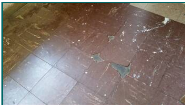
damaged 9 by 9 tiles left side hallway
