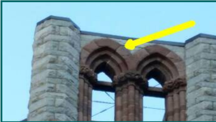
damage grout line right side tower arch
