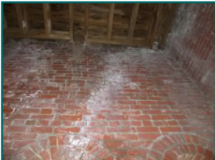
Efflorescence on right side tower walls, evidence of water intrusion.
