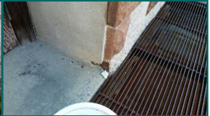
damaged wall surface left side of building at stairway
