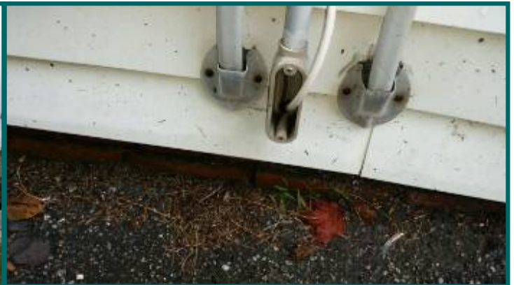
open conduit below meters
