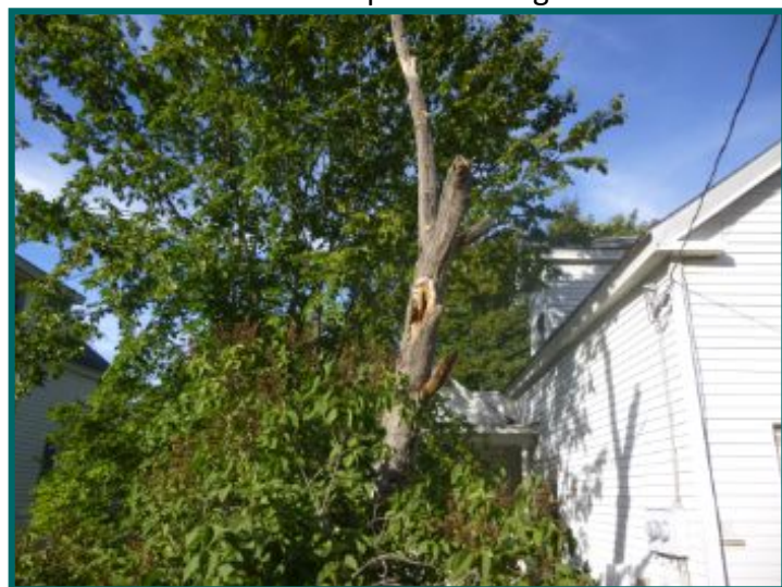
Trees overhanging roof should be cut back or removed.
