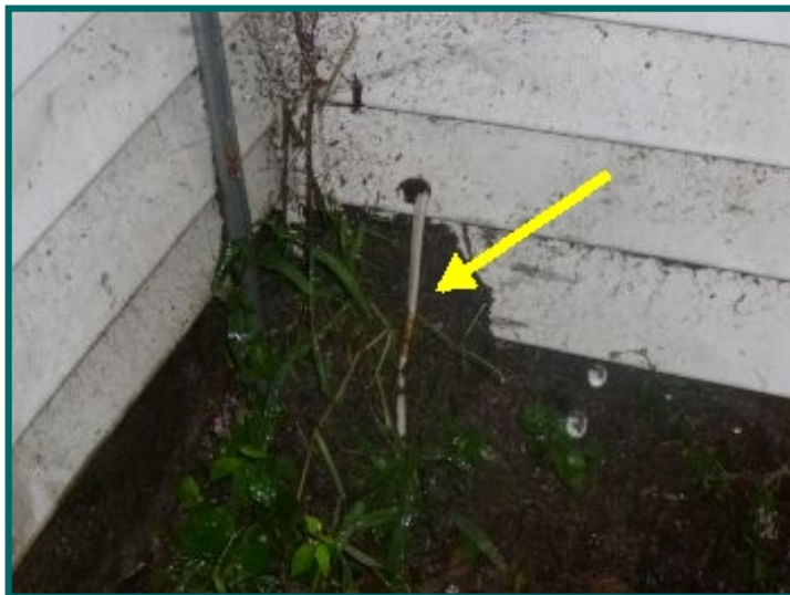
Exposed wires at rear of house
