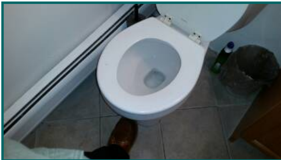
left side apartment toilet is loose
