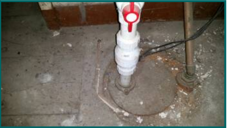
Expulsion pump for basement plumbing fixtures.
