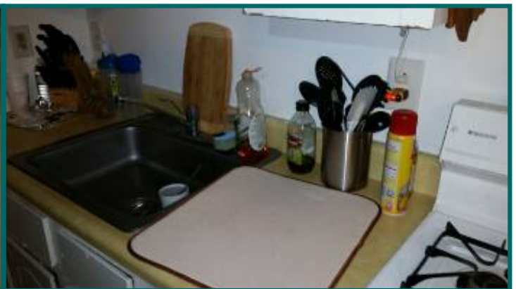
No GFI protection at kitchen outlets.
