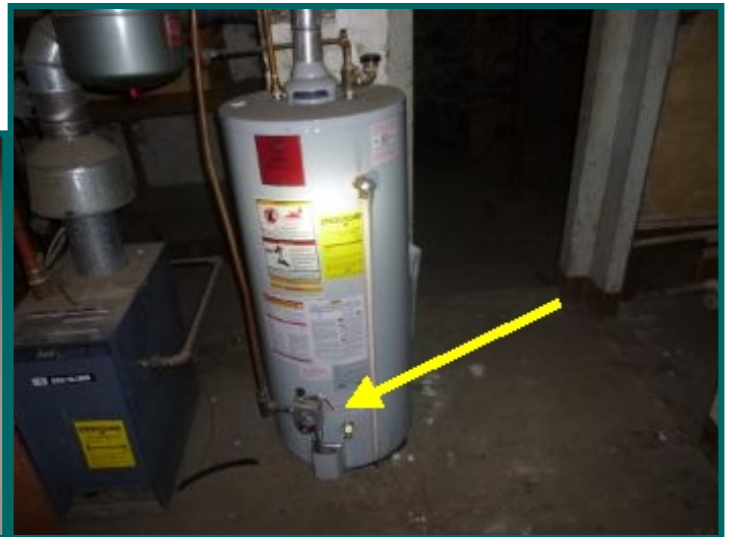
Mixing valve / burner control to adjust water temperature.
