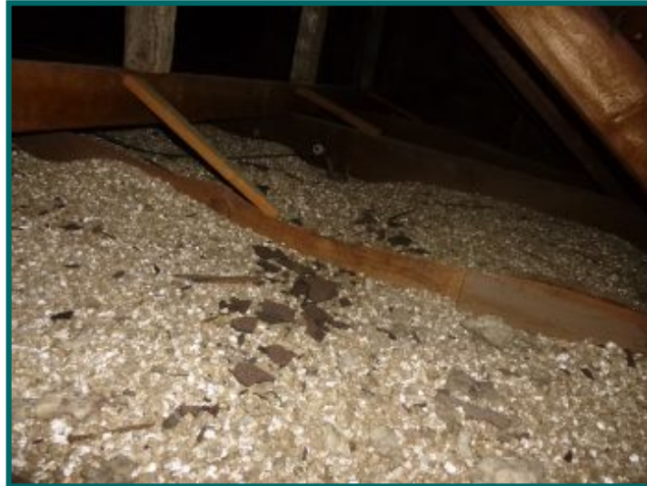
Vermiculite insulation
