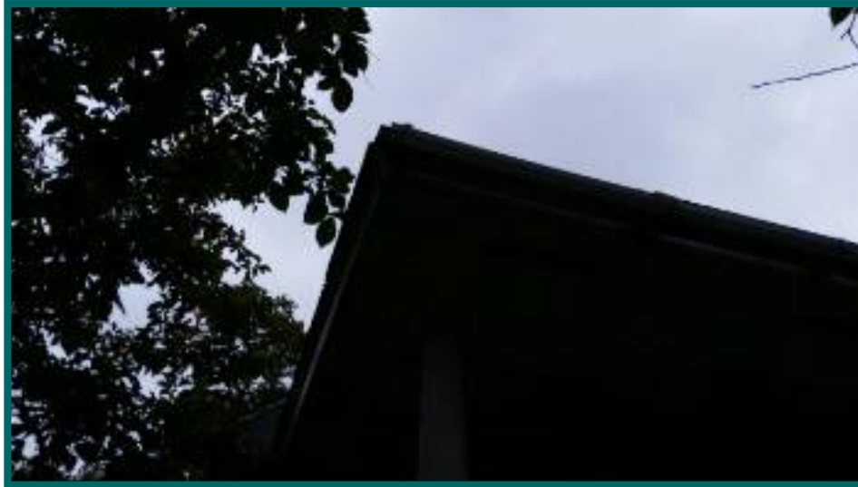
missing end cap & downspout at front porch
