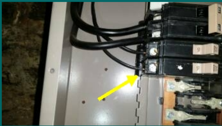
14 gage wire on 20 amp breaker left side apartment panel.
