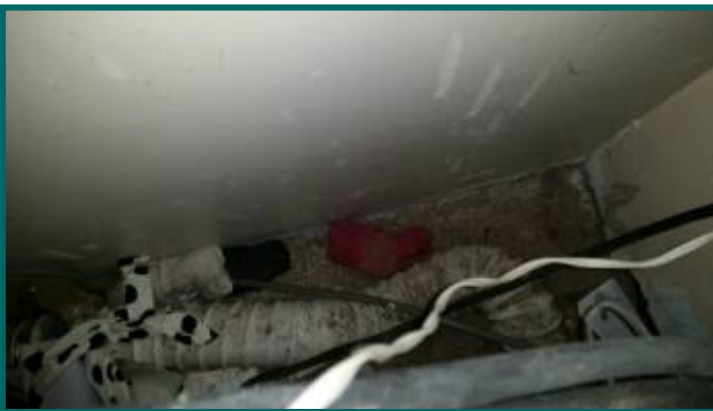
Accordion type dryer hose right side.
