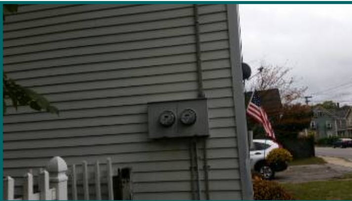
separate electric meters
