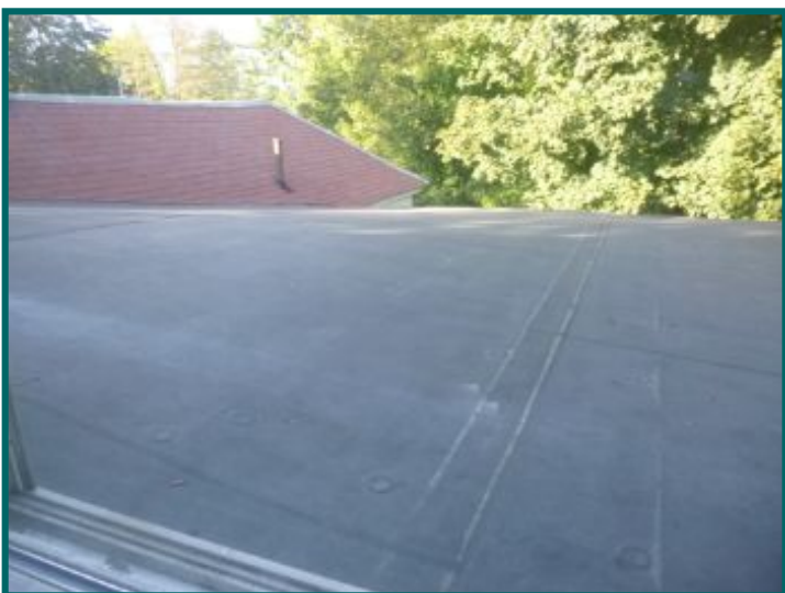
Rubber rolled roof
