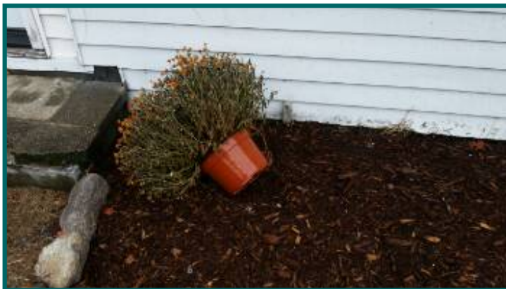
contact with finish grade front of house
