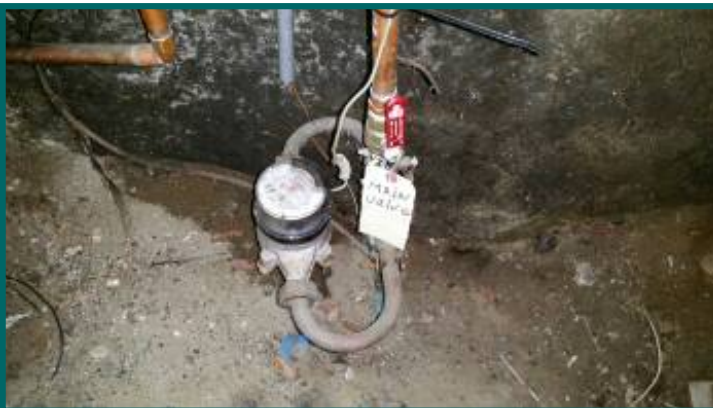
Main water shut off valve is located at water meter.
