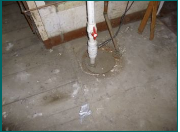
Expulsion pump for basement plumbing fixtures.
