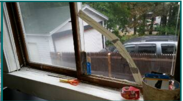
right side apartment family room window has broken glass will not open
