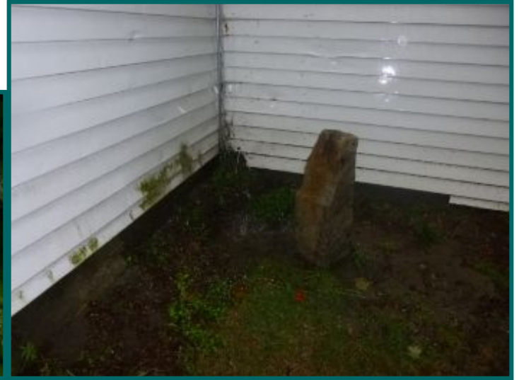
Rain water ponding at rear of house
