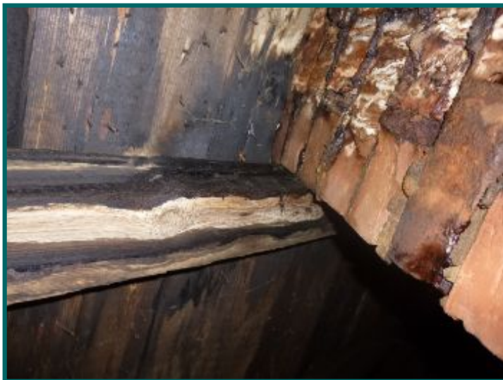
Leak around chimney.
