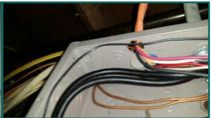
open knock outs, missing bushings
