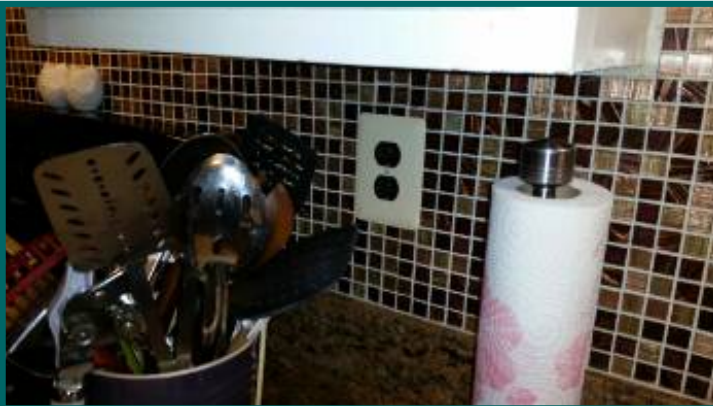
No GFI protection at kitchen outlets.
