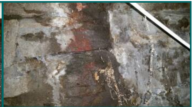
leak below side window
