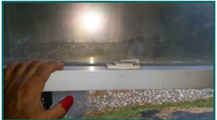
right side apartment dining room window is fogged will not lock.
