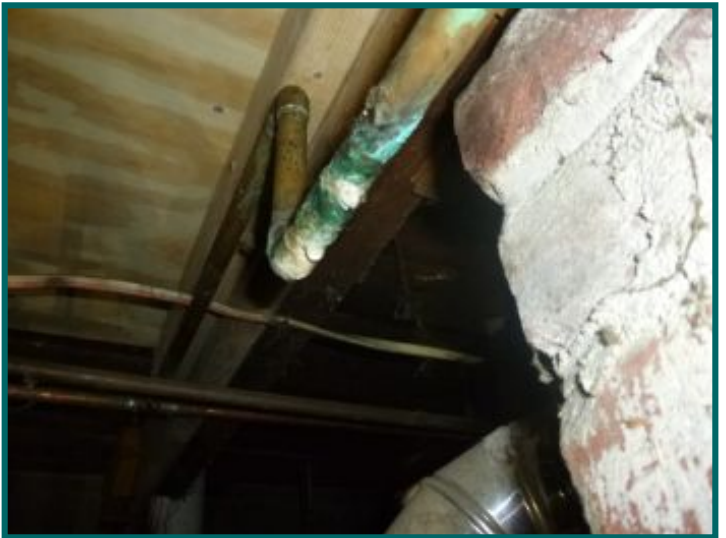
Leak on plumbing line in basement.
