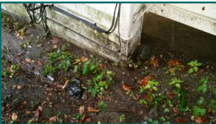
contact with finish grade side of house
