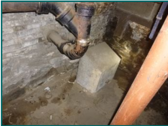
Main drain line termination.
