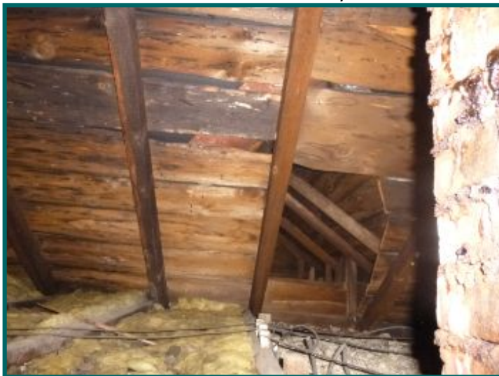
Leak around chimney.
