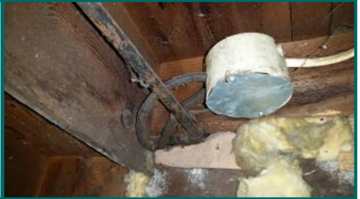
improperly secured junction box, wires in contact with pipes
