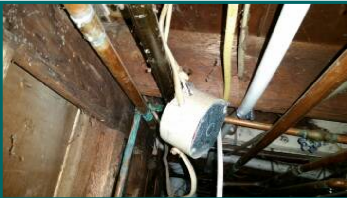
improperly secured junction box, wires in contact with pipes
