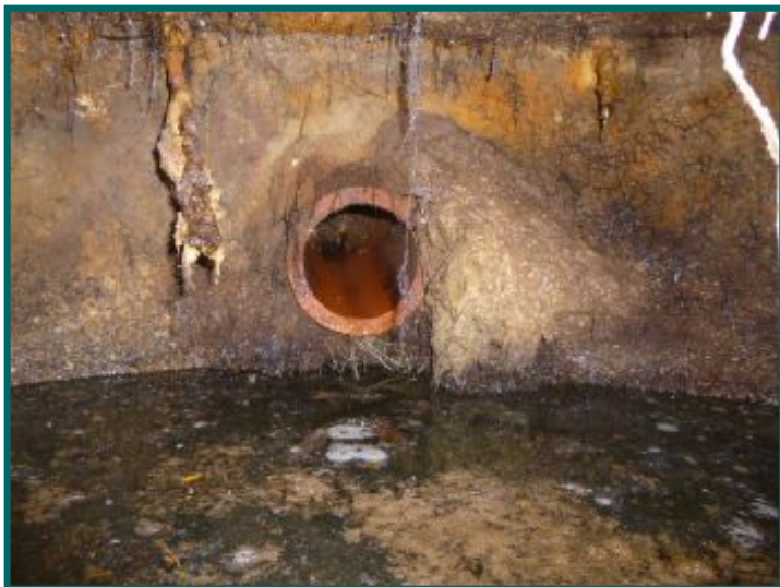
Inlet baffle missing
