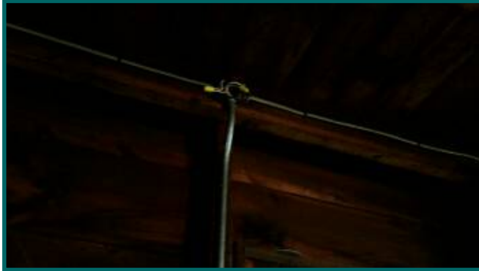
numerous open junction boxes in garage
