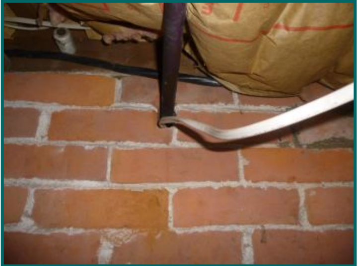
Wires in contact with plumbing lines
