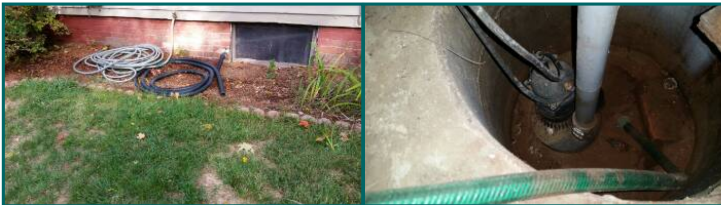
Sump pump drain line termination.
