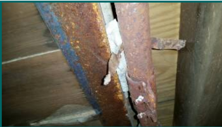
some remnants of old style suspected asbestos insulation on wrapped steam pipes
