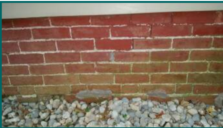
step cracking and repairs to brick on left side of house
