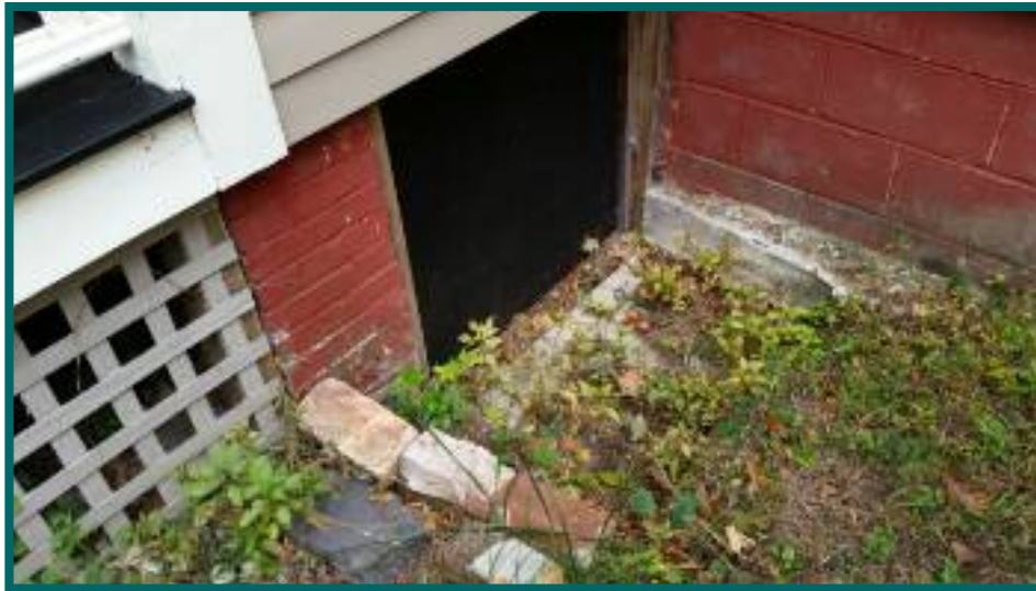
old bulkhead door well may be conducive to ponding and water intrusion
