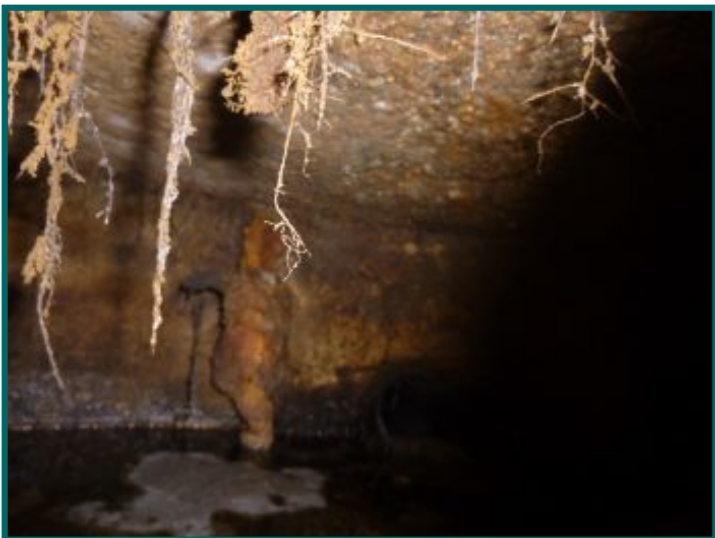
Outlet baffle missing
