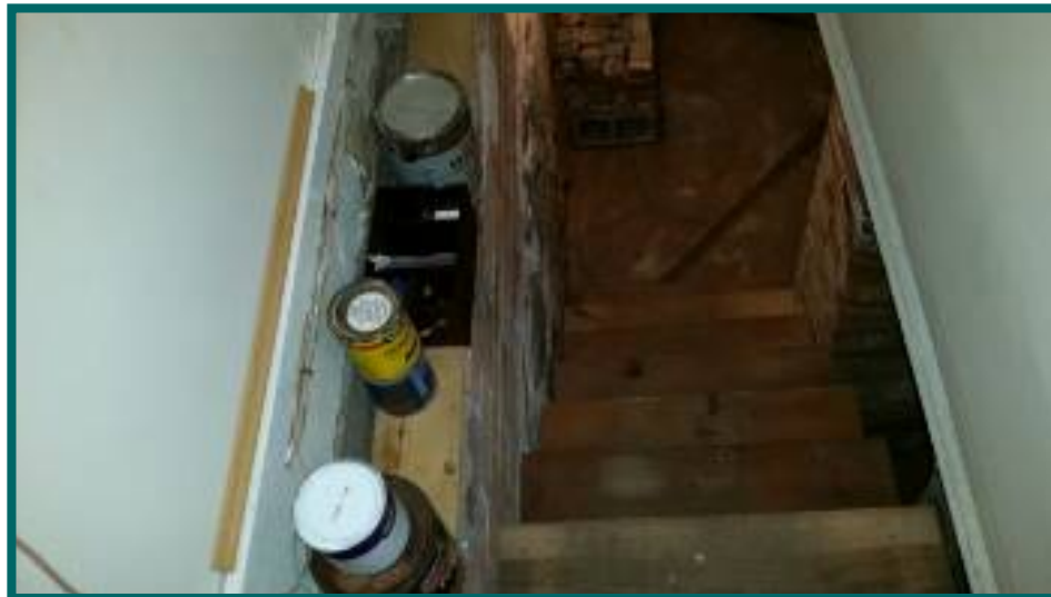
missing hand rail at basement stairs.
