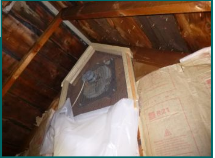
Thermostatically controlled fans are not operated.
