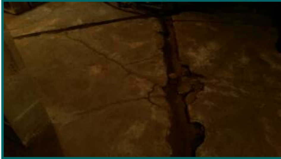
French drain and floor leading towards sump pump
