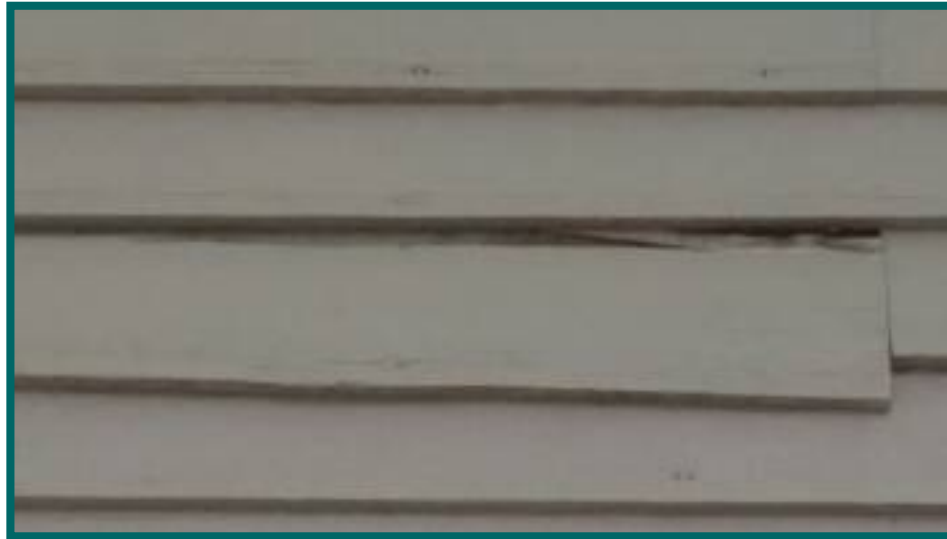
loose siding on rear barn wall
