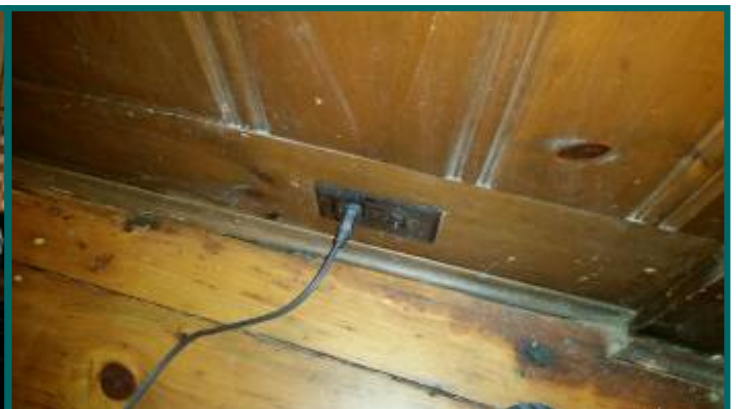
numerous ungrounded outlets on first floor
