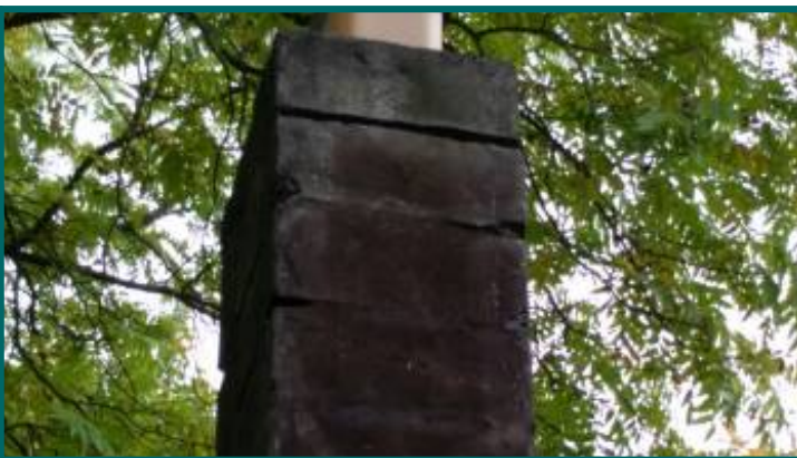
deterioration to mortar on rear chimney
