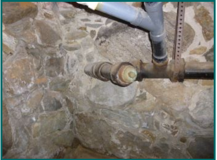
Secondary gray water drain line termination.
