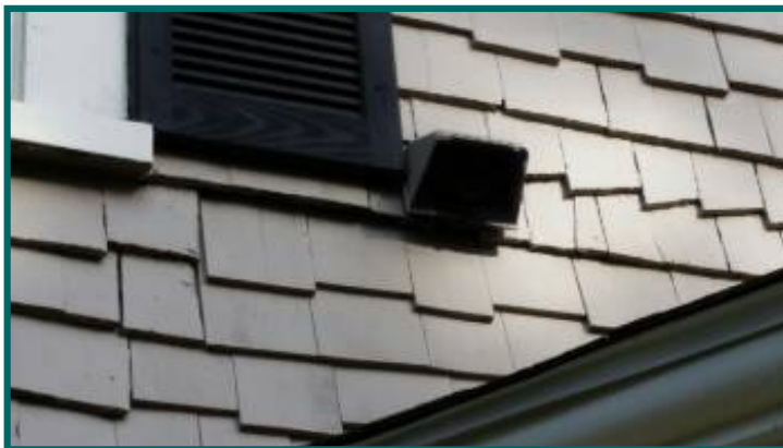
Dryer vent termination
