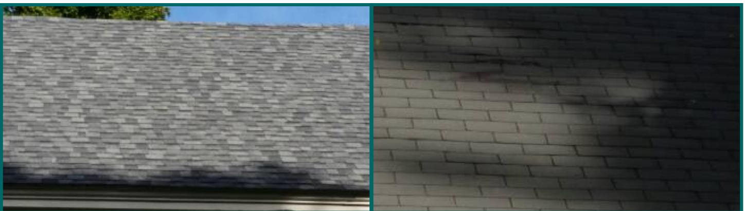
Garage roof is older, a few areas of damaged shingles over garage
