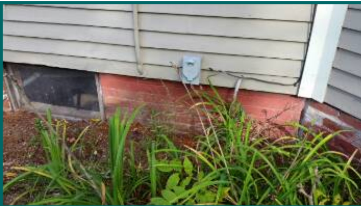
Generator transfer switch connection next to electric meter
