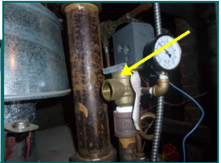
Missing down pipe for pressure relief valve
