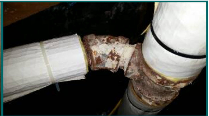
Remnants of older suspected asbestos insulation.
