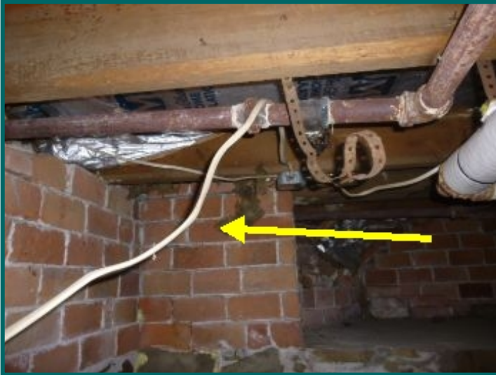
improperly secured wires in basement.
