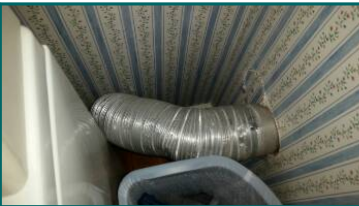
Semi rigid dryer vent hose is an approved material.
