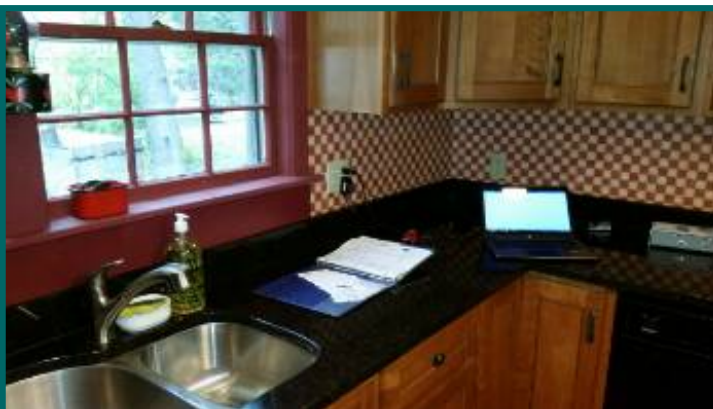
No GFI protection at kitchen outlets.
