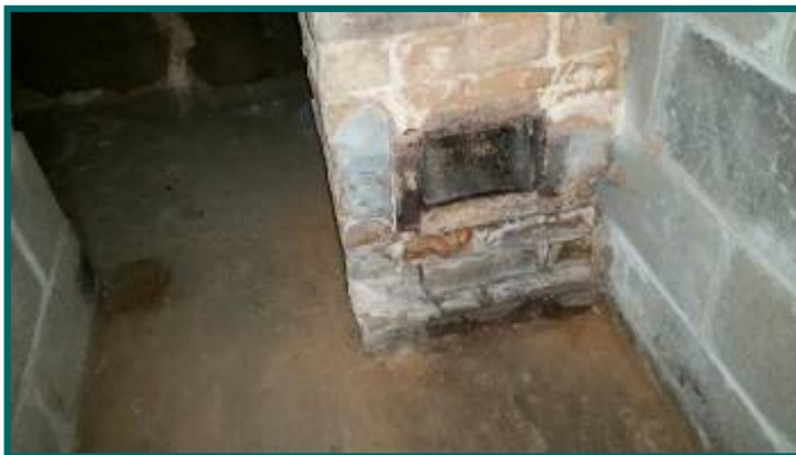
deterioration basement chimney surfaces.
