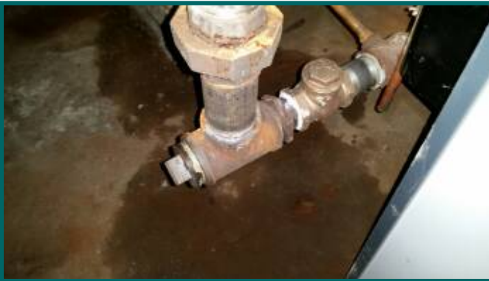
leak on fitting near boiler
