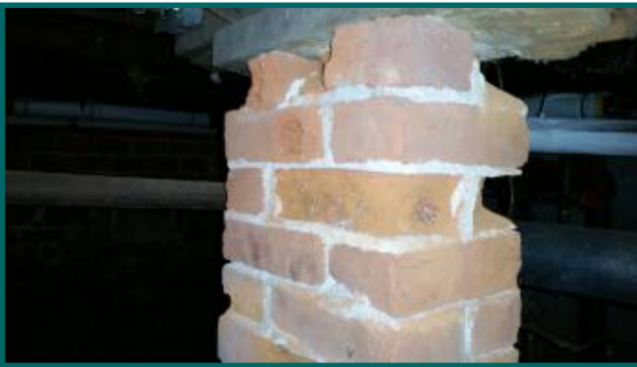
deterioration to brick support posts
