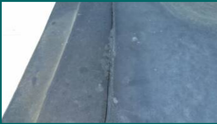
lifting seam
