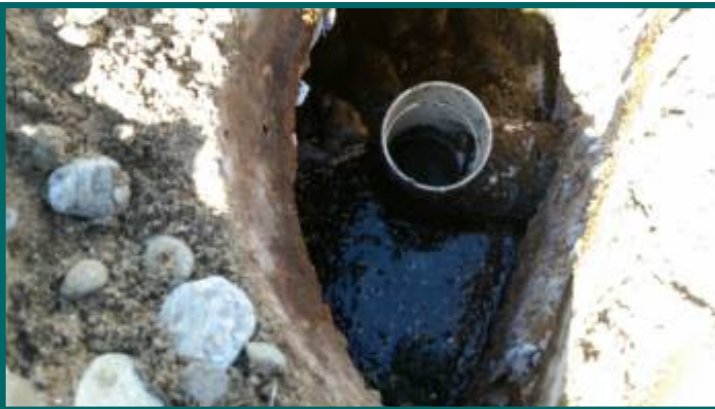
Septic tank outlet baffle.
