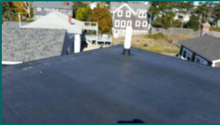
upper plumbing vent stack
