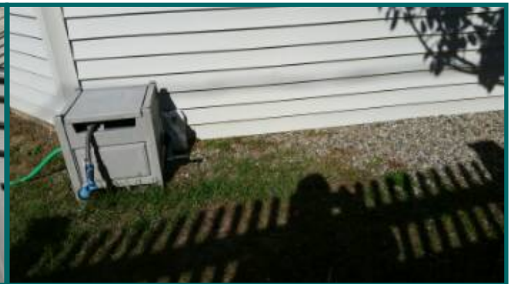
Siding in contact with finish grade.
