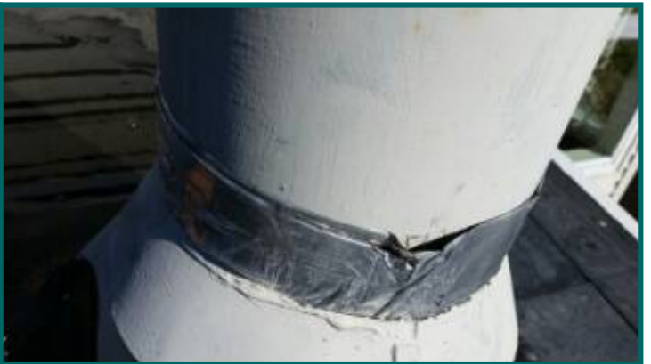
flashing tape is lifting on fireplace vent stack
