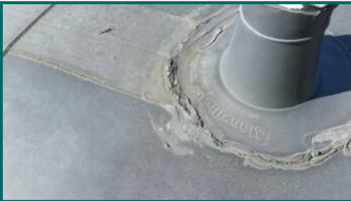
crack sealant on second roof vent stack
