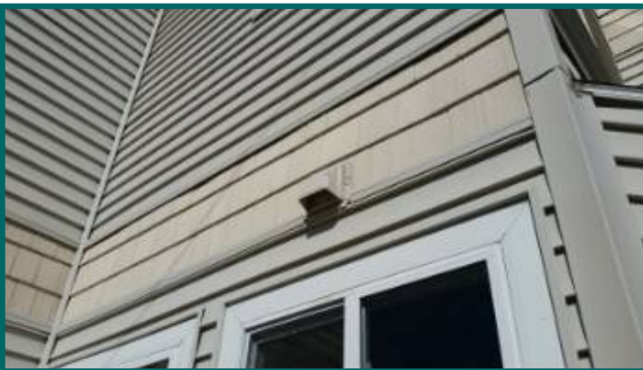
First floor bath fan termination.
