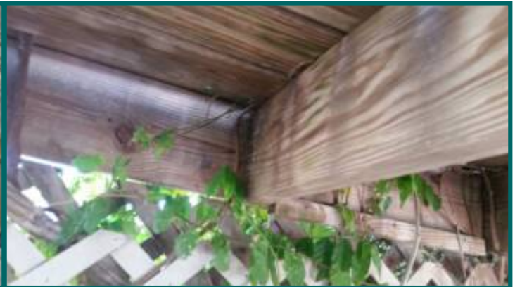
missing joist hangers at outside rim frame
