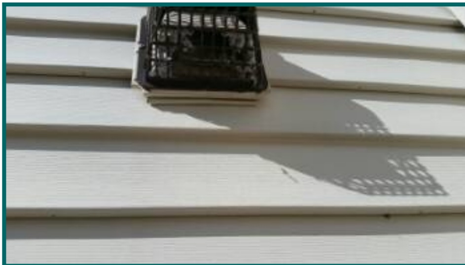
Dryer vent termination
