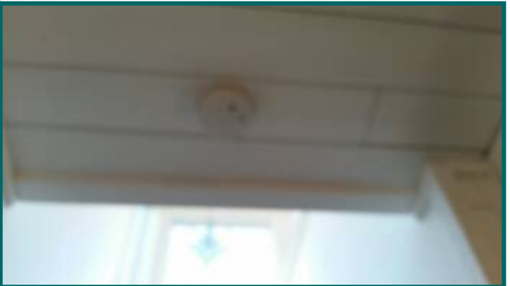
There is one smoke detector in bedroom hallway area, no smoke or CO detectors in bedrooms.
