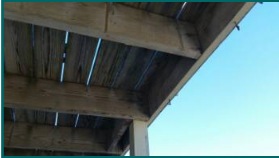
Missing Joist hangers.
