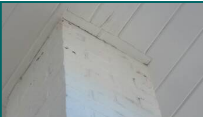
Ceiling stains at chimney roof penetration.
