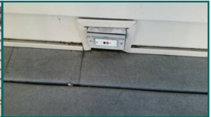
no power missing weatherproof cover at lower sliding door area
