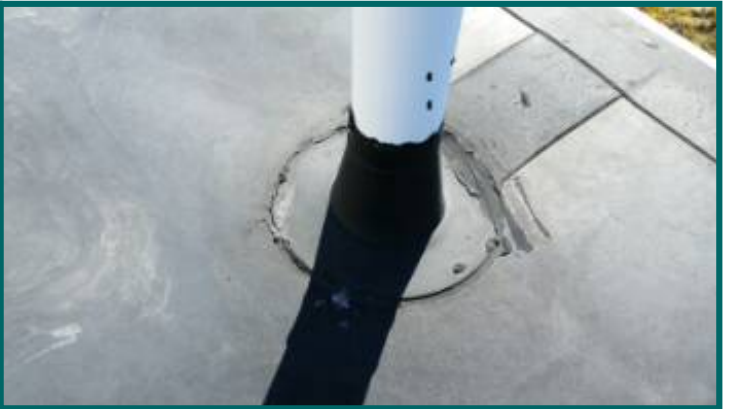
lower roof vent stack
